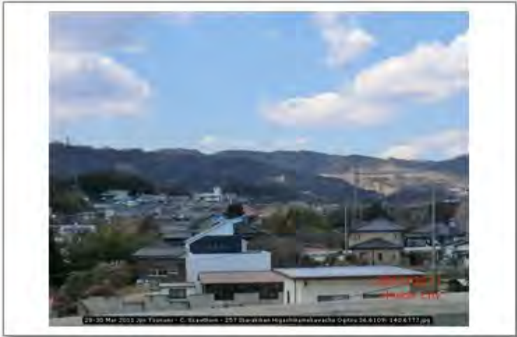
28-30 Mar 2011 Jpn Tsunami - C. Scawthorn - 257 Ibarakiken Higashinamekawacho Ogitsu 36.6109; 140.6777
