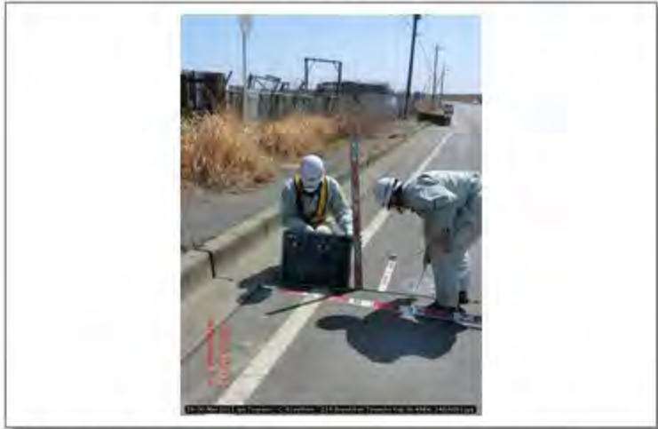
28-30 Mar 2011 Jpn Tsunami - C. Scawthorn - 219 Ibarakiken Tomecho Kuji 36.4864; 140.6081
