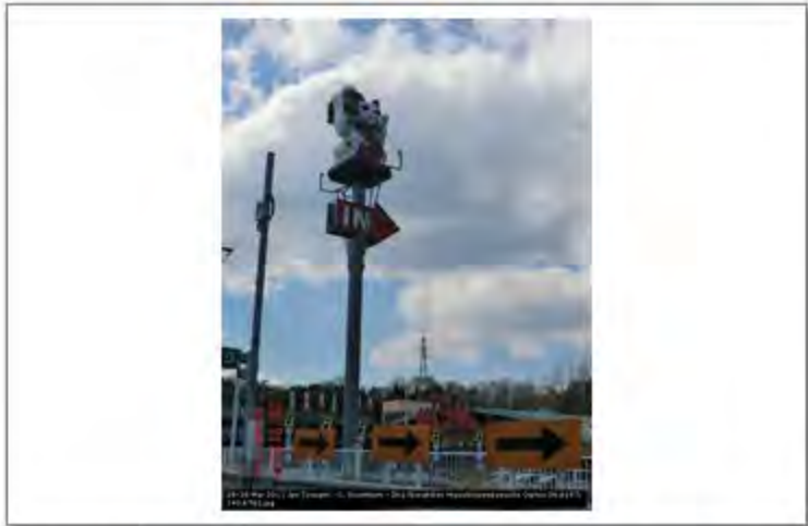
28-30 Mar 2011 Jpn Tsunami - C. Scawthorn - 261 Ibarakiken Higashinamekawacho Ogitsu 36.6187; 140.6768
