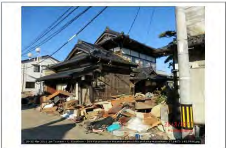
28-30 Mar 2011 Jpn Tsunami - C. Scawthorn - 389 Fukushimaken Hisanohamamachihisanohama H 11 1 1 27 4107 440 0000
