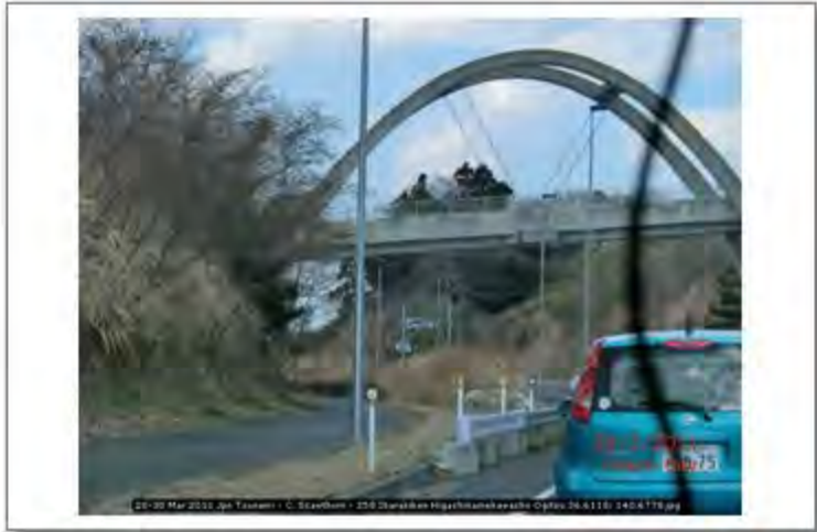
28-30 Mar 2011 Jpn Tsunami - C. Scawthorn - 258 Ibarakiken Higashinamekawacho Ogitsu 36.6118; 140.6776
