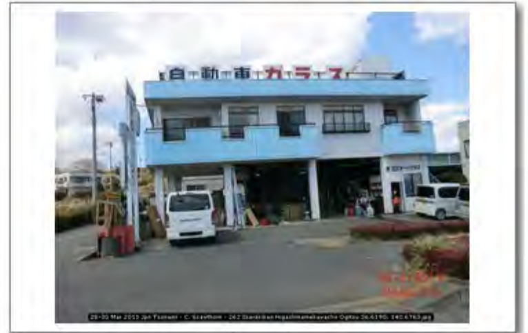
28-30 Mar 2011 Jpn Tsunami - C. Scawthorn - 262 Ibarakiken Higashinamekawacho Ogitsu 36.6190; 140.6768
