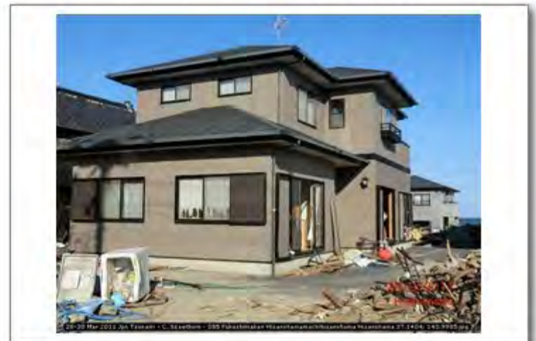
28-30 Mar 2011 Jpn Tsunami - C. Scawthorn - 385 Fukushimaken Hisanohamamachihisanohama H 11 1 1 27 4104 440 0005
