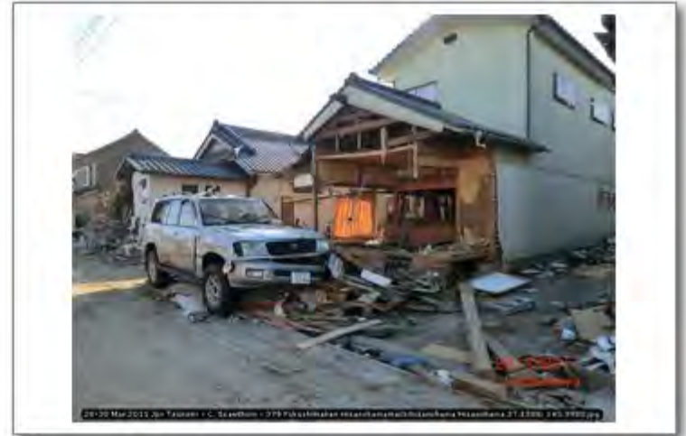
28-30 Mar 2011 Jpn Tsunami - C. Scawthorn - 379 Fukushimaken Hisanohamamachihisanohama H 11 1 1 27 4000 440 0000
