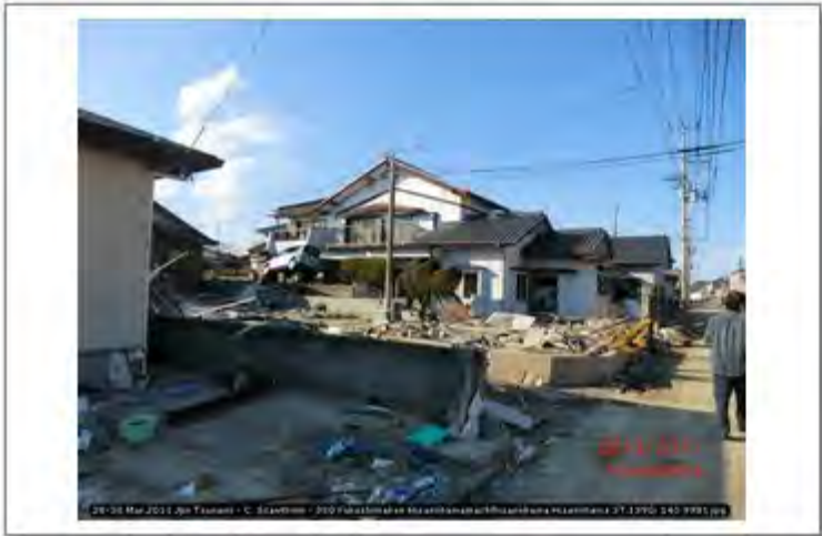
28-30 Mar 2011 Jpn Tsunami - C. Scawthorn - 380 Fukushimaken Hisanohamamachihisanohama H 11 1 1 27 4000 440 0004
