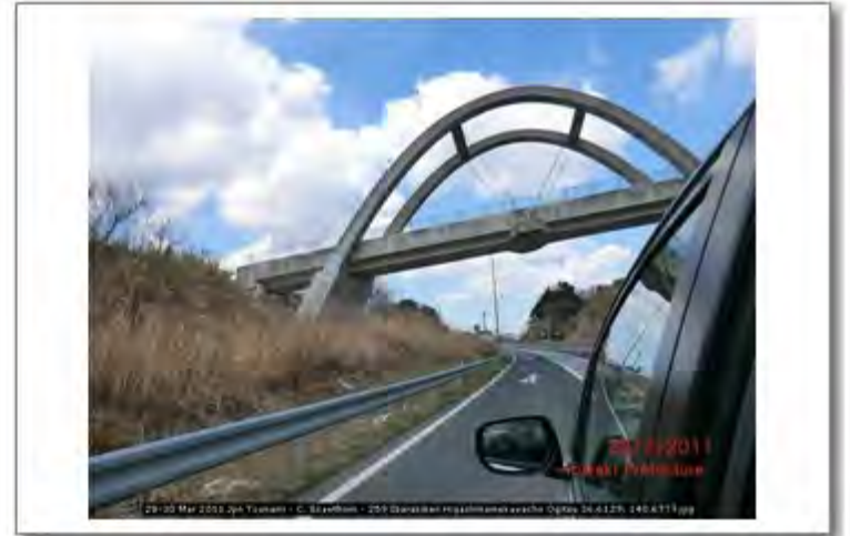
28-30 Mar 2011 Jpn Tsunami - C. Scawthorn - 259 Ibarakiken Higashinamekawacho Ogitsu 36.6129; 140.6777
