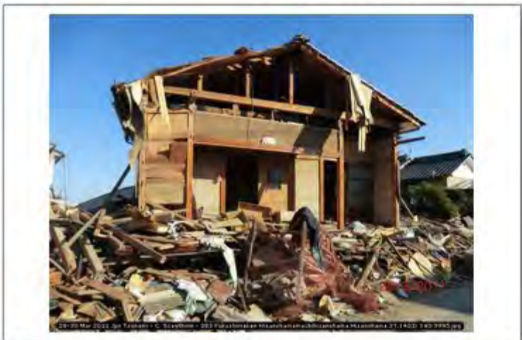
28-30 Mar 2011 Jpn Tsunami - C. Scawthorn - 383 Fukushimaken Hisanohamamachihisanohama H 11 1 1 27 4100 440 0005
