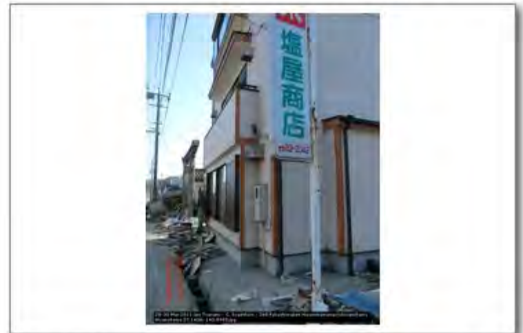
28-30 Mar 2011 Jpn Tsunami - C. Scawthorn - 388 Fukushimaken Hisanohamamachihisanohama H 11 1 1 27 4100 440 0005
