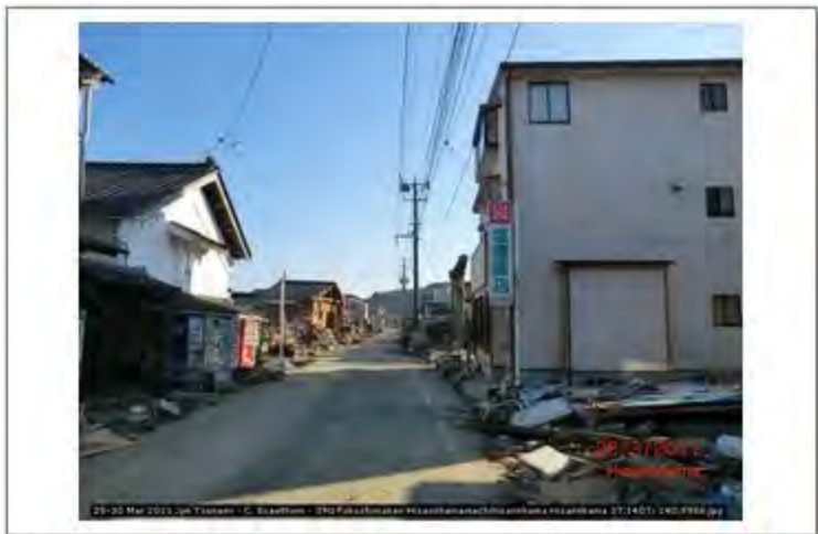
28-30 Mar 2011 Jpn Tsunami - C. Scawthorn - 390 Fukushimaken Hisanohamamachihisanohama H 11 1 1 27 4107 440 0000
