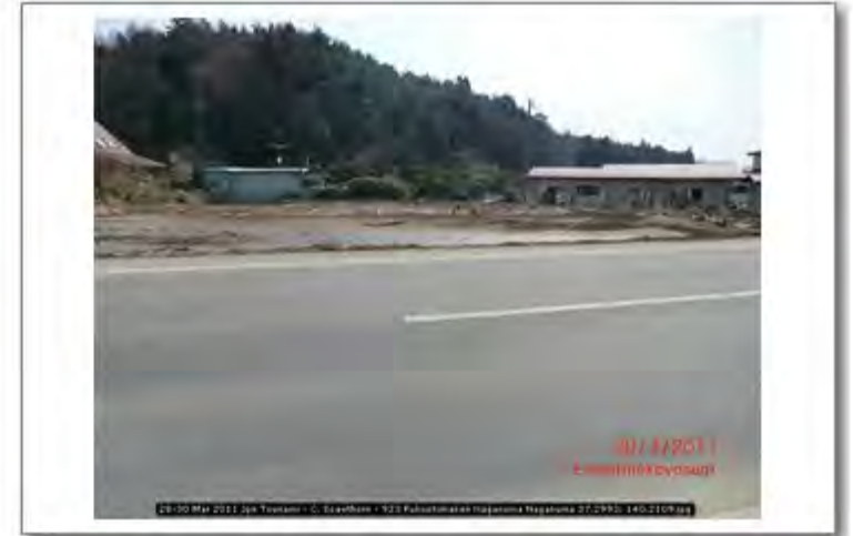
28-30 Mar 2011 Jpn Tsunami - C. Scawthorn - 923 Fukushimaken Naganuma Naganuma 37.2993; 140.2100
