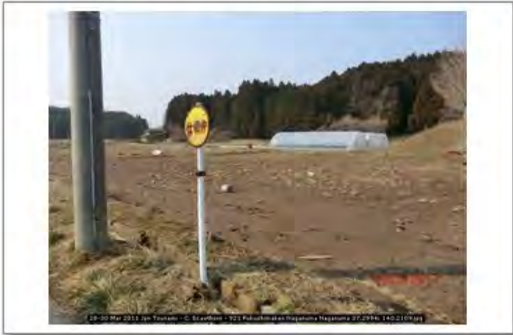
28-30 Mar 2011 Jpn Tsunami - C. Scawthorn - 921 Fukushimaken Naganuma Naganuma 37.2994; 140.2100
