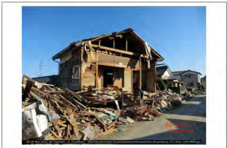
28-30 Mar 2011 Jpn Tsunami - C. Scawthorn - 384 Fukushimaken Hisanohamamachihisanohama H 11 1 1 27 4104 440 0005
