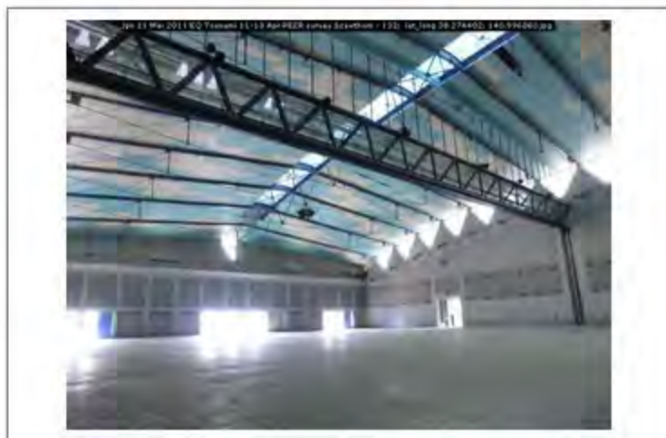
Jpn 11 Mar 2011 EQ Tsunami 11-13 Apr PEER survey Scawthorn - 132; lat_long 38.274402; 140.996060
