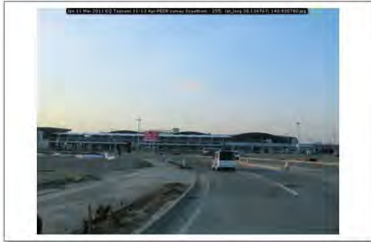
Jpn 11 Mar 2011 EQ Tsunami 11-13 Apr PEER survey Scawthorn - 255; lat_long 38.134767; 140.930780
