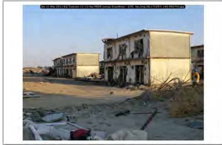
Jpn 11 Mar 2011 EQ Tsunami 11-13 Apr PEER survey Scawthorn - 225; lat_long 38.171057; 140.950792
