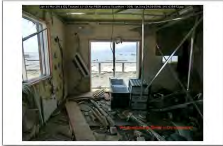
Jpn 11 Mar 2011 EQ Tsunami 11-13 Apr PEER survey Scawthorn - 309; lat_long 39.010598; 141.635872
