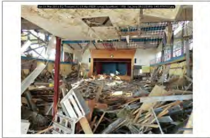
Jpn 11 Mar 2011 EQ Tsunami 11-13 Apr PEER survey Scawthorn - 153; lat_long 38.222383; 140.979703
