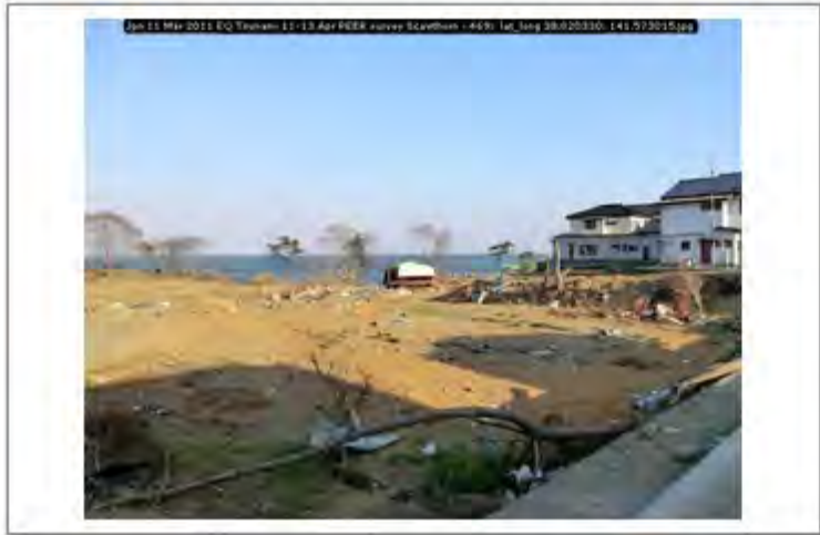
Jpn 11 Mar 2011 EQ Tsunami 11-13 Apr PEER survey Scawthorn - 469; lat_long 38.820330; 141.573015
