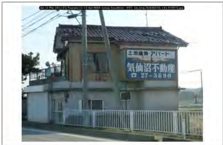
Jpn 11 Mar 2011 EQ Tsunami 11-13 Apr PEER survey Scawthorn - 457; lat_long 38.836070; 141.578572
