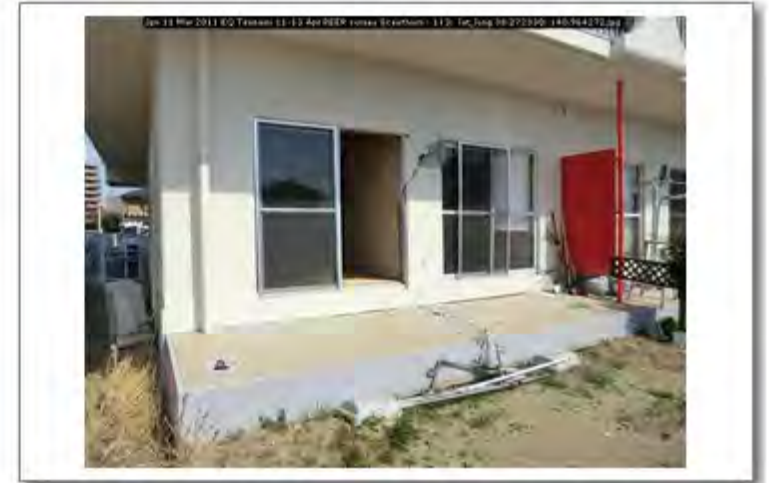
Jpn 11 Mar 2011 EQ Tsunami 11-13 Apr PEER survey Scawthorn - 113; lat_long 38.272330; 140.964272
