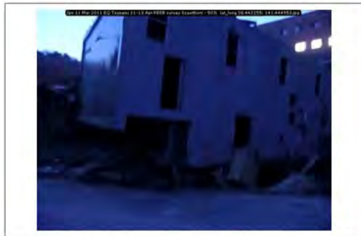
Jpn 11 Mar 2011 EQ Tsunami 11-13 Apr PEER survey Scawthorn - 503; lat_long 38.442255; 141.444953
