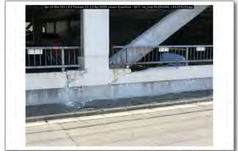
Jpn 11 Mar 2011 EQ Tsunami 11-13 Apr PEER survey Scawthorn - 067; lat_long 38.254248; 140.925103
