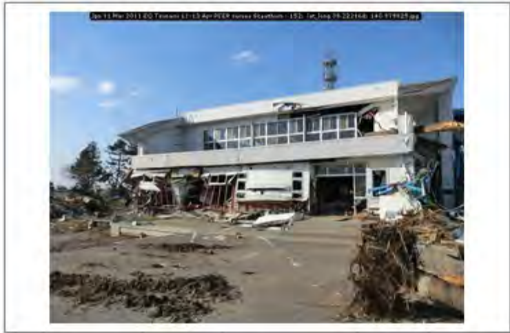
Jpn 11 Mar 2011 EQ Tsunami 11-13 Apr PEER survey Scawthorn - 152; lat_long 38.222168; 140.979825
