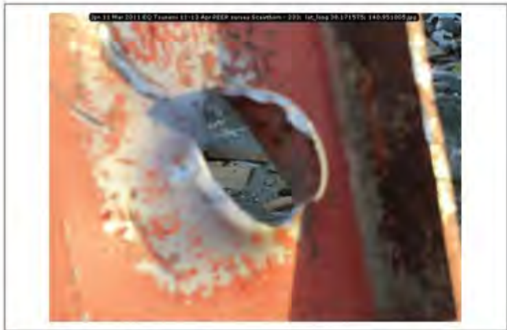
Jpn 11 Mar 2011 EQ Tsunami 11-13 Apr PEER survey Scawthorn - 233; lat_long 38.171575; 140.951005
