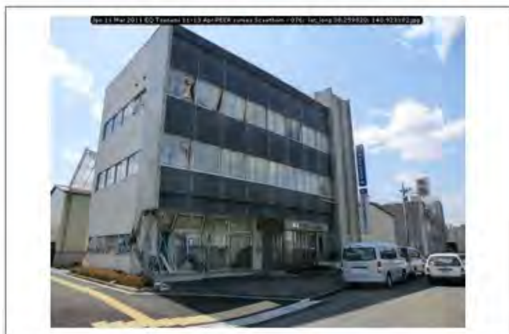
Jpn 11 Mar 2011 EQ Tsunami 11-13 Apr PEER survey Scawthorn - 076; lat_long 38.259820; 140.923182
