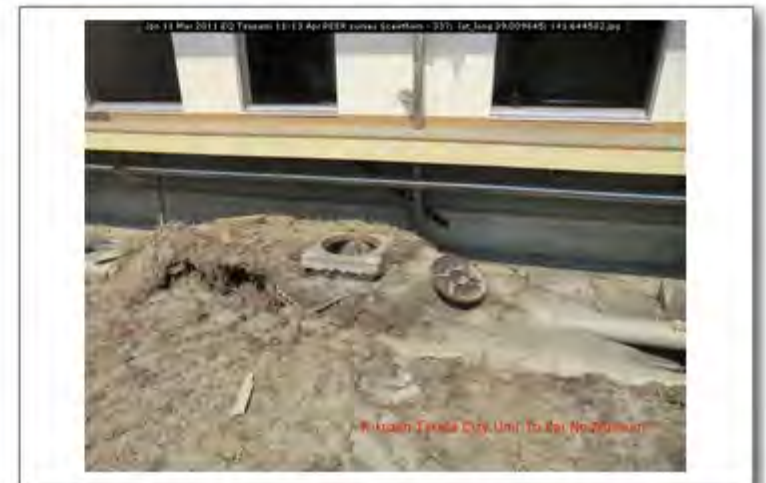
Jpn 11 Mar 2011 EQ Tsunami 11-13 Apr PEER survey Scawthorn - 337; lat_long 39.009645; 141.644582
