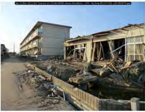
Jpn 11 Mar 2011 EQ Tsunami 11-13 Apr PEER survey Scawthorn - 197; lat_long 38.171722; 140.952870
