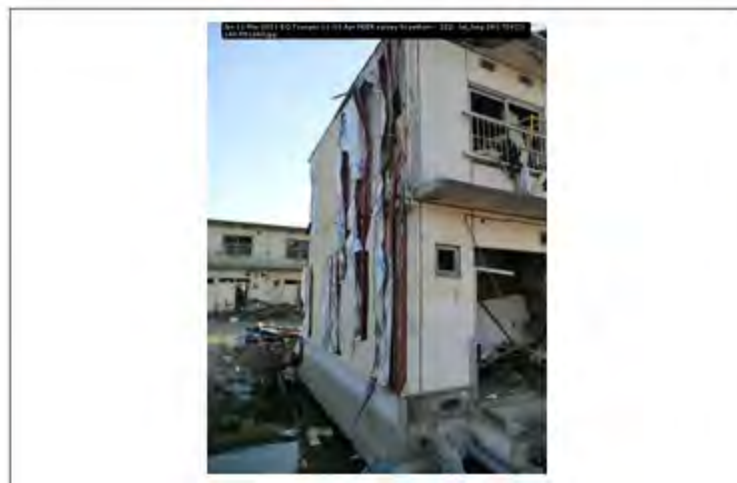
Jpn 11 Mar 2011 EQ Tsunami 11-13 Apr PEER survey Scawthorn - 222; lat_long 38.170923; 140.951040
