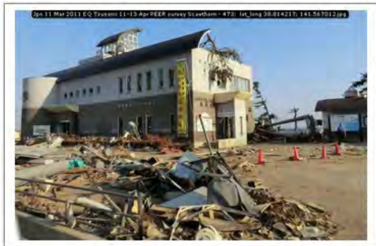
Jpn 11 Mar 2011 EQ Tsunami 11-13 Apr PEER survey Scawthorn - 473; lat_long 38.814217; 141.567012
