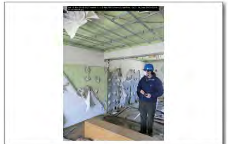
Jpn 11 Mar 2011 EQ Tsunami 11-13 Apr PEER survey Scawthorn - 307; lat_long 39.010285; 141.635865
