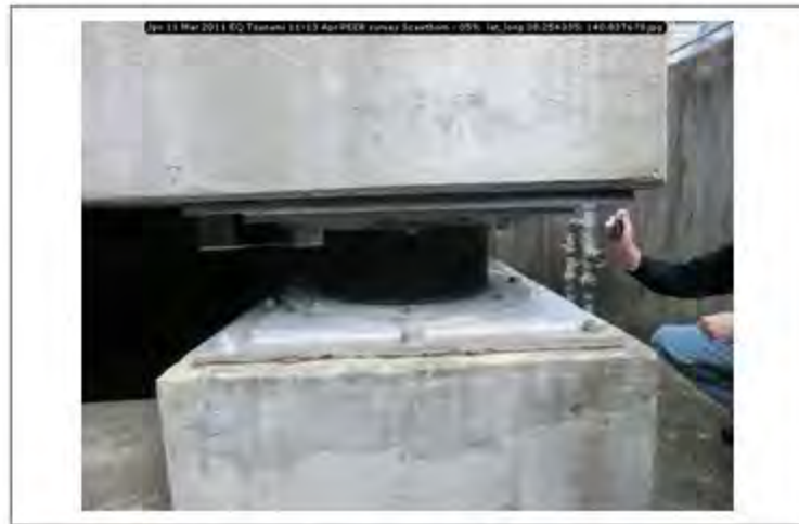
Jpn 11 Mar 2011 EQ Tsunami 11-13 Apr PEER survey Scawthorn - 059; lat_long 38.254335; 140.837678
