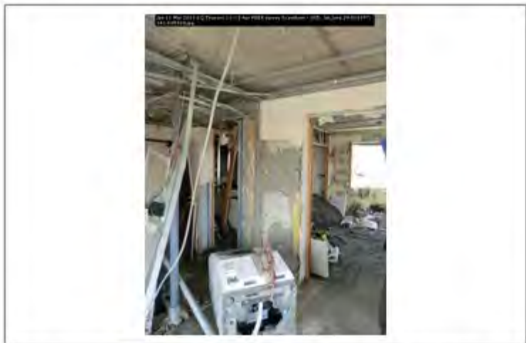
Jpn 11 Mar 2011 EQ Tsunami 11-13 Apr PEER survey Scawthorn - 305; lat_long 39.010397; 141.635910
