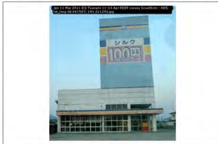
Jpn 11 Mar 2011 EQ Tsunami 11-13 Apr PEER survey Scawthorn - 485; lat_long 38.441507; 141.311292
