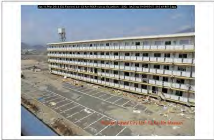
Jpn 11 Mar 2011 EQ Tsunami 11-13 Apr PEER survey Scawthorn - 332; lat_long 39.009767; 141.644612
