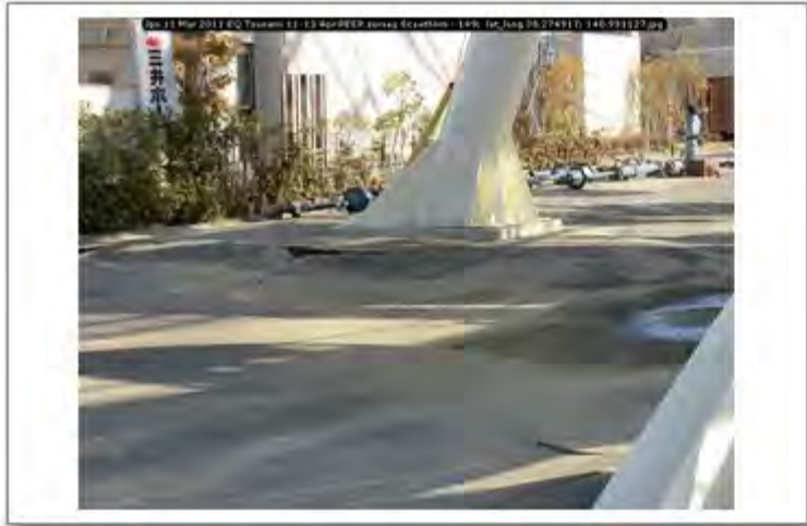
Jpn 11 Mar 2011 EQ Tsunami 11-13 Apr PEER survey Scawthorn - 149; lat_long 38.274917; 140.991127
