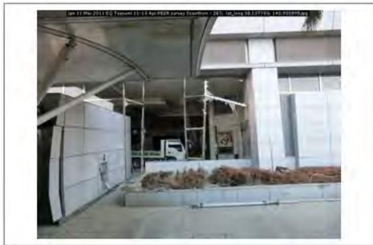
Jpn 11 Mar 2011 EQ Tsunami 11-13 Apr PEER survey Scawthorn - 267; lat_long 38.137783; 140.930995
