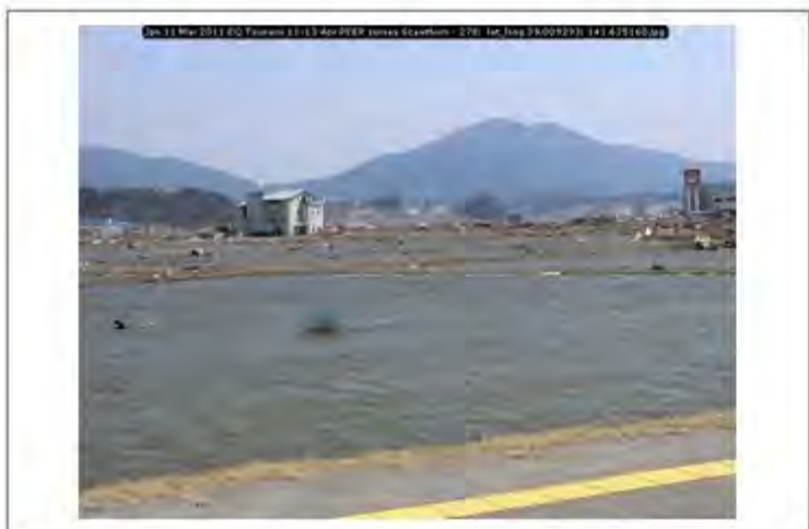
Jpn 11 Mar 2011 EQ Tsunami 11-13 Apr PEER survey Scawthorn - 278; lat_long 39.009293; 141.625160
