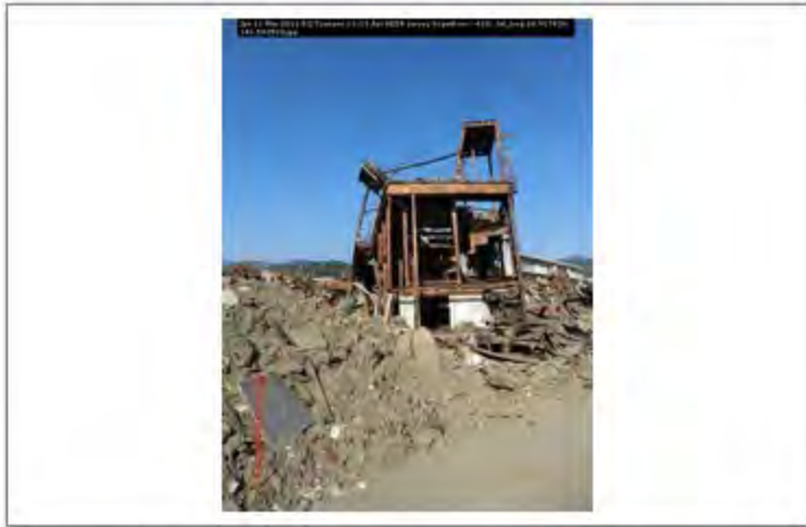
Jpn 11 Mar 2011 EQ Tsunami 11-13 Apr PEER survey Scawthorn - 410; lat_long 38.917838; 141.582528
