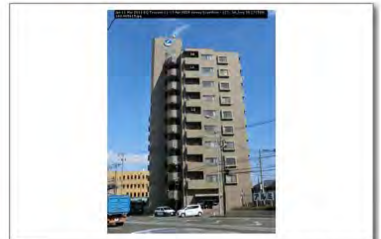
Jpn 11 Mar 2011 EQ Tsunami 11-13 Apr PEER survey Scawthorn - 127; lat_long 38.271588; 140.965615
