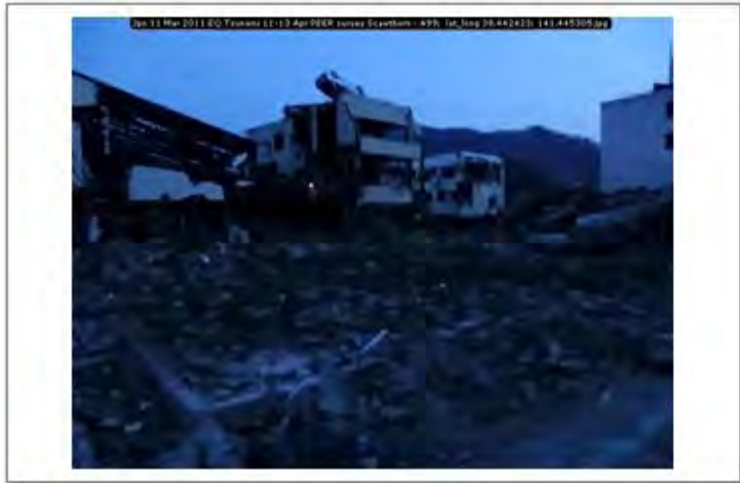
Jpn 11 Mar 2011 EQ Tsunami 11-13 Apr PEER survey Scawthorn - 499; lat_long 38.442423; 141.445305
