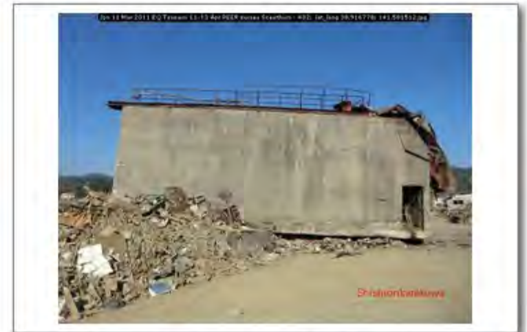
Jpn 11 Mar 2011 EQ Tsunami 11-13 Apr PEER survey Scawthorn - 432; lat_long 38.916778; 141.581512
