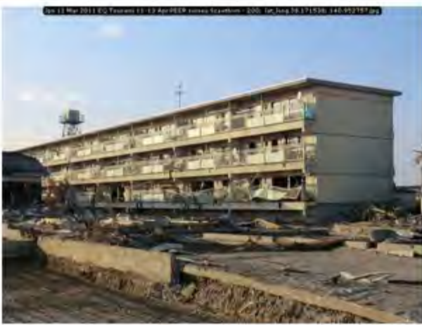
Jpn 11 Mar 2011 EQ Tsunami 11-13 Apr PEER survey Scawthorn - 200; lat_long 38.171538; 140.952757
