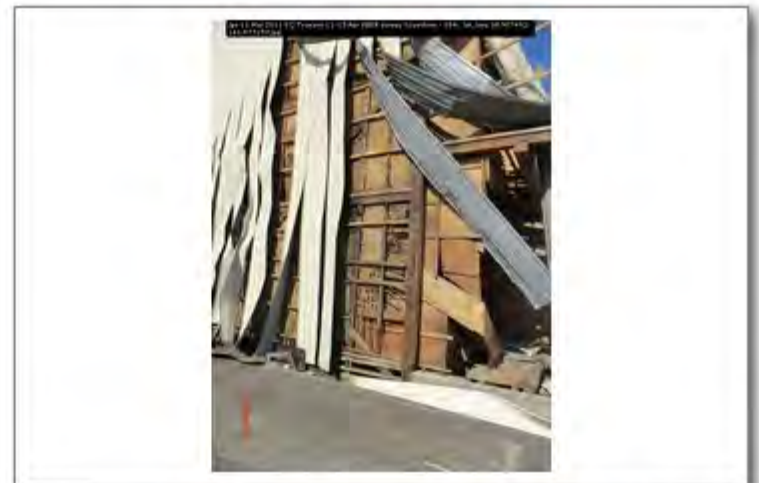
Jpn 11 Mar 2011 EQ Tsunami 11-13 Apr PEER survey Scawthorn - 384; lat_long 38.907492; 141.577257
