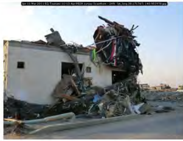
Jpn 11 Mar 2011 EQ Tsunami 11-13 Apr PEER survey Scawthorn - 249; lat_long 38.171767; 140.952978
