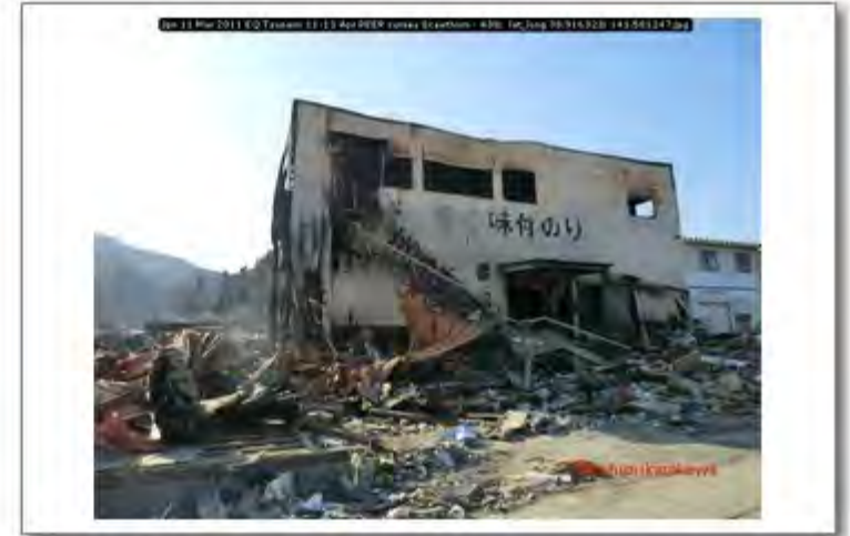
Jpn 11 Mar 2011 EQ Tsunami 11-13 Apr PEER survey Scawthorn - 438; lat_long 38.916323; 141.581247
