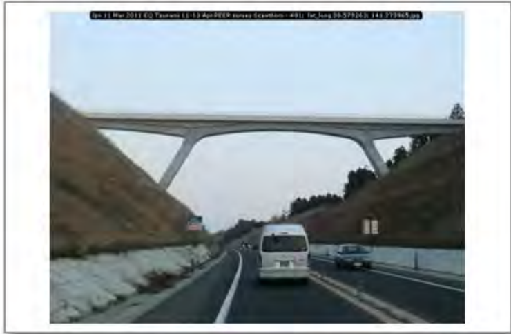
Jpn 11 Mar 2011 EQ Tsunami 11-13 Apr PEER survey Scawthorn - 481; lat_long 38.579263; 141.273965
