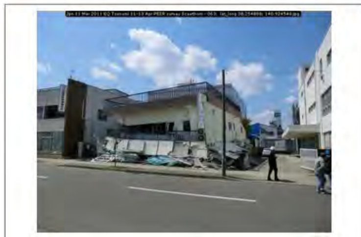
Jpn 11 Mar 2011 EQ Tsunami 11-13 Apr PEER survey Scawthorn - 063; lat_long 38.254888; 140.924548
