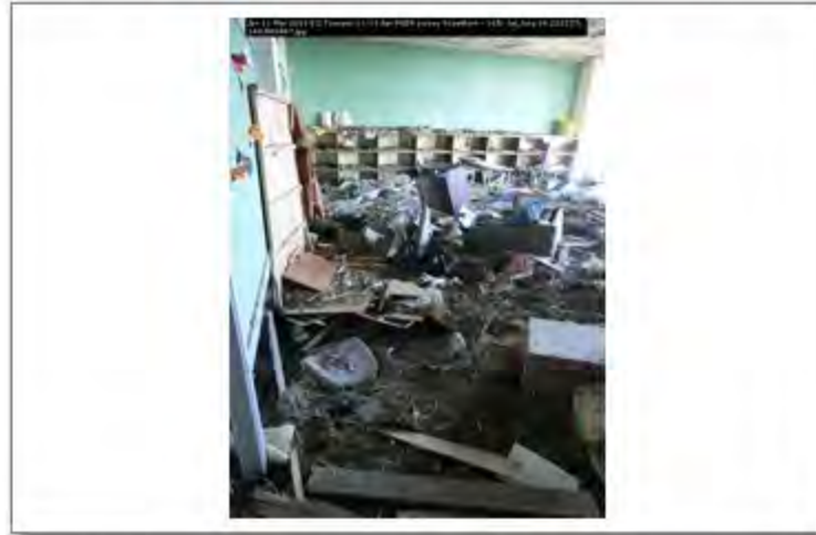
Jpn 11 Mar 2011 EQ Tsunami 11-13 Apr PEER survey Scawthorn - 165; lat_long 38.222237; 140.980487
