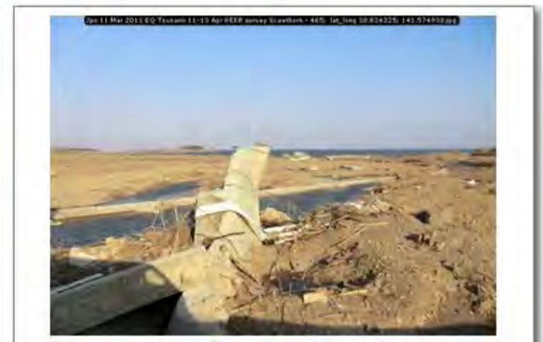
Jpn 11 Mar 2011 EQ Tsunami 11-13 Apr PEER survey Scawthorn - 465; lat_long 38.824225; 141.574938
