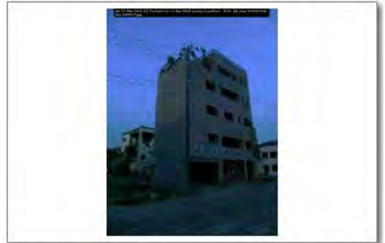
Jpn 11 Mar 2011 EQ Tsunami 11-13 Apr PEER survey Scawthorn - 514; lat_long 38.442468; 141.445547
