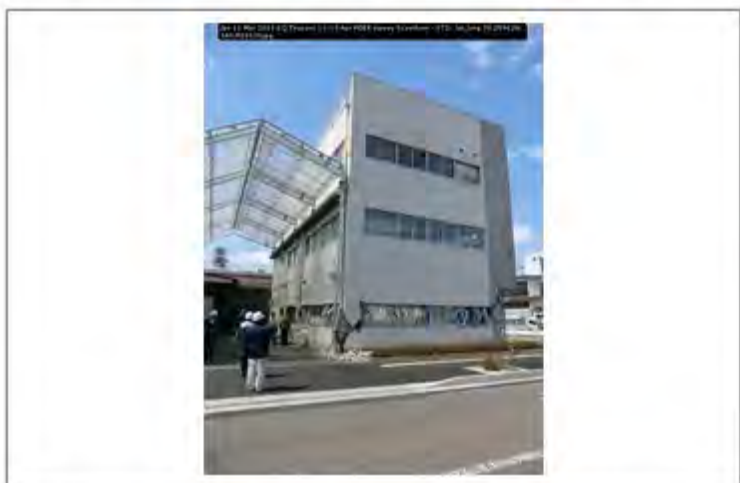
Jpn 11 Mar 2011 EQ Tsunami 11-13 Apr PEER survey Scawthorn - 072; lat_long 38.259628; 140.923320
