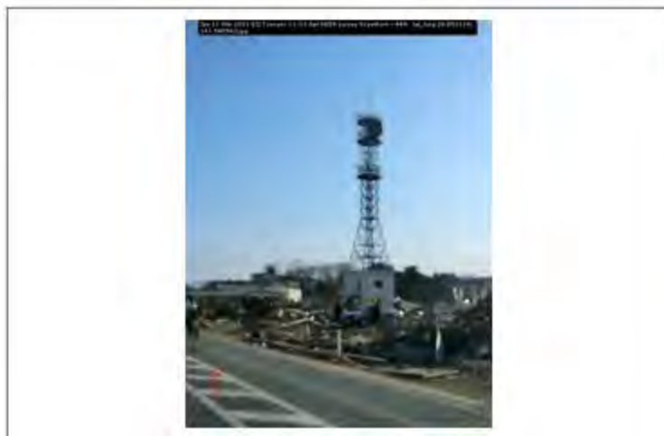
Jpn 11 Mar 2011 EQ Tsunami 11-13 Apr PEER survey Scawthorn - 449; lat_long 38.853118; 141.580542
