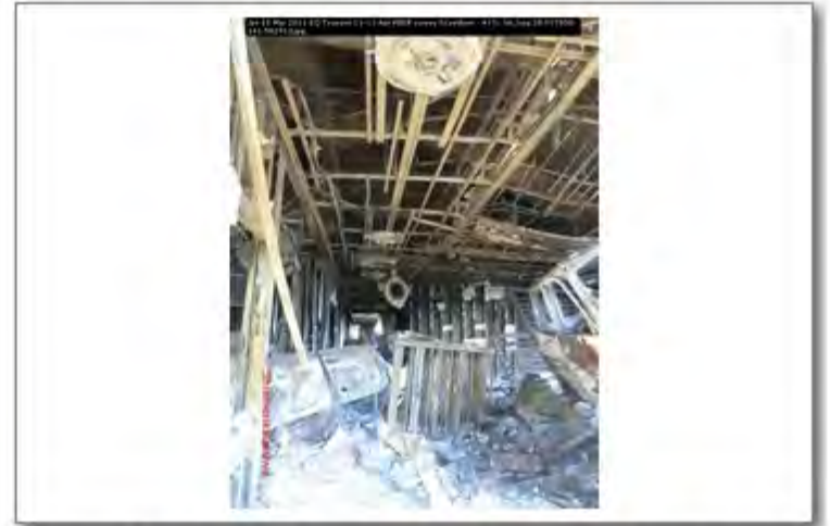
Jpn 11 Mar 2011 EQ Tsunami 11-13 Apr PEER survey Scawthorn - 417; lat_long 38.917500; 141.582913
