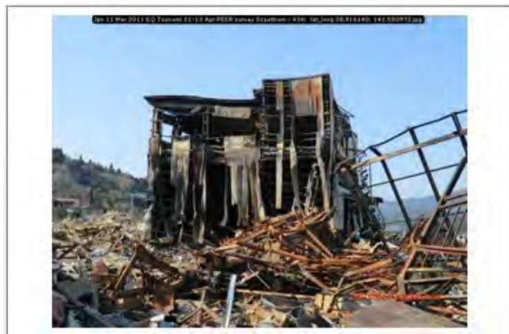
Jpn 11 Mar 2011 EQ Tsunami 11-13 Apr PEER survey Scawthorn - 434; lat_long 38.916140; 141.580972
