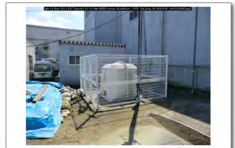
Jpn 11 Mar 2011 EQ Tsunami 11-13 Apr PEER survey Scawthorn - 095; lat_long 38.266318; 140.928480
