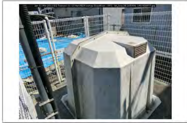
Jpn 11 Mar 2011 EQ Tsunami 11-13 Apr PEER survey Scawthorn - 097; lat_long 38.265908; 140.928877
