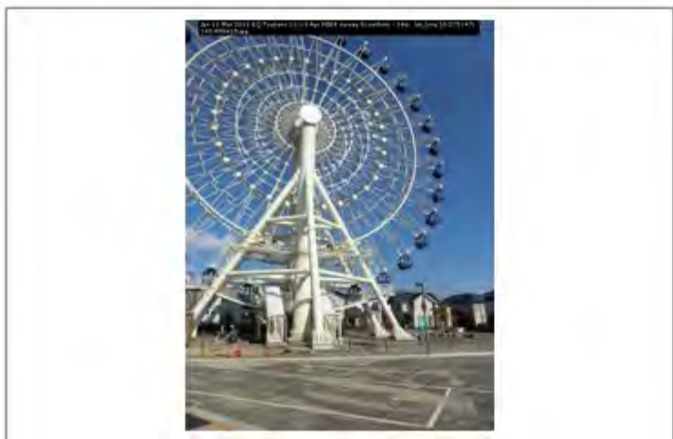
Jpn 11 Mar 2011 EQ Tsunami 11-13 Apr PEER survey Scawthorn - 146; lat_long 38.275147; 140.990425
