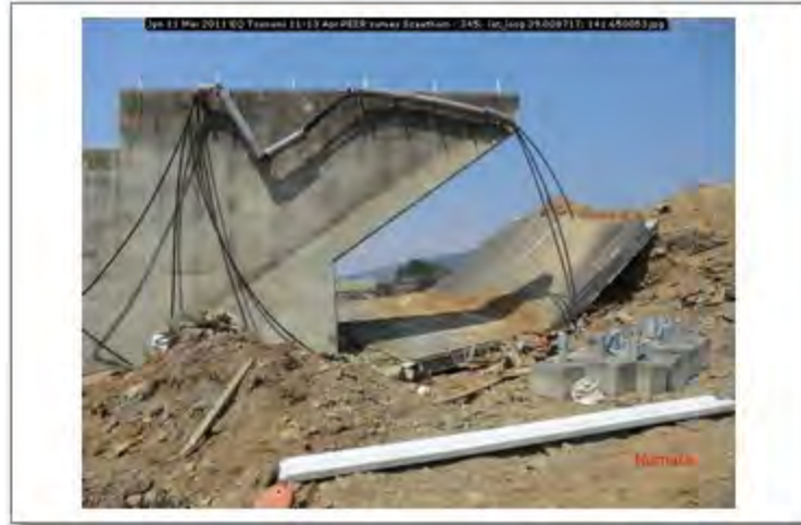
Jpn 11 Mar 2011 EQ Tsunami 11-13 Apr PEER survey Scawthorn - 345; lat_long 39.008717; 141.650053
