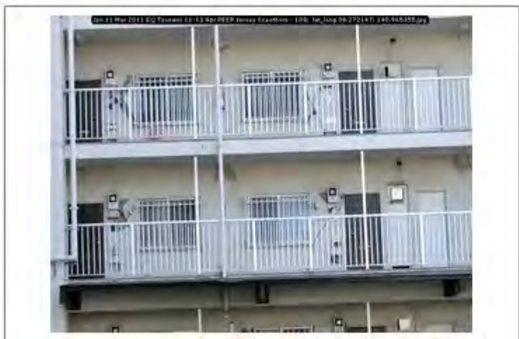
Jpn 11 Mar 2011 EQ Tsunami 11-13 Apr PEER survey Scawthorn - 108; lat_long 38.272147; 140.965355
