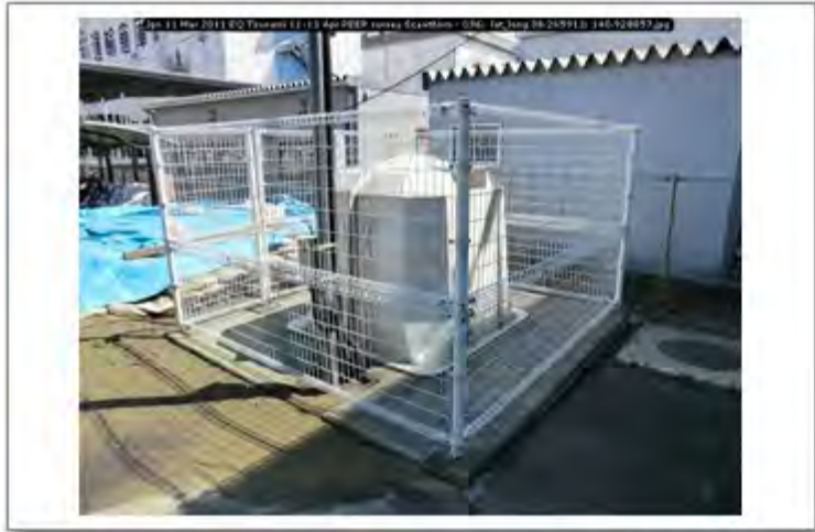
Jpn 11 Mar 2011 EQ Tsunami 11-13 Apr PEER survey Scawthorn - 096; lat_long 38.265913; 140.928857
