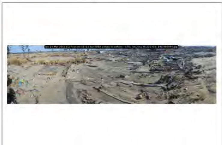
Jpn 11 Mar 2011 EQ Tsunami 11-13 Apr PEER survey Scawthorn - 176; lat_long 38.222333; 140.980597
