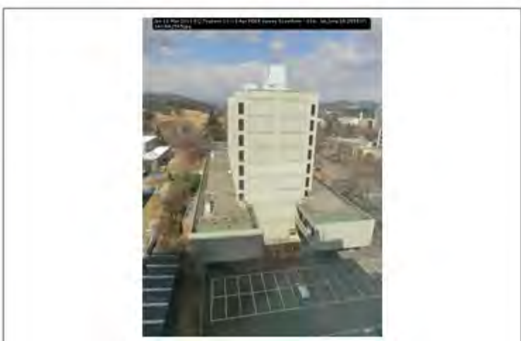
Jpn 11 Mar 2011 EQ Tsunami 11-13 Apr PEER survey Scawthorn - 016; lat_long 38.255537; 140.842565
