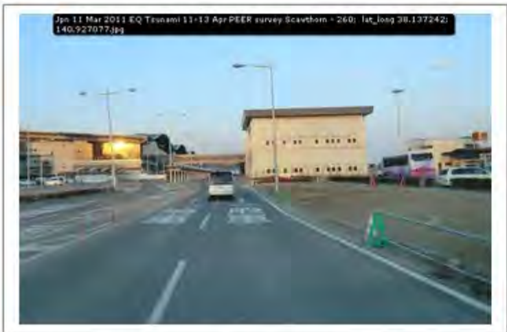
Jpn 11 Mar 2011 EQ Tsunami 11-13 Apr PEER survey Scawthorn - 260; lat_long 38.137242; 140.927077
