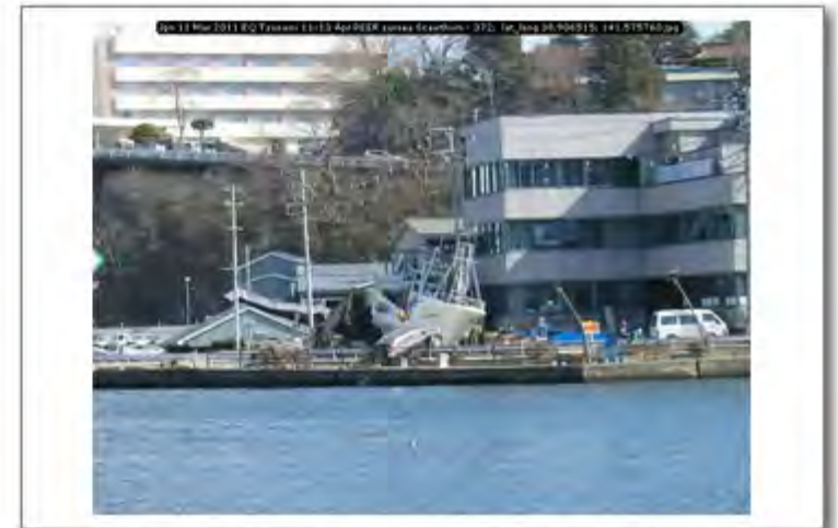
Jpn 11 Mar 2011 EQ Tsunami 11-13 Apr PEER survey Scawthorn - 372; lat_long 38.906515; 141.575760
