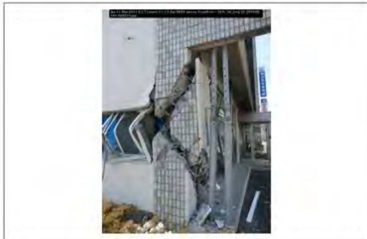
Jpn 11 Mar 2011 EQ Tsunami 11-13 Apr PEER survey Scawthorn - 069; lat_long 38.259845; 140.923210
