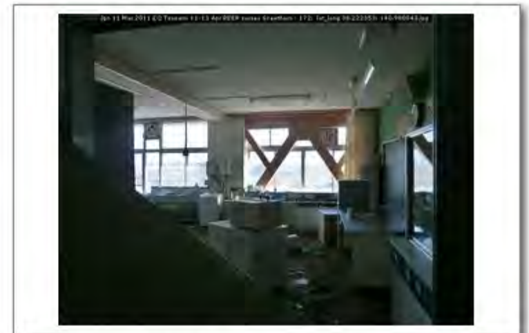
Jpn 11 Mar 2011 EQ Tsunami 11-13 Apr PEER survey Scawthorn - 172; lat_long 38.222353; 140.980843
