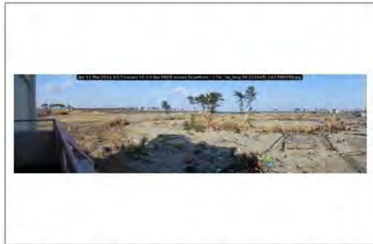
Jpn 11 Mar 2011 EQ Tsunami 11-13 Apr PEER survey Scawthorn - 174; lat_long 38.222465; 140.980358
