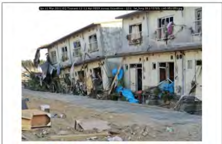
Jpn 11 Mar 2011 EQ Tsunami 11-13 Apr PEER survey Scawthorn - 221; lat_long 38.170785; 140.951053
