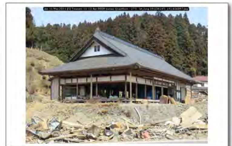
Jpn 11 Mar 2011 EQ Tsunami 11-13 Apr PEER survey Scawthorn - 277; lat_long 39.034147; 141.606897
