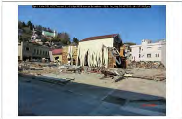
Jpn 11 Mar 2011 EQ Tsunami 11-13 Apr PEER survey Scawthorn - 383; lat_long 38.907330; 141.577102
