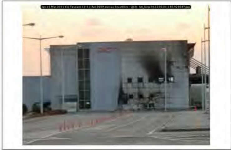
Jpn 11 Mar 2011 EQ Tsunami 11-13 Apr PEER survey Scawthorn - 269; lat_long 38.137640; 140.928697
