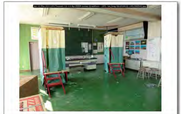
Jpn 11 Mar 2011 EQ Tsunami 11-13 Apr PEER survey Scawthorn - 187; lat_long 38.222432; 140.980542
