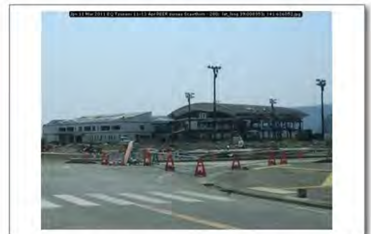
Jpn 11 Mar 2011 EQ Tsunami 11-13 Apr PEER survey Scawthorn - 280; lat_long 39.008353; 141.626052
