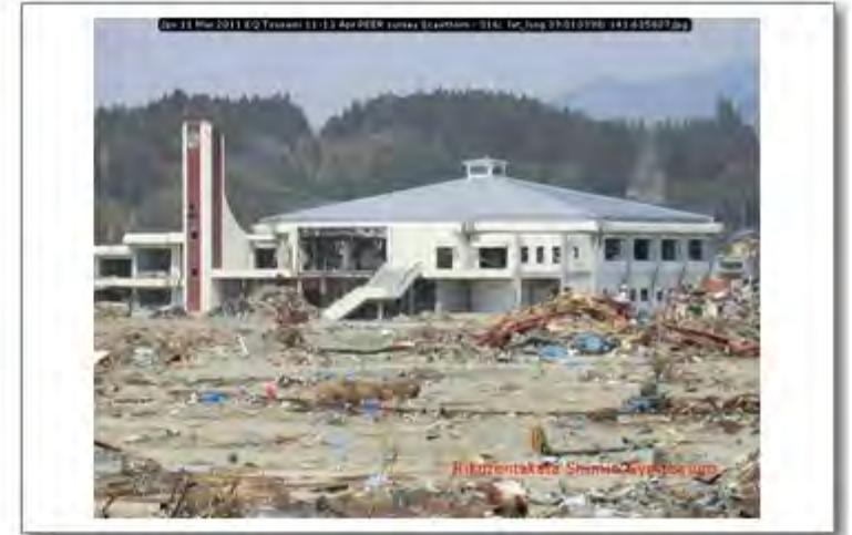
Jpn 11 Mar 2011 EQ Tsunami 11-13 Apr PEER survey Scawthorn - 316; lat_long 39.010398; 141.635807
