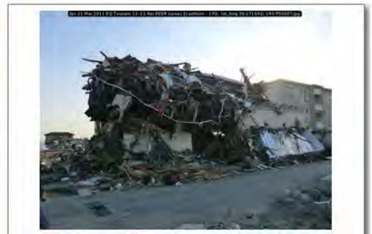
Jpn 11 Mar 2011 EQ Tsunami 11-13 Apr PEER survey Scawthorn - 193; lat_long 38.171842; 140.953007
