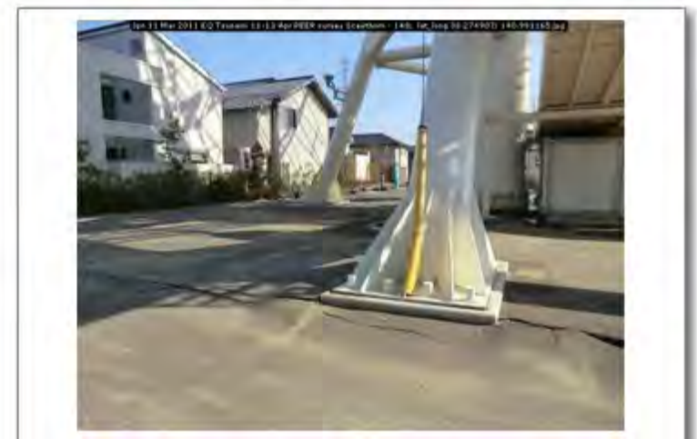
Jpn 11 Mar 2011 EQ Tsunami 11-13 Apr PEER survey Scawthorn - 148; lat_long 38.274907; 140.991165
