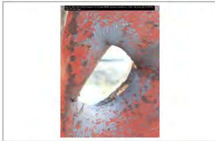
Jpn 11 Mar 2011 EQ Tsunami 11-13 Apr PEER survey Scawthorn - 234; lat_long 38.171575; 140.951017
