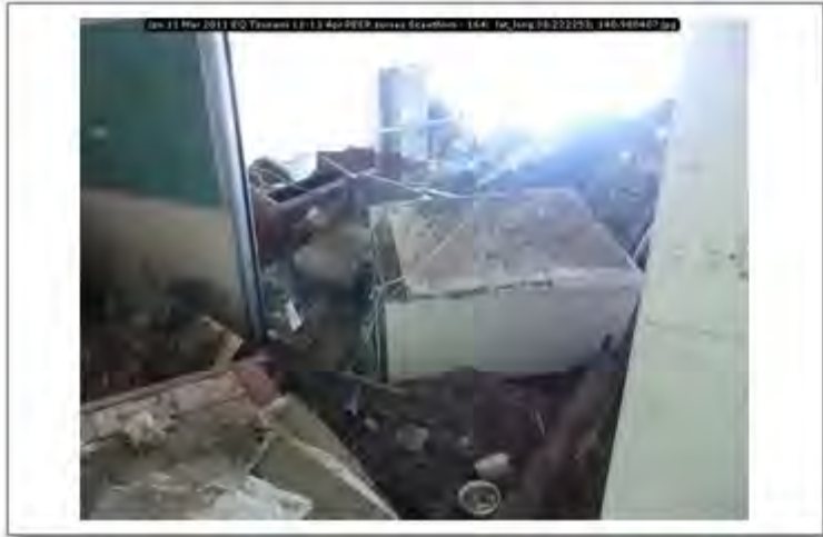
Jpn 11 Mar 2011 EQ Tsunami 11-13 Apr PEER survey Scawthorn - 164; lat_long 38.222253; 140.980407
