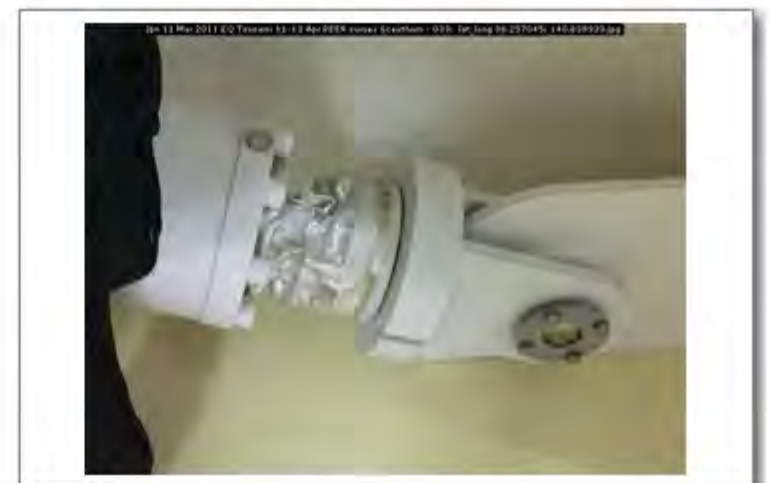
Jpn 11 Mar 2011 EQ Tsunami 11-13 Apr PEER survey Scawthorn - 033; lat_long 38.257045; 140.838933
