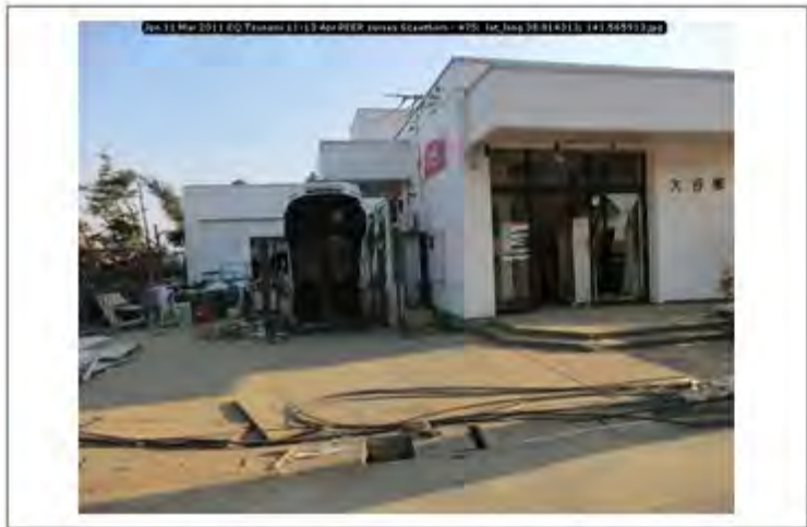
Jpn 11 Mar 2011 EQ Tsunami 11-13 Apr PEER survey Scawthorn - 475; lat_long 38.814313; 141.565913
