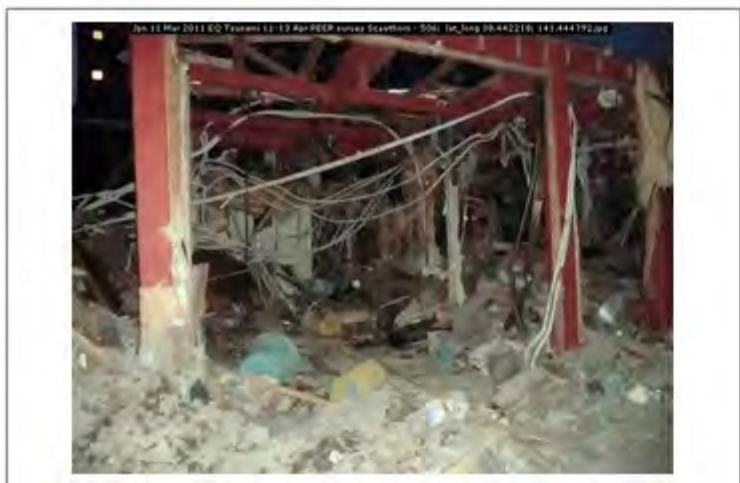
Jpn 11 Mar 2011 EQ Tsunami 11-13 Apr PEER survey Scawthorn - 506; lat_long 38.442218; 141.444792
