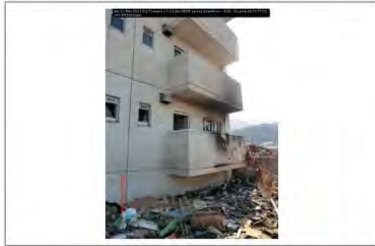
Jpn 11 Mar 2011 EQ Tsunami 11-13 Apr PEER survey Scawthorn - 425; lat_long 38.917973; 141.583322
