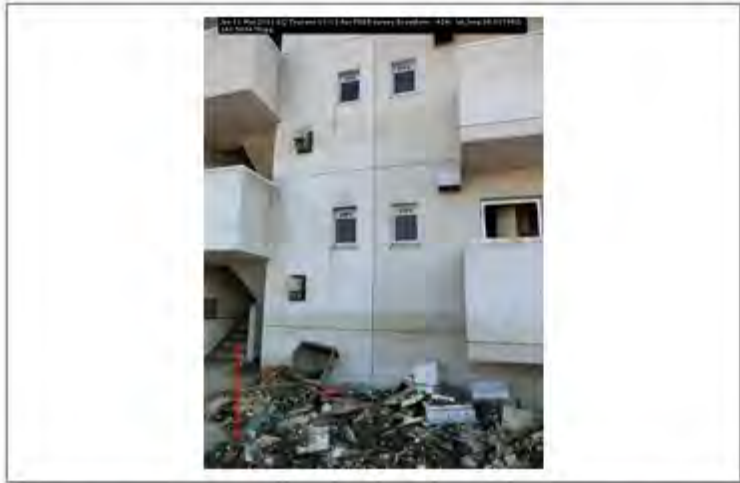
Jpn 11 Mar 2011 EQ Tsunami 11-13 Apr PEER survey Scawthorn - 424; lat_long 38.917952; 141.583478
