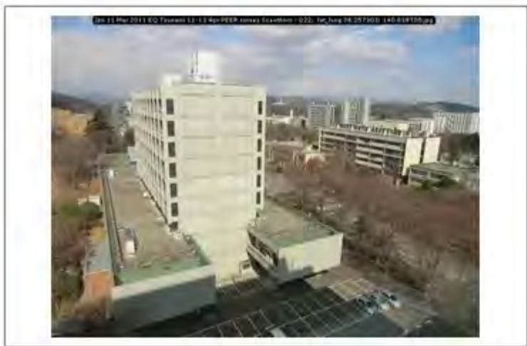
Jpn 11 Mar 2011 EQ Tsunami 11-13 Apr PEER survey Scawthorn - 022; lat_long 38.257303; 140.838705
