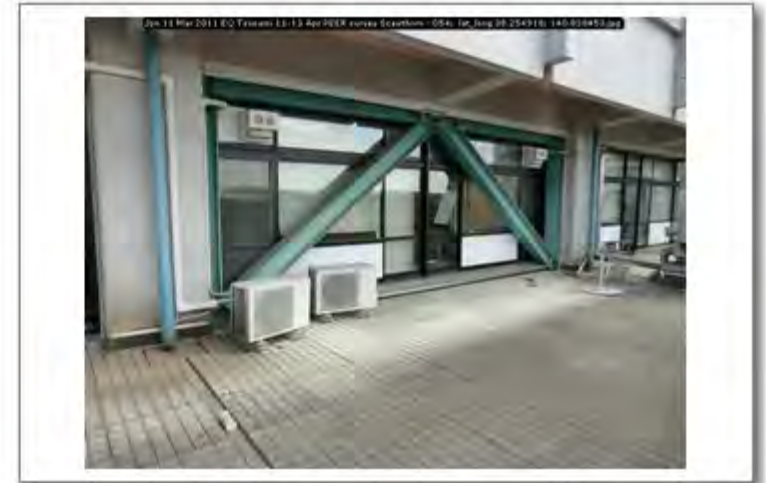
Jpn 11 Mar 2011 EQ Tsunami 11-13 Apr PEER survey Scawthorn - 054; lat_long 38.254918; 140.838453
