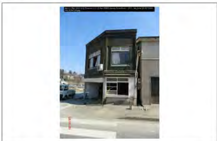
Jpn 11 Mar 2011 EQ Tsunami 11-13 Apr PEER survey Scawthorn - 397; lat_long 38.907668; 141.576733
