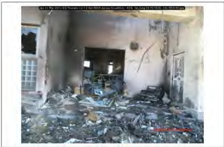
Jpn 11 Mar 2011 EQ Tsunami 11-13 Apr PEER survey Scawthorn - 418; lat_long 38.917635; 141.583140
