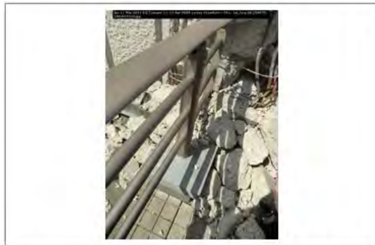
Jpn 11 Mar 2011 EQ Tsunami 11-13 Apr PEER survey Scawthorn - 041; lat_long 38.254875; 140.839333
