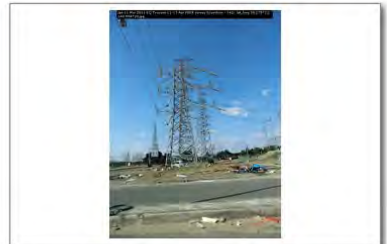
Jpn 11 Mar 2011 EQ Tsunami 11-13 Apr PEER survey Scawthorn - 142; lat_long 38.275772; 140.994720
