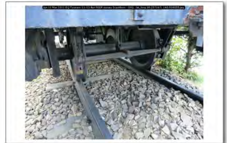
Jpn 11 Mar 2011 EQ Tsunami 11-13 Apr PEER survey Scawthorn - 092; lat_long 38.257167; 140.938055
