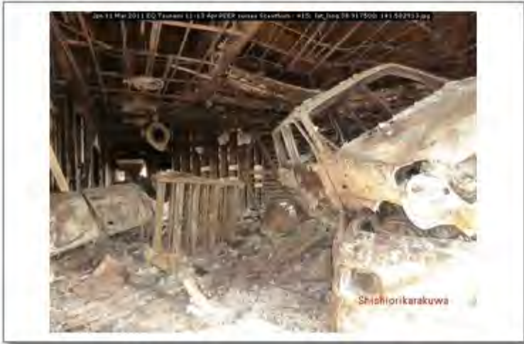
Jpn 11 Mar 2011 EQ Tsunami 11-13 Apr PEER survey Scawthorn - 415; lat_long 38.917500; 141.582913
