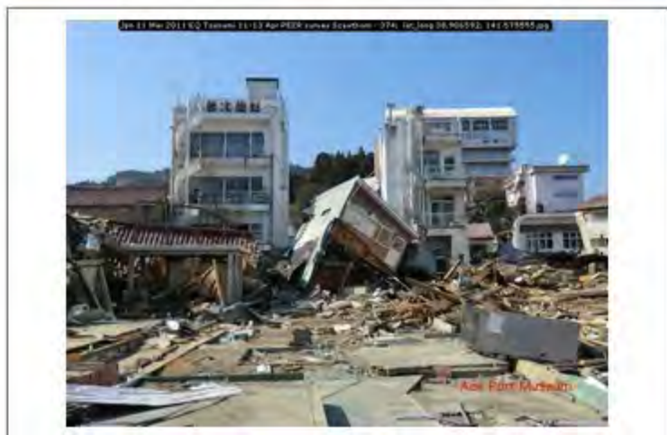
Jpn 11 Mar 2011 EQ Tsunami 11-13 Apr PEER survey Scawthorn - 374; lat_long 38.906592; 141.575555
