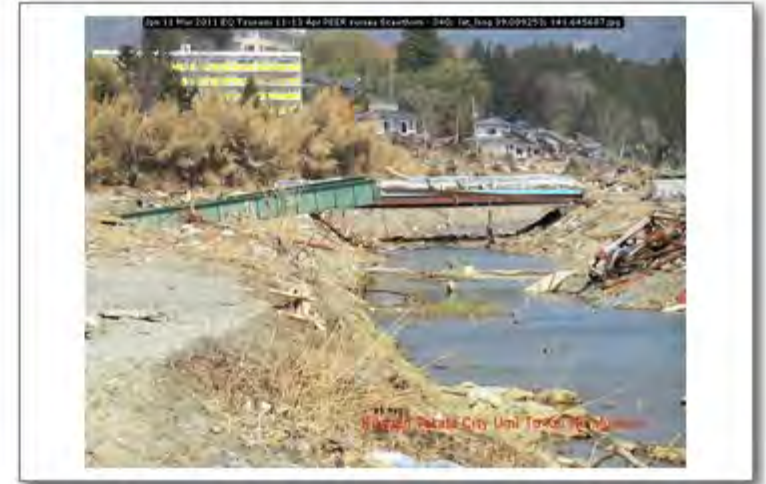
Jpn 11 Mar 2011 EQ Tsunami 11-13 Apr PEER survey Scawthorn - 340; lat_long 39.009253; 141.645687
