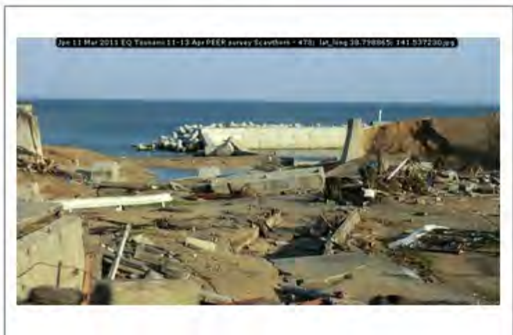
Jpn 11 Mar 2011 EQ Tsunami 11-13 Apr PEER survey Scawthorn - 478; lat_long 38.798865; 141.537230
