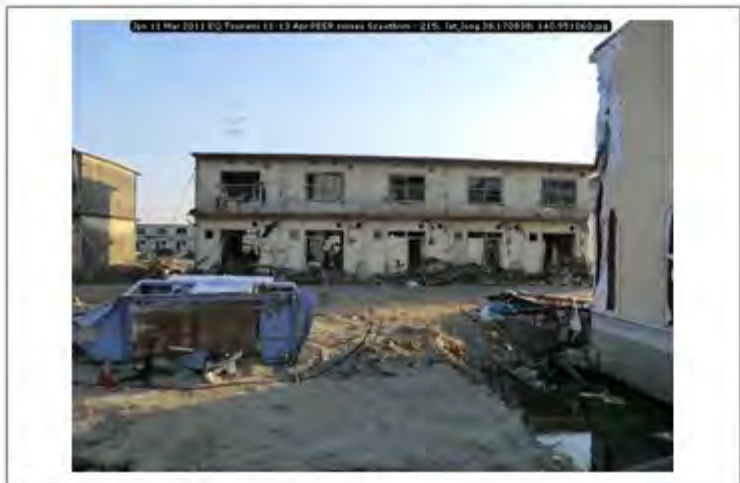
Jpn 11 Mar 2011 EQ Tsunami 11-13 Apr PEER survey Scawthorn - 215; lat_long 38.170838; 140.951060
