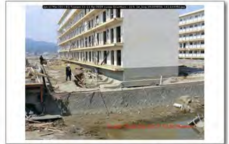
Jpn 11 Mar 2011 EQ Tsunami 11-13 Apr PEER survey Scawthorn - 319; lat_long 39.009558; 141.644950
