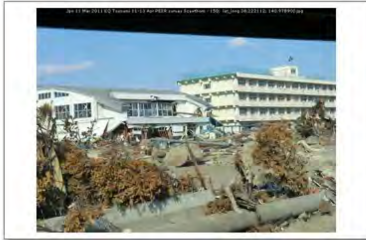
Jpn 11 Mar 2011 EQ Tsunami 11-13 Apr PEER survey Scawthorn - 150; lat_long 38.222112; 140.978900
