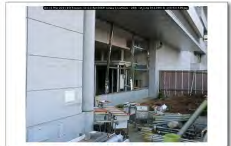
Jpn 11 Mar 2011 EQ Tsunami 11-13 Apr PEER survey Scawthorn - 268; lat_long 38.138018; 140.931435
