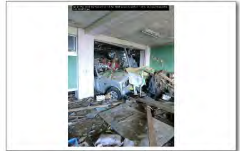
Jpn 11 Mar 2011 EQ Tsunami 11-13 Apr PEER survey Scawthorn - 169; lat_long 38.222268; 140.980453
