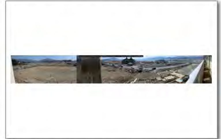
Jpn 11 Mar 2011 EQ Tsunami 11-13 Apr PEER survey Scawthorn - 331; lat_long 39.009822; 141.644580
