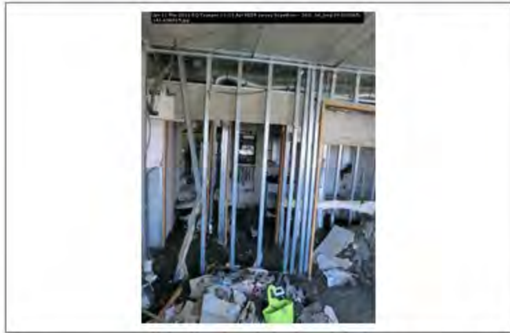
Jpn 11 Mar 2011 EQ Tsunami 11-13 Apr PEER survey Scawthorn - 303; lat_long 39.010065; 141.636015
