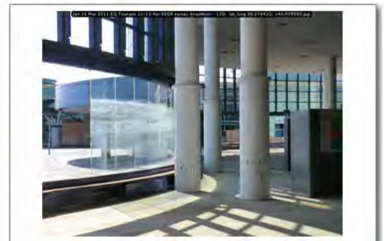
Jpn 11 Mar 2011 EQ Tsunami 11-13 Apr PEER survey Scawthorn - 133; lat_long 38.274422; 140.995550
