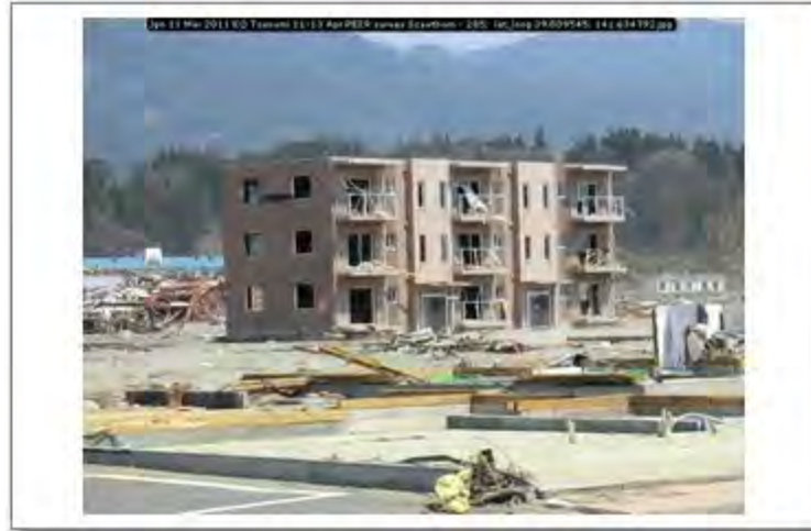
Jpn 11 Mar 2011 EQ Tsunami 11-13 Apr PEER survey Scawthorn - 285; lat_long 39.009545; 141.634792
