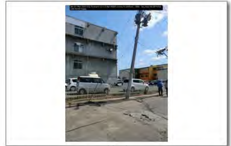
Jpn 11 Mar 2011 EQ Tsunami 11-13 Apr PEER survey Scawthorn - 086; lat_long 38.257692; 140.937873
