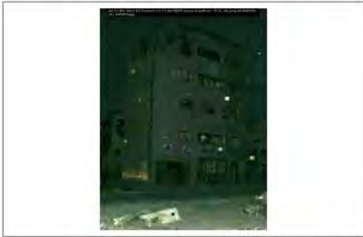
Jpn 11 Mar 2011 EQ Tsunami 11-13 Apr PEER survey Scawthorn - 513; lat_long 38.442438; 141.445453
