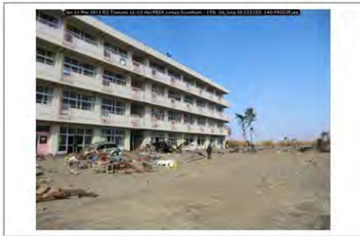
Jpn 11 Mar 2011 EQ Tsunami 11-13 Apr PEER survey Scawthorn - 159; lat_long 38.222223; 140.980235
