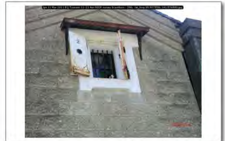
Jpn 11 Mar 2011 EQ Tsunami 11-13 Apr PEER survey Scawthorn - 396; lat_long 38.907558; 141.576880
