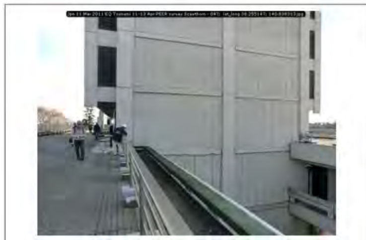
Jpn 11 Mar 2011 EQ Tsunami 11-13 Apr PEER survey Scawthorn - 047; lat_long 38.255147; 140.838313
