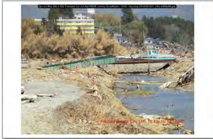
Jpn 11 Mar 2011 EQ Tsunami 11-13 Apr PEER survey Scawthorn - 339; lat_long 39.009247; 141.645688
