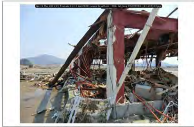
Jpn 11 Mar 2011 EQ Tsunami 11-13 Apr PEER survey Scawthorn - 288; lat_long 39.009853; 141.638132
