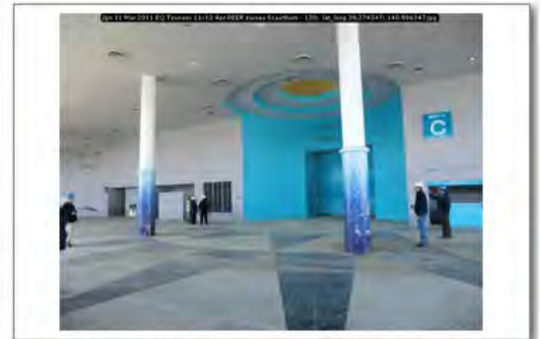
Jpn 11 Mar 2011 EQ Tsunami 11-13 Apr PEER survey Scawthorn - 130; lat_long 38.274347; 140.996347
