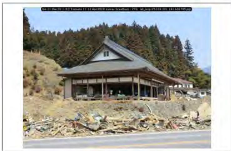
Jpn 11 Mar 2011 EQ Tsunami 11-13 Apr PEER survey Scawthorn - 276; lat_long 39.034183; 141.606785
