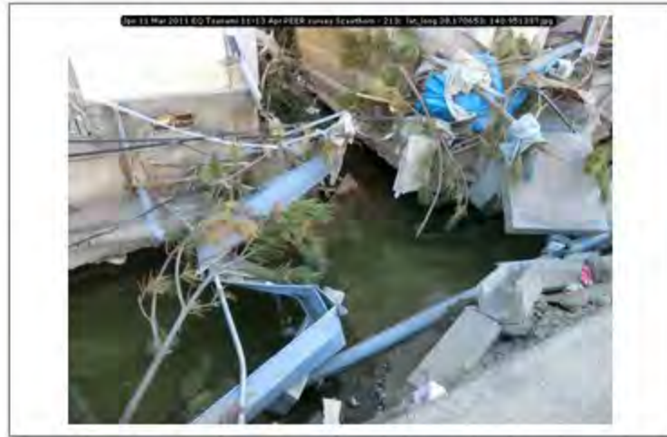
Jpn 11 Mar 2011 EQ Tsunami 11-13 Apr PEER survey Scawthorn - 213; lat_long 38.170653; 140.951337
