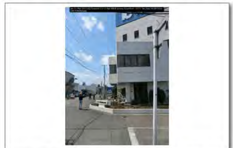
Jpn 11 Mar 2011 EQ Tsunami 11-13 Apr PEER survey Scawthorn - 077; lat_long 38.257532; 140.938260
