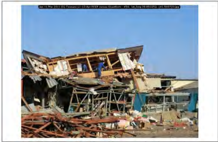
Jpn 11 Mar 2011 EQ Tsunami 11-13 Apr PEER survey Scawthorn - 454; lat_long 38.850252; 141.580723
