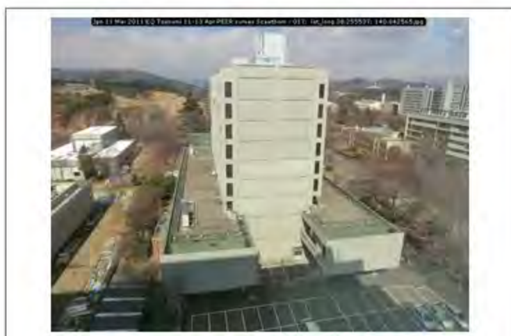
Jpn 11 Mar 2011 EQ Tsunami 11-13 Apr PEER survey Scawthorn - 017; lat_long 38.255537; 140.842565
