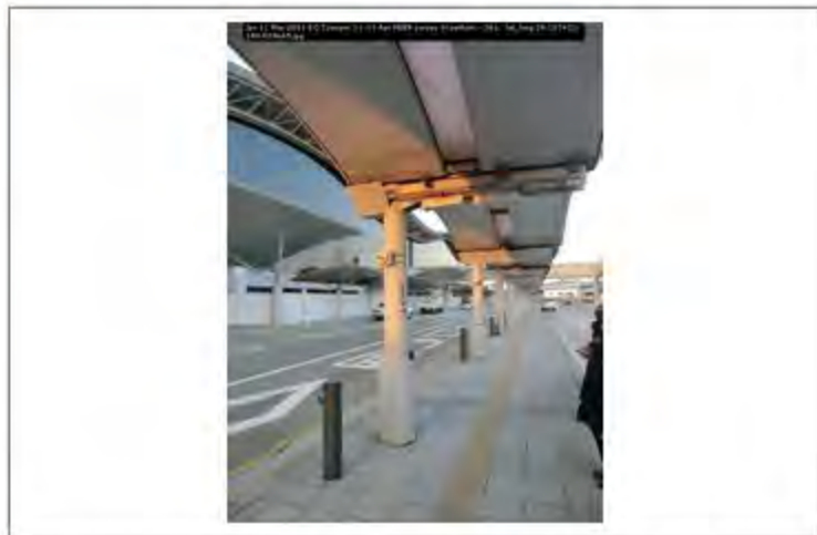
Jpn 11 Mar 2011 EQ Tsunami 11-13 Apr PEER survey Scawthorn - 261; lat_long 38.137422; 140.929665
