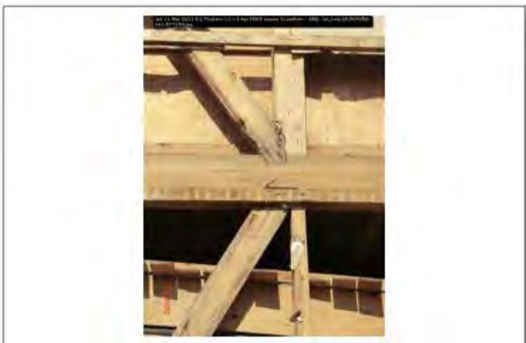
Jpn 11 Mar 2011 EQ Tsunami 11-13 Apr PEER survey Scawthorn - 388; lat_long 38.907658; 141.577150
