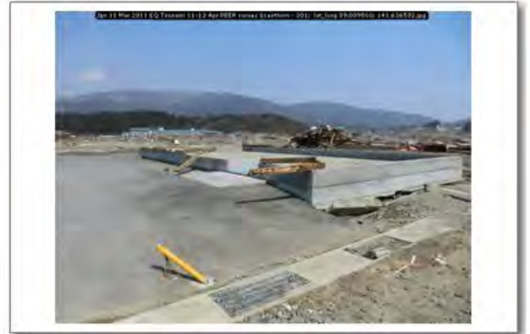
Jpn 11 Mar 2011 EQ Tsunami 11-13 Apr PEER survey Scawthorn - 301; lat_long 39.009560; 141.636532
