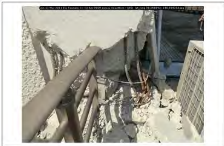
Jpn 11 Mar 2011 EQ Tsunami 11-13 Apr PEER survey Scawthorn - 040; lat_long 38.254892; 140.839268
