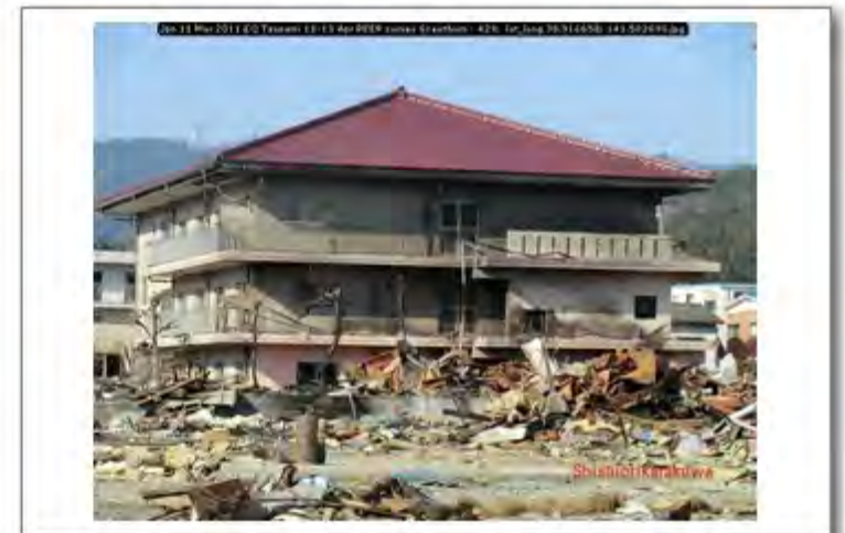
Jpn 11 Mar 2011 EQ Tsunami 11-13 Apr PEER survey Scawthorn - 429; lat_long 38.916658; 141.582698
