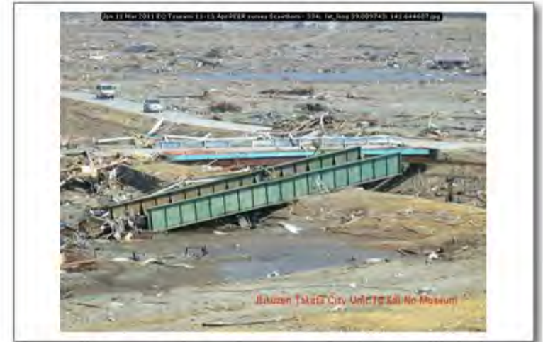
Jpn 11 Mar 2011 EQ Tsunami 11-13 Apr PEER survey Scawthorn - 334; lat_long 39.009743; 141.644607
