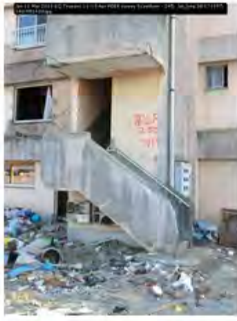
Jpn 11 Mar 2011 EQ Tsunami 11-13 Apr PEER survey Scawthorn - 245; lat_long 38.171397; 140.951433
