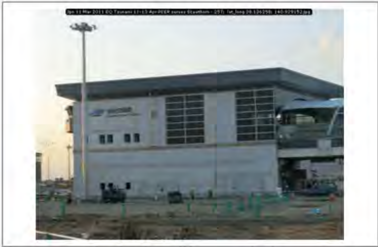
Jpn 11 Mar 2011 EQ Tsunami 11-13 Apr PEER survey Scawthorn - 257; lat_long 38.136258; 140.929152
