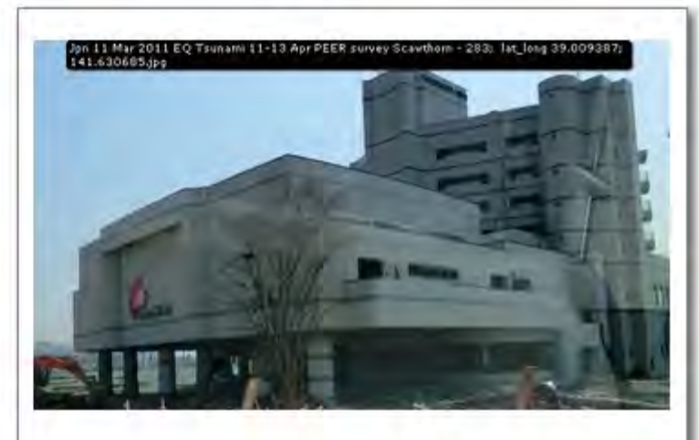
Jpn 11 Mar 2011 EQ Tsunami 11-13 Apr PEER survey Scawthorn - 283; lat_long 39.009387; 141.630685
