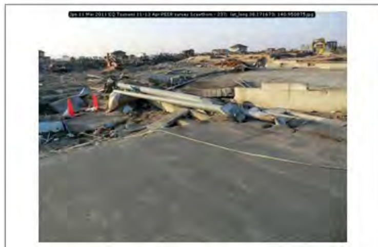
Jpn 11 Mar 2011 EQ Tsunami 11-13 Apr PEER survey Scawthorn - 237; lat_long 38.171673; 140.950875
