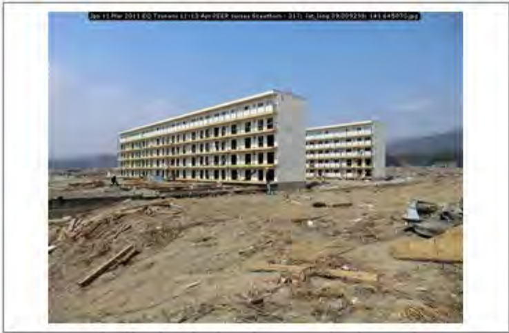
Jpn 11 Mar 2011 EQ Tsunami 11-13 Apr PEER survey Scawthorn - 317; lat_long 39.009298; 141.645070
