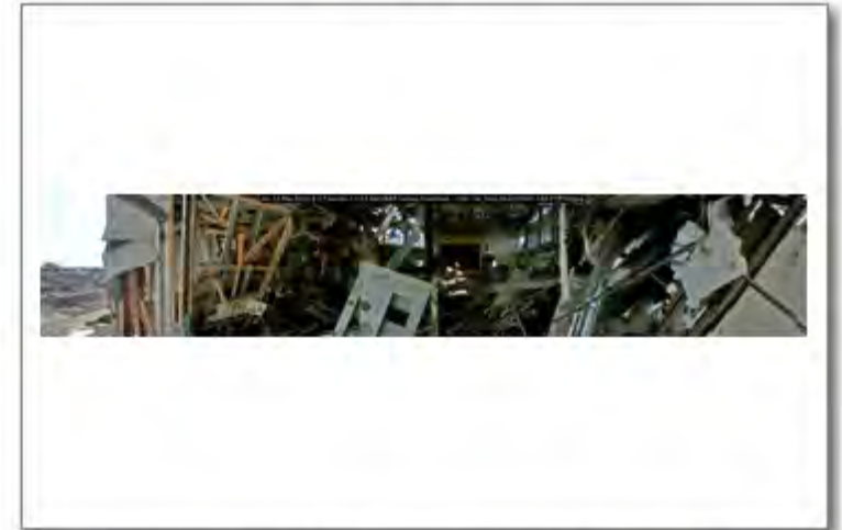
Jpn 11 Mar 2011 EQ Tsunami 11-13 Apr PEER survey Scawthorn - 154; lat_long 38.222383; 140.979703
