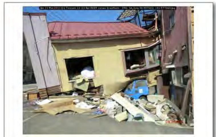
Jpn 11 Mar 2011 EQ Tsunami 11-13 Apr PEER survey Scawthorn - 390; lat_long 38.907682; 141.577060
