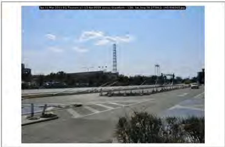
Jpn 11 Mar 2011 EQ Tsunami 11-13 Apr PEER survey Scawthorn - 128; lat_long 38.273862; 140.996365
