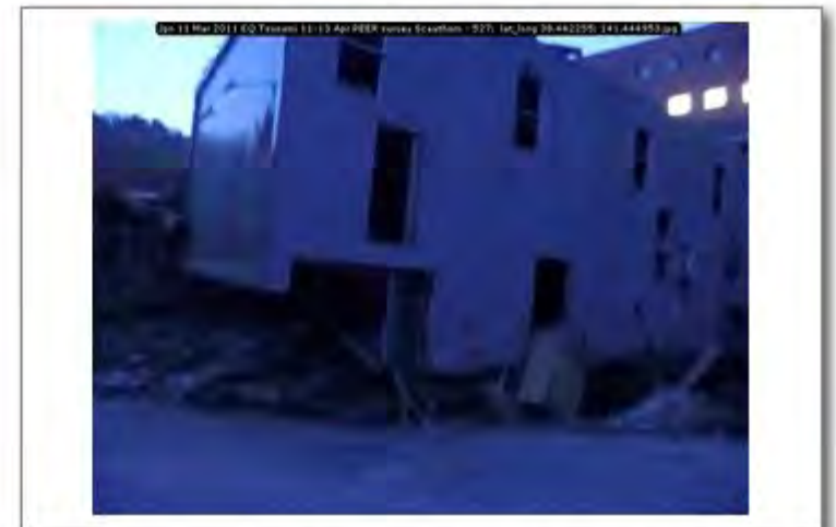
Jpn 11 Mar 2011 EQ Tsunami 11-13 Apr PEER survey Scawthorn - 527; lat_long 38.442255; 141.444953
