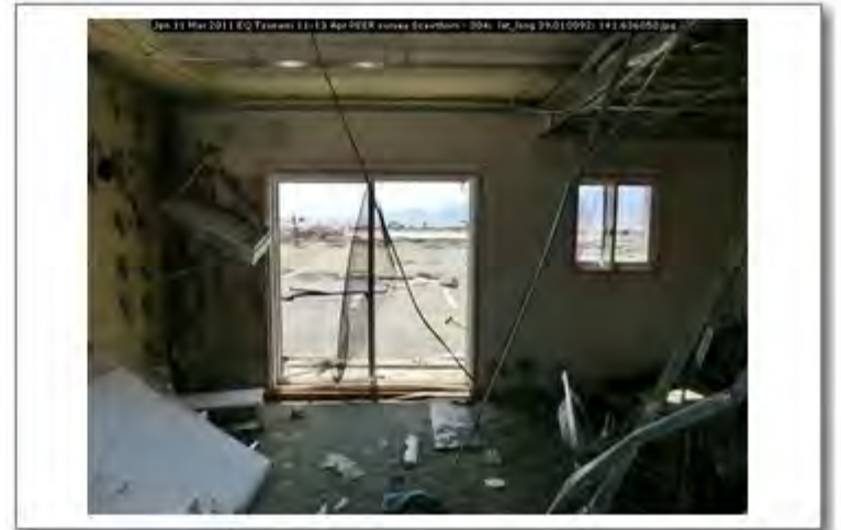
Jpn 11 Mar 2011 EQ Tsunami 11-13 Apr PEER survey Scawthorn - 304; lat_long 39.010092; 141.636050
