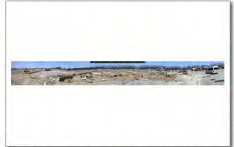
Jpn 11 Mar 2011 EQ Tsunami 11-13 Apr PEER survey Scawthorn - 286; lat_long 39.009532; 141.638258
