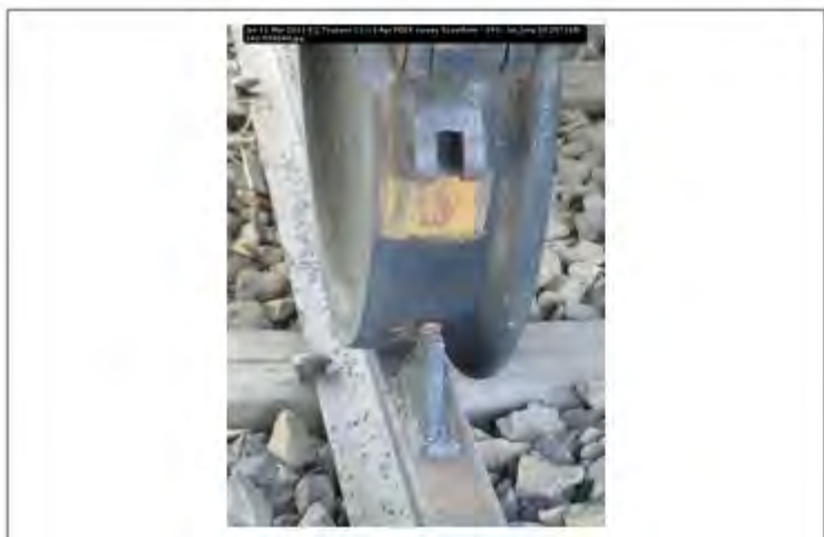
Jpn 11 Mar 2011 EQ Tsunami 11-13 Apr PEER survey Scawthorn - 093; lat_long 38.257165; 140.938048
