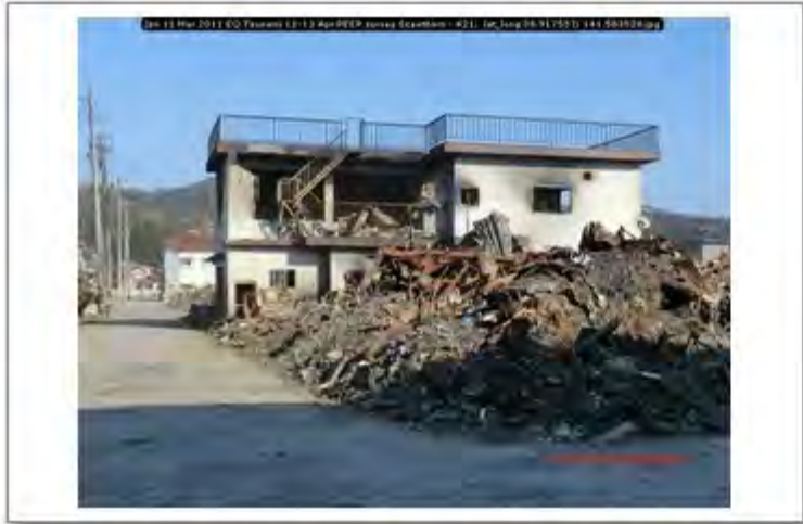
Jpn 11 Mar 2011 EQ Tsunami 11-13 Apr PEER survey Scawthorn - 421; lat_long 38.917557; 141.583528
