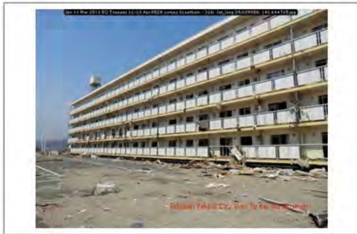
Jpn 11 Mar 2011 EQ Tsunami 11-13 Apr PEER survey Scawthorn - 324; lat_long 39.009858; 141.644715
