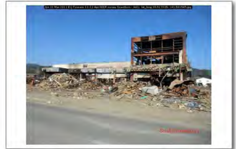
Jpn 11 Mar 2011 EQ Tsunami 11-13 Apr PEER survey Scawthorn - 441; lat_long 38.917335; 141.581545
