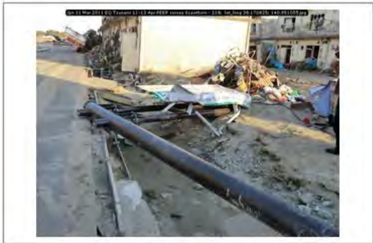
Jpn 11 Mar 2011 EQ Tsunami 11-13 Apr PEER survey Scawthorn - 218; lat_long 38.170825; 140.951055
