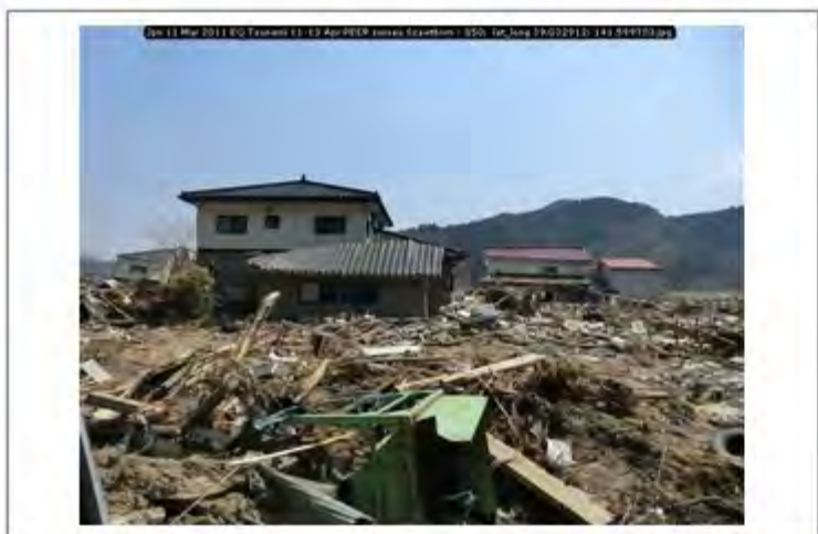
Jpn 11 Mar 2011 EQ Tsunami 11-13 Apr PEER survey Scawthorn - 350; lat_long 39.032912; 141.599703
