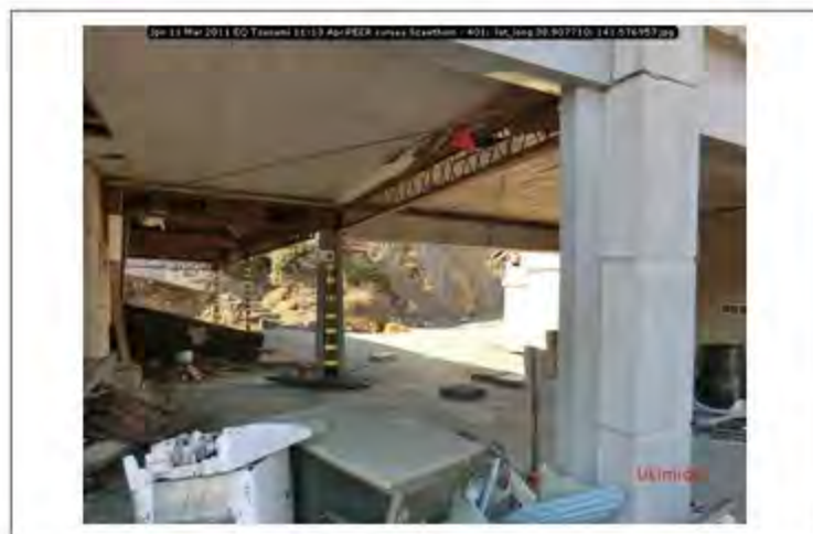
Jpn 11 Mar 2011 EQ Tsunami 11-13 Apr PEER survey Scawthorn - 401; lat_long 38.907710; 141.576957
