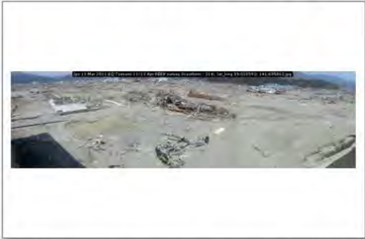
Jpn 11 Mar 2011 EQ Tsunami 11-13 Apr PEER survey Scawthorn - 314; lat_long 39.010592; 141.635862
