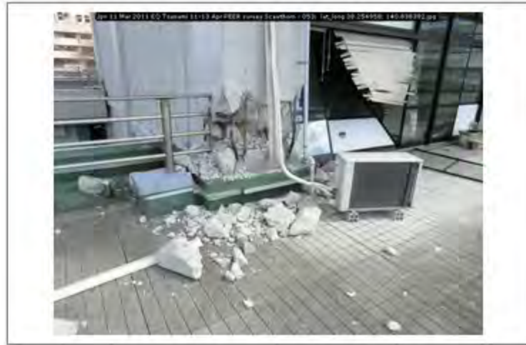
Jpn 11 Mar 2011 EQ Tsunami 11-13 Apr PEER survey Scawthorn - 053; lat_long 38.254958; 140.838382
