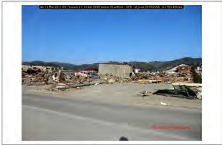
Jpn 11 Mar 2011 EQ Tsunami 11-13 Apr PEER survey Scawthorn - 439; lat_long 38.916558; 141.581400
