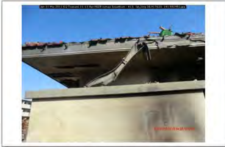
Jpn 11 Mar 2011 EQ Tsunami 11-13 Apr PEER survey Scawthorn - 413; lat_long 38.917623; 141.582952
