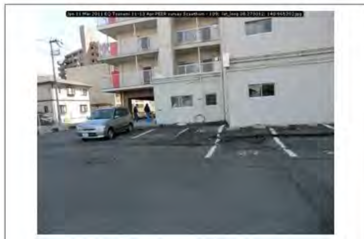
Jpn 11 Mar 2011 EQ Tsunami 11-13 Apr PEER survey Scawthorn - 109; lat_long 38.273012; 140.965202
