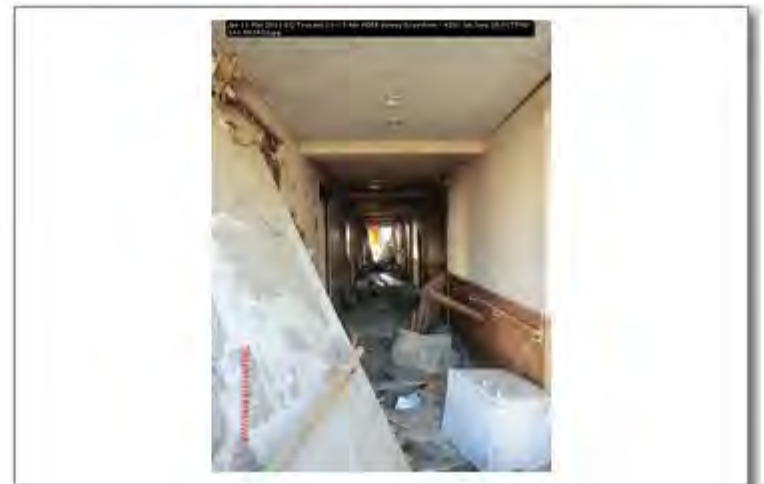
Jpn 11 Mar 2011 EQ Tsunami 11-13 Apr PEER survey Scawthorn - 420; lat_long 38.917590; 141.583433
