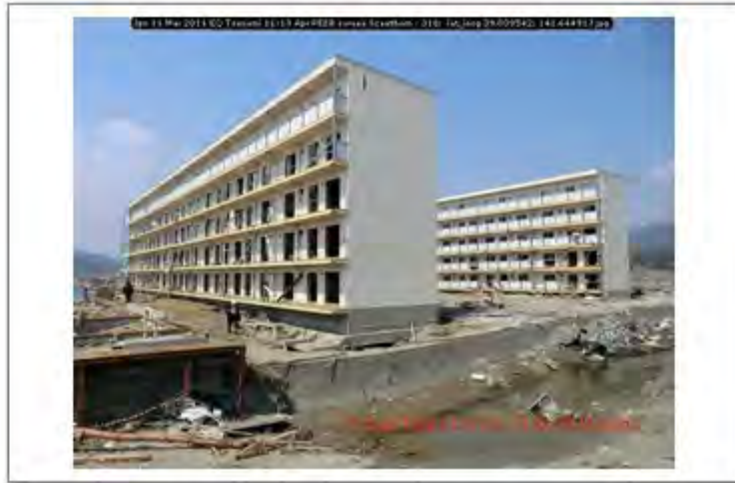
Jpn 11 Mar 2011 EQ Tsunami 11-13 Apr PEER survey Scawthorn - 318; lat_long 39.009542; 141.644917
