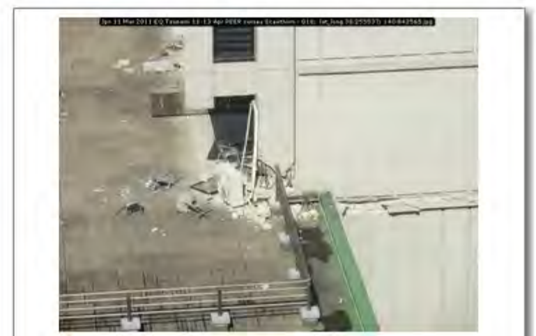
Jpn 11 Mar 2011 EQ Tsunami 11-13 Apr PEER survey Scawthorn - 018; lat_long 38.255537; 140.842565
