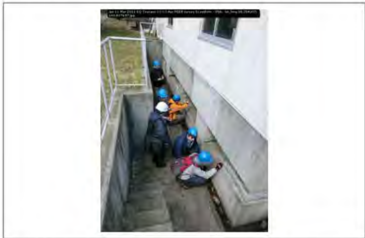
Jpn 11 Mar 2011 EQ Tsunami 11-13 Apr PEER survey Scawthorn - 058; lat_long 38.254307; 140.837697
