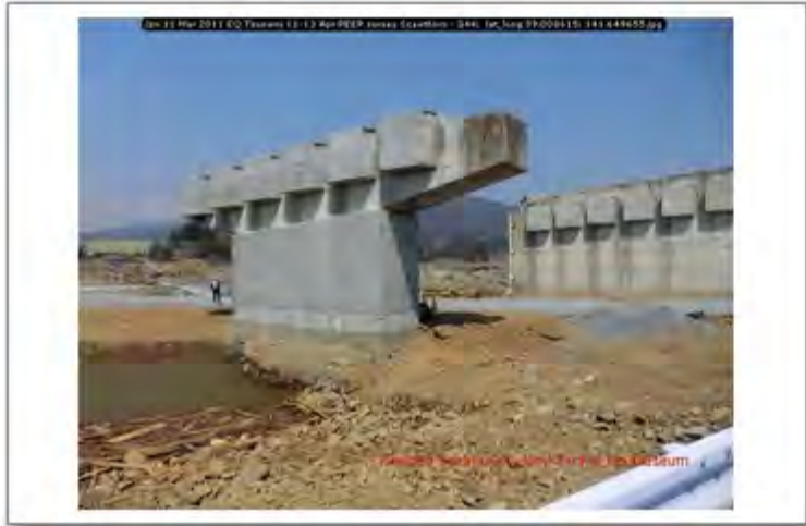
Jpn 11 Mar 2011 EQ Tsunami 11-13 Apr PEER survey Scawthorn - 344; lat_long 39.008615; 141.649655
