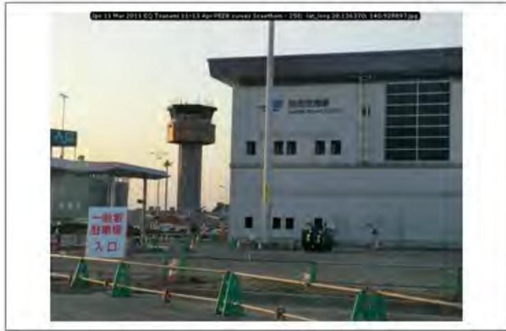
Jpn 11 Mar 2011 EQ Tsunami 11-13 Apr PEER survey Scawthorn - 258; lat_long 38.136370; 140.928897
