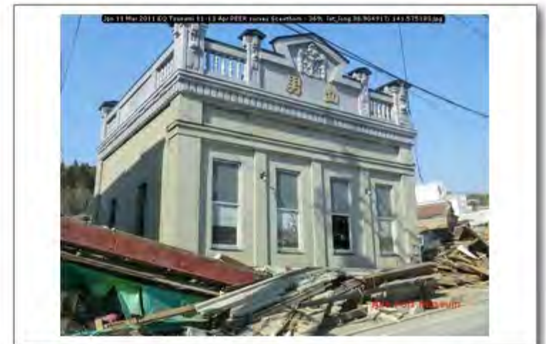
Jpn 11 Mar 2011 EQ Tsunami 11-13 Apr PEER survey Scawthorn - 369; lat_long 38.904917; 141.575183
