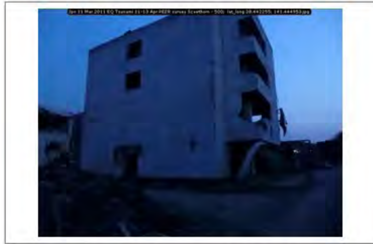
Jpn 11 Mar 2011 EQ Tsunami 11-13 Apr PEER survey Scawthorn - 500; lat_long 38.442255; 141.444953
