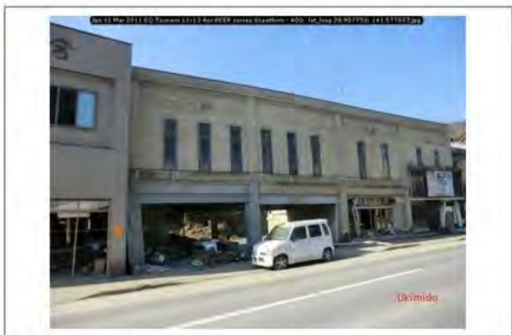
Jpn 11 Mar 2011 EQ Tsunami 11-13 Apr PEER survey Scawthorn - 400; lat_long 38.907753; 141.577037
