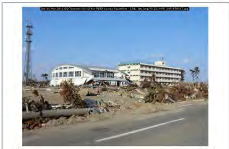
Jpn 11 Mar 2011 EQ Tsunami 11-13 Apr PEER survey Scawthorn - 191; lat_long 38.221997; 140.978917
