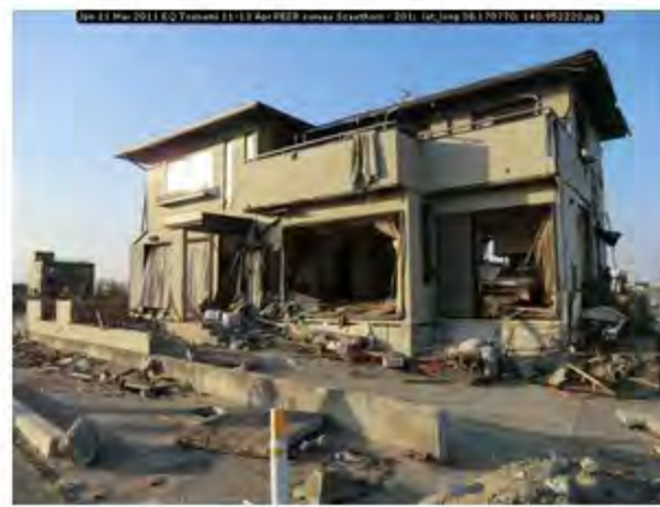
Jpn 11 Mar 2011 EQ Tsunami 11-13 Apr PEER survey Scawthorn - 201; lat_long 38.170770; 140.952220
