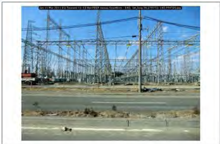
Jpn 11 Mar 2011 EQ Tsunami 11-13 Apr PEER survey Scawthorn - 140; lat_long 38.275772; 140.994720
