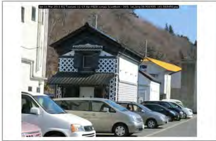
Jpn 11 Mar 2011 EQ Tsunami 11-13 Apr PEER survey Scawthorn - 365; lat_long 38.906935; 141.568450
