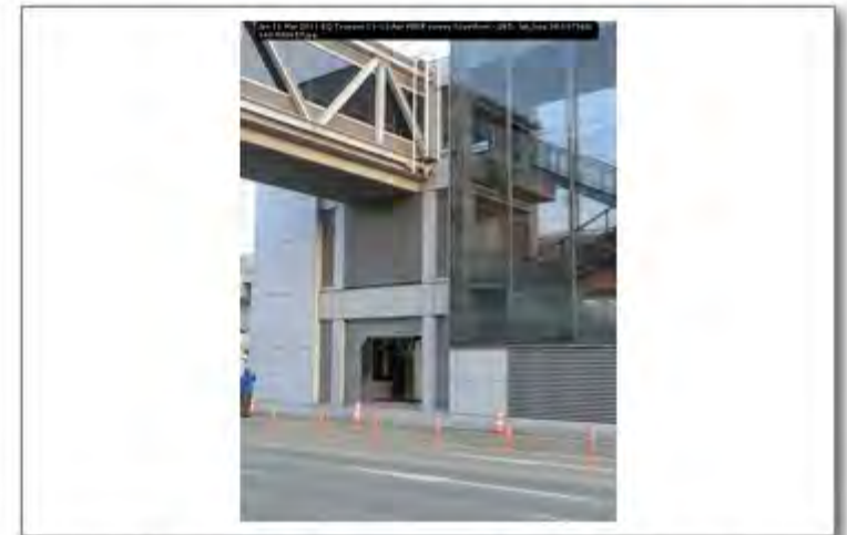
Jpn 11 Mar 2011 EQ Tsunami 11-13 Apr PEER survey Scawthorn - 265; lat_long 38.137568; 140.930657
