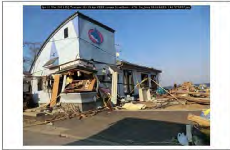
Jpn 11 Mar 2011 EQ Tsunami 11-13 Apr PEER survey Scawthorn - 470; lat_long 38.816283; 141.573307
