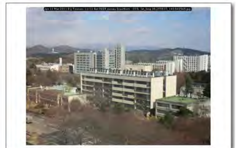
Jpn 11 Mar 2011 EQ Tsunami 11-13 Apr PEER survey Scawthorn - 015; lat_long 38.255537; 140.842565
