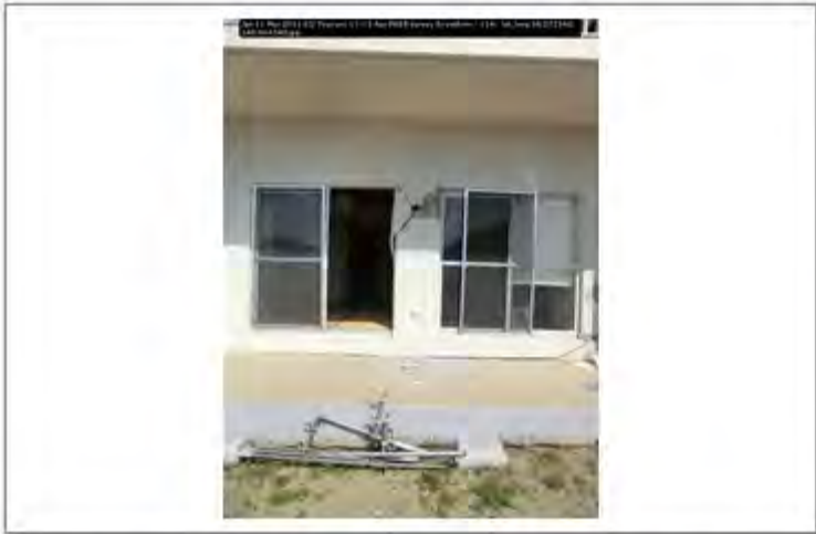
Jpn 11 Mar 2011 EQ Tsunami 11-13 Apr PEER survey Scawthorn - 114; lat_long 38.272342; 140.964243
