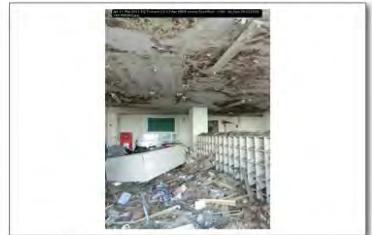
Jpn 11 Mar 2011 EQ Tsunami 11-13 Apr PEER survey Scawthorn - 160; lat_long 38.222323; 140.980362
