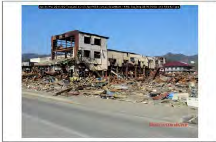
Jpn 11 Mar 2011 EQ Tsunami 11-13 Apr PEER survey Scawthorn - 440; lat_long 38.917043; 141.581427
