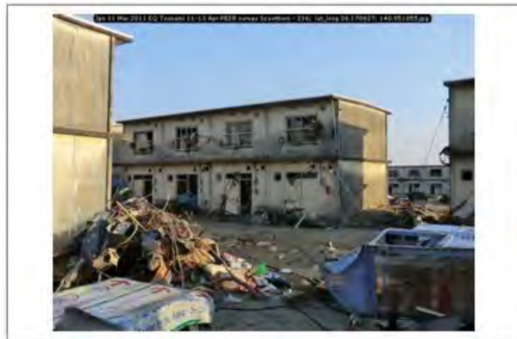
Jpn 11 Mar 2011 EQ Tsunami 11-13 Apr PEER survey Scawthorn - 216; lat_long 38.170827; 140.951055
