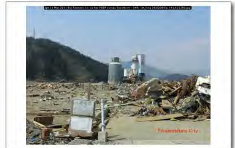
Jpn 11 Mar 2011 EQ Tsunami 11-13 Apr PEER survey Scawthorn - 349; lat_long 39.020683; 141.621250
