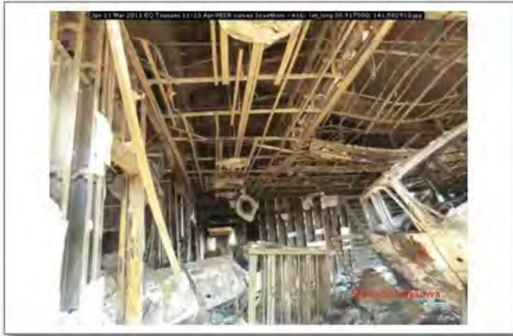
Jpn 11 Mar 2011 EQ Tsunami 11-13 Apr PEER survey Scawthorn - 416; lat_long 38.917500; 141.582913
