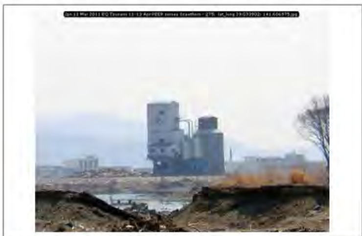
Jpn 11 Mar 2011 EQ Tsunami 11-13 Apr PEER survey Scawthorn - 275; lat_long 39.033902; 141.606975
