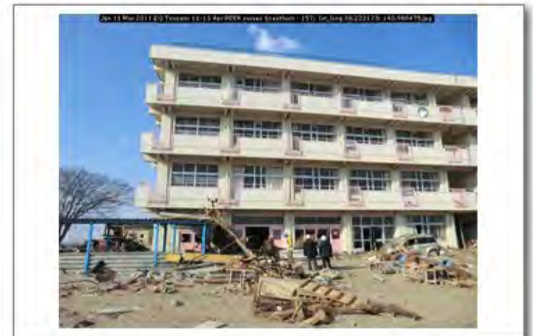
Jpn 11 Mar 2011 EQ Tsunami 11-13 Apr PEER survey Scawthorn - 157; lat_long 38.222173; 140.980475
