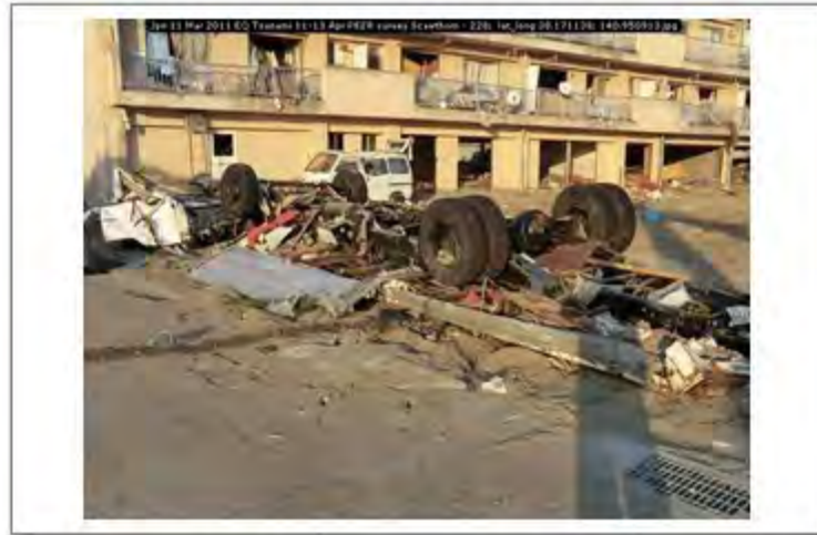
Jpn 11 Mar 2011 EQ Tsunami 11-13 Apr PEER survey Scawthorn - 228; lat_long 38.171138; 140.950913
