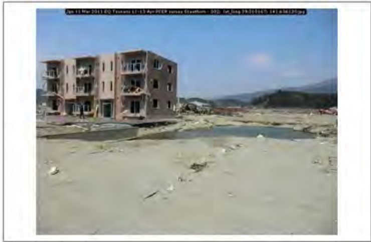
Jpn 11 Mar 2011 EQ Tsunami 11-13 Apr PEER survey Scawthorn - 302; lat_long 39.010167; 141.636120
