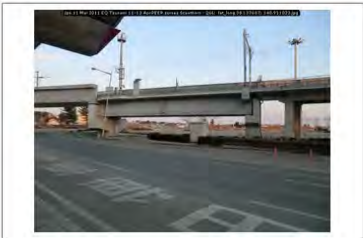
Jpn 11 Mar 2011 EQ Tsunami 11-13 Apr PEER survey Scawthorn - 266; lat_long 38.137687; 140.931023
