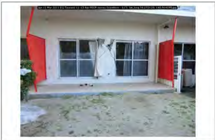
Jpn 11 Mar 2011 EQ Tsunami 11-13 Apr PEER survey Scawthorn - 117; lat_long 38.272128; 140.964095
