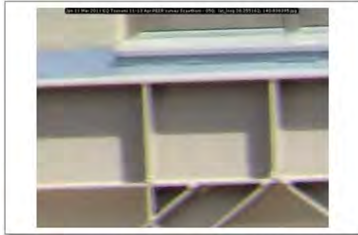
Jpn 11 Mar 2011 EQ Tsunami 11-13 Apr PEER survey Scawthorn - 050; lat_long 38.255162; 140.838395
