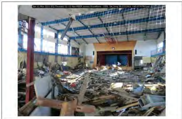
Jpn 11 Mar 2011 EQ Tsunami 11-13 Apr PEER survey Scawthorn - 155; lat_long 38.222262; 140.979750
