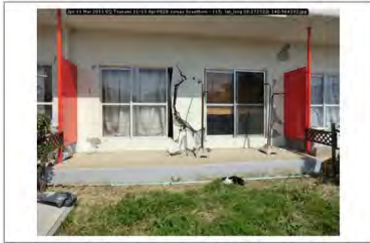
Jpn 11 Mar 2011 EQ Tsunami 11-13 Apr PEER survey Scawthorn - 115; lat_long 38.272323; 140.964232
