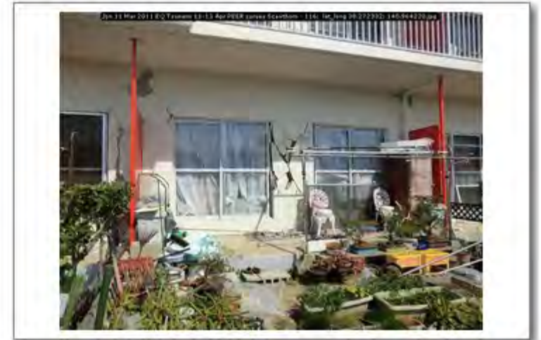
Jpn 11 Mar 2011 EQ Tsunami 11-13 Apr PEER survey Scawthorn - 116; lat_long 38.272332; 140.964220
