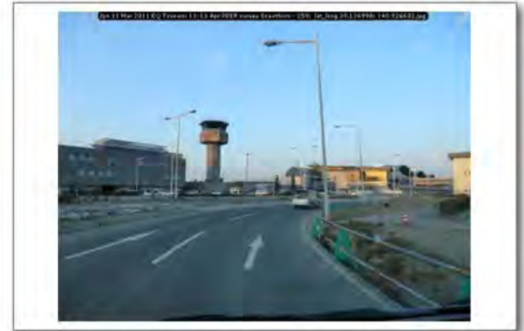
Jpn 11 Mar 2011 EQ Tsunami 11-13 Apr PEER survey Scawthorn - 259; lat_long 38.136998; 140.926632
