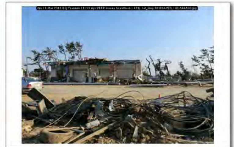
Jpn 11 Mar 2011 EQ Tsunami 11-13 Apr PEER survey Scawthorn - 474; lat_long 38.814257; 141.566530
