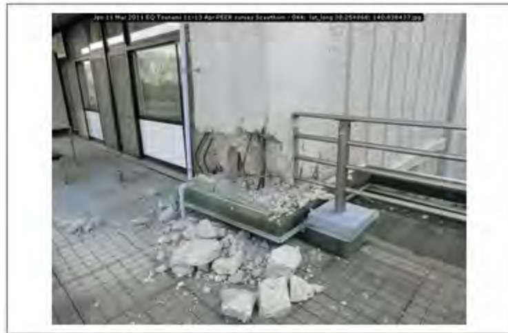
Jpn 11 Mar 2011 EQ Tsunami 11-13 Apr PEER survey Scawthorn - 044; lat_long 38.254868; 140.838437
