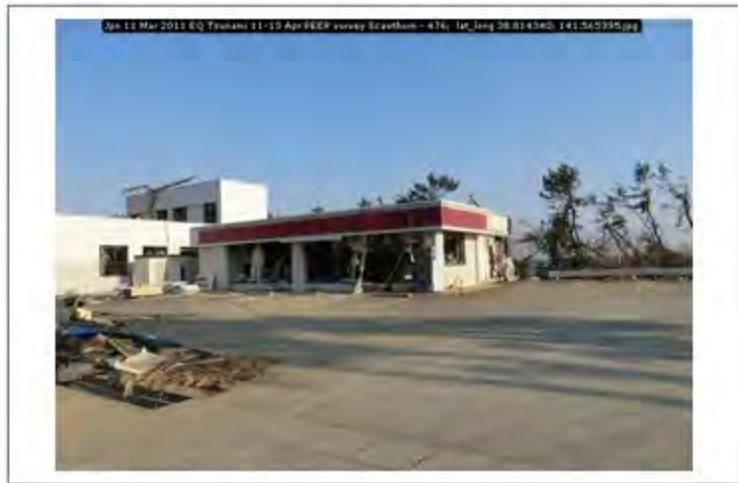
Jpn 11 Mar 2011 EQ Tsunami 11-13 Apr PEER survey Scawthorn - 476; lat_long 38.814340; 141.565395
