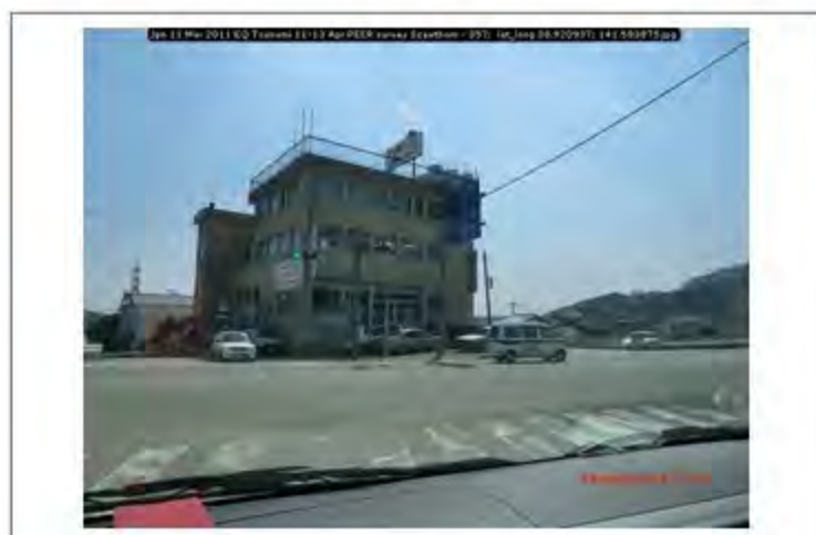
Jpn 11 Mar 2011 EQ Tsunami 11-13 Apr PEER survey Scawthorn - 357; lat_long 38.920937; 141.583875
