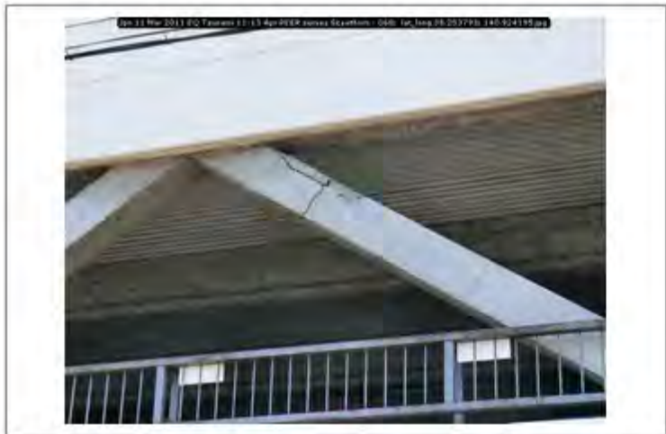
Jpn 11 Mar 2011 EQ Tsunami 11-13 Apr PEER survey Scawthorn - 068; lat_long 38.253793; 140.924195
