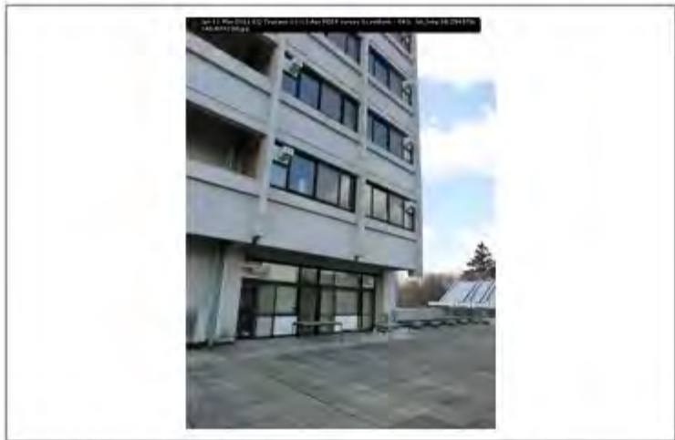
Jpn 11 Mar 2011 EQ Tsunami 11-13 Apr PEER survey Scawthorn - 043; lat_long 38.254978; 140.839238
