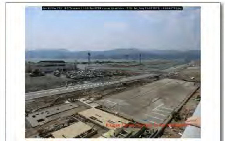
Jpn 11 Mar 2011 EQ Tsunami 11-13 Apr PEER survey Scawthorn - 328; lat_long 39.009872; 141.644783
