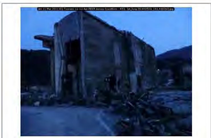
Jpn 11 Mar 2011 EQ Tsunami 11-13 Apr PEER survey Scawthorn - 493; lat_long 38.440923; 141.446360
