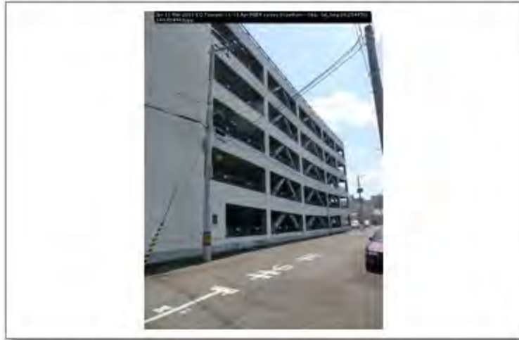
Jpn 11 Mar 2011 EQ Tsunami 11-13 Apr PEER survey Scawthorn - 066; lat_long 38.254450; 140.924963
