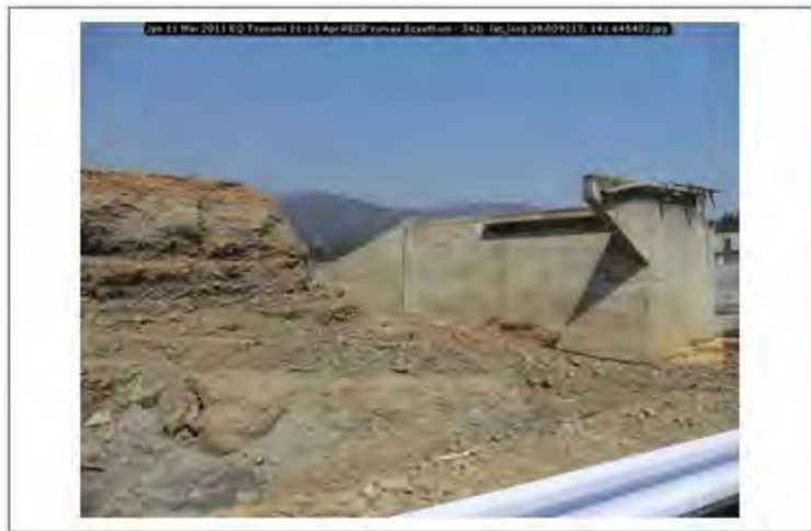
Jpn 11 Mar 2011 EQ Tsunami 11-13 Apr PEER survey Scawthorn - 342; lat_long 39.009217; 141.645402
