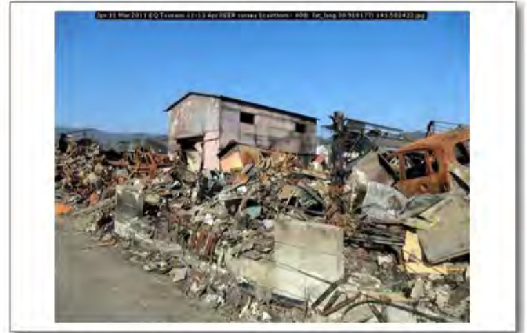
Jpn 11 Mar 2011 EQ Tsunami 11-13 Apr PEER survey Scawthorn - 408; lat_long 38.918177; 141.582422
