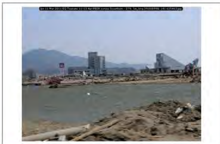
Jpn 11 Mar 2011 EQ Tsunami 11-13 Apr PEER survey Scawthorn - 279; lat_long 39.008998; 141.625463
