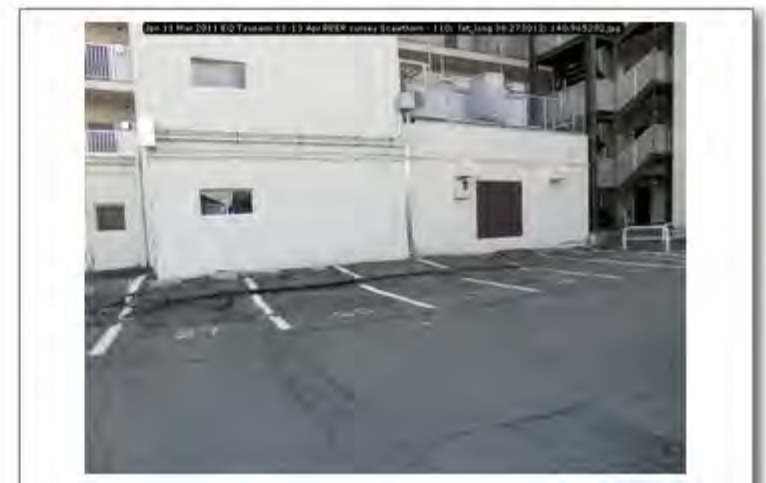
Jpn 11 Mar 2011 EQ Tsunami 11-13 Apr PEER survey Scawthorn - 110; lat_long 38.273012; 140.965202
