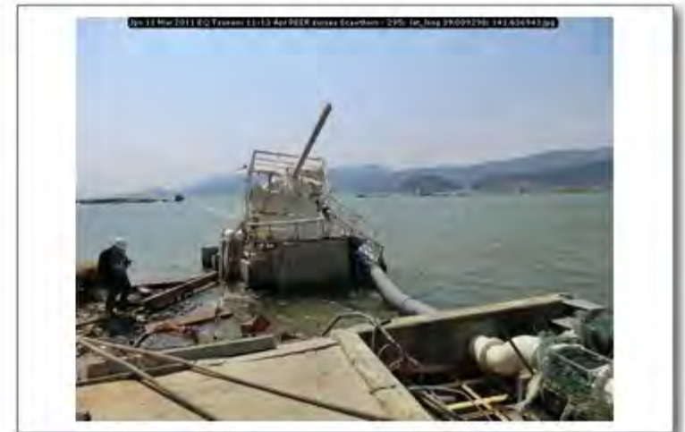
Jpn 11 Mar 2011 EQ Tsunami 11-13 Apr PEER survey Scawthorn - 295; lat_long 39.009298; 141.636943
