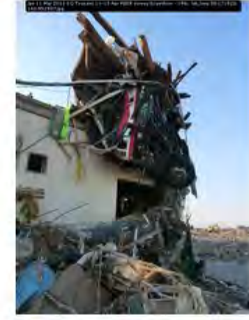
Jpn 11 Mar 2011 EQ Tsunami 11-13 Apr PEER survey Scawthorn - 196; lat_long 38.171823; 140.952937
