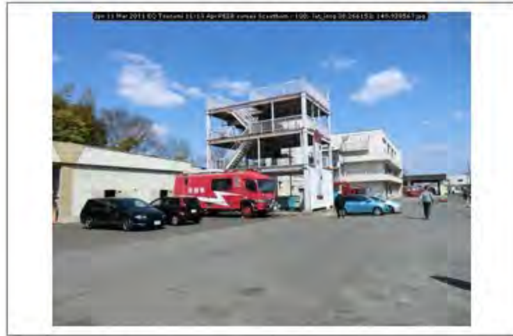
Jpn 11 Mar 2011 EQ Tsunami 11-13 Apr PEER survey Scawthorn - 100; lat_long 38.266153; 140.928567
