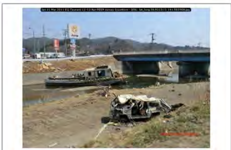
Jpn 11 Mar 2011 EQ Tsunami 11-13 Apr PEER survey Scawthorn - 356; lat_long 38.921317; 141.583908
