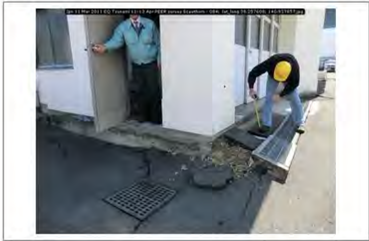
Jpn 11 Mar 2011 EQ Tsunami 11-13 Apr PEER survey Scawthorn - 084; lat_long 38.257608; 140.937857
