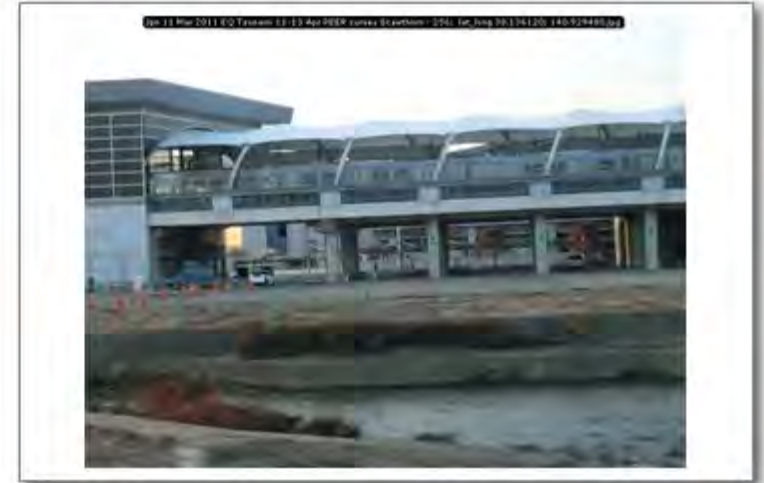
Jpn 11 Mar 2011 EQ Tsunami 11-13 Apr PEER survey Scawthorn - 256; lat_long 38.136120; 140.929480
