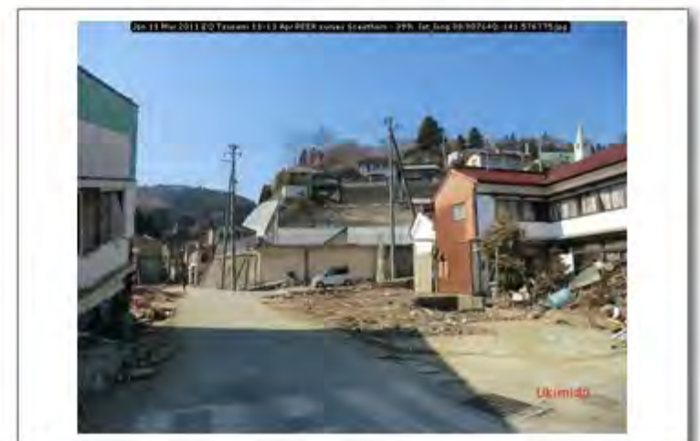
Jpn 11 Mar 2011 EQ Tsunami 11-13 Apr PEER survey Scawthorn - 399; lat_long 38.907640; 141.576775
