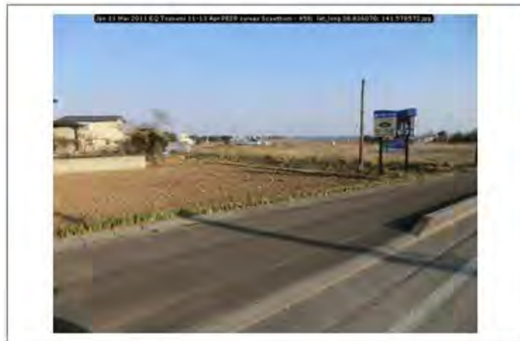
Jpn 11 Mar 2011 EQ Tsunami 11-13 Apr PEER survey Scawthorn - 458; lat_long 38.836070; 141.578572
