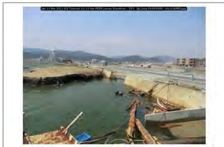
Jpn 11 Mar 2011 EQ Tsunami 11-13 Apr PEER survey Scawthorn - 297; lat_long 39.009305; 141.636950
