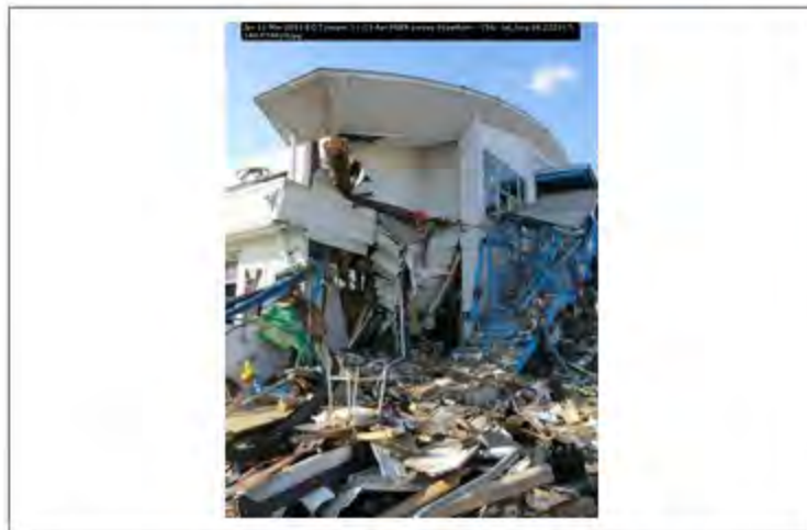
Jpn 11 Mar 2011 EQ Tsunami 11-13 Apr PEER survey Scawthorn - 156; lat_long 38.222317; 140.979828
