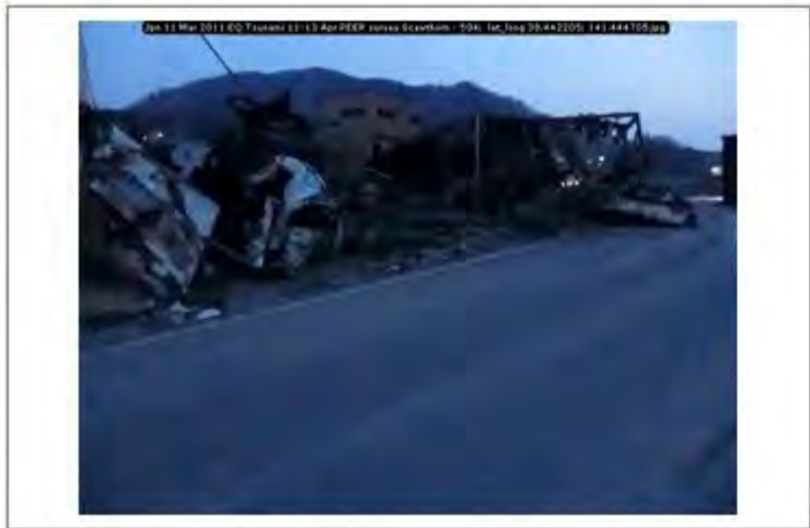
Jpn 11 Mar 2011 EQ Tsunami 11-13 Apr PEER survey Scawthorn - 504; lat_long 38.442205; 141.444705
