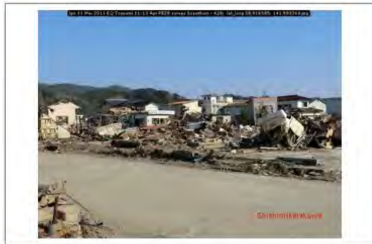
Jpn 11 Mar 2011 EQ Tsunami 11-13 Apr PEER survey Scawthorn - 428; lat_long 38.916585; 141.583268
