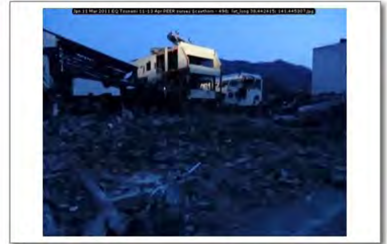
Jpn 11 Mar 2011 EQ Tsunami 11-13 Apr PEER survey Scawthorn - 498; lat_long 38.442415; 141.445307
