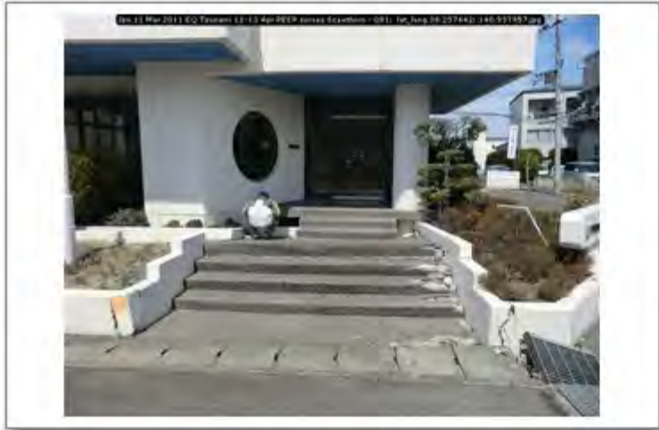
Jpn 11 Mar 2011 EQ Tsunami 11-13 Apr PEER survey Scawthorn - 081; lat_long 38.257442; 140.937957
