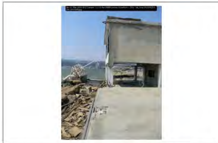
Jpn 11 Mar 2011 EQ Tsunami 11-13 Apr PEER survey Scawthorn - 291; lat_long 39.009253; 141.637165
