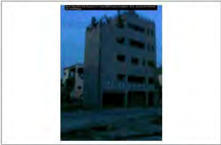
Jpn 11 Mar 2011 EQ Tsunami 11-13 Apr PEER survey Scawthorn - 512; lat_long 38.442438; 141.445455
