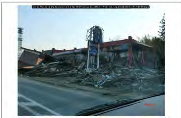
Jpn 11 Mar 2011 EQ Tsunami 11-13 Apr PEER survey Scawthorn - 448; lat_long 38.853807; 141.580482
