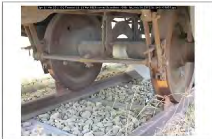
Jpn 11 Mar 2011 EQ Tsunami 11-13 Apr PEER survey Scawthorn - 088; lat_long 38.257220; 140.937857
