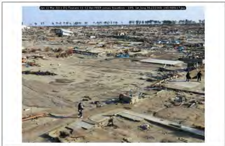
Jpn 11 Mar 2011 EQ Tsunami 11-13 Apr PEER survey Scawthorn - 185; lat_long 38.222348; 140.980617
