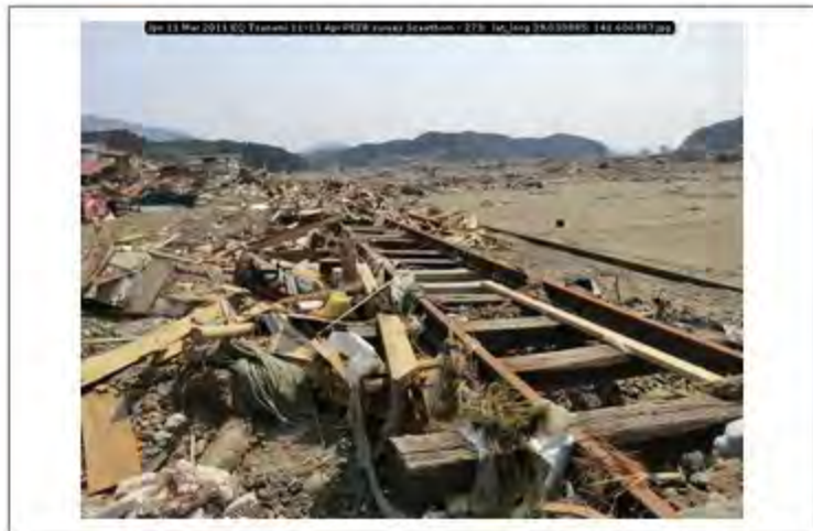
Jpn 11 Mar 2011 EQ Tsunami 11-13 Apr PEER survey Scawthorn - 273; lat_long 39.033885; 141.606987
