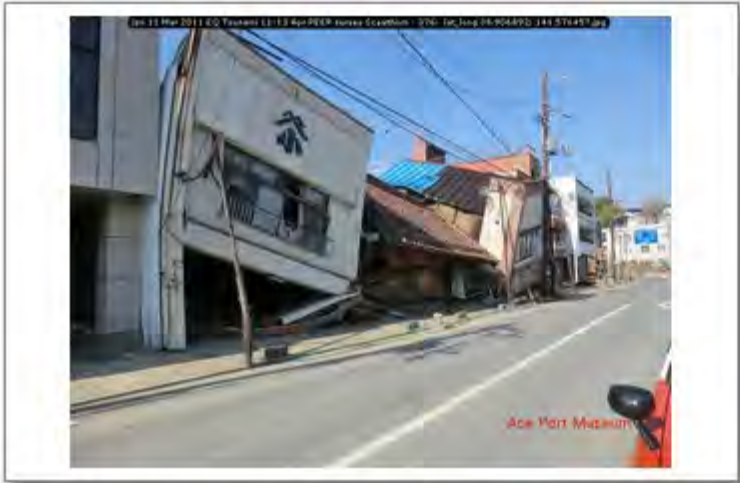
Jpn 11 Mar 2011 EQ Tsunami 11-13 Apr PEER survey Scawthorn - 376; lat_long 38.906892; 141.576457
