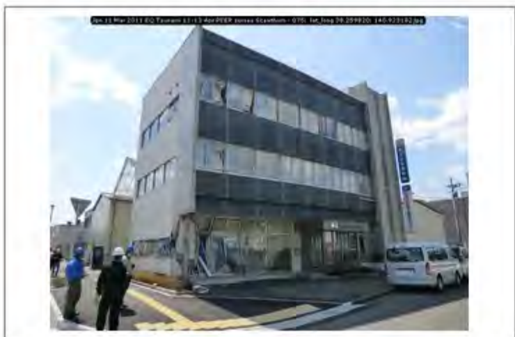
Jpn 11 Mar 2011 EQ Tsunami 11-13 Apr PEER survey Scawthorn - 075; lat_long 38.259820; 140.923182
