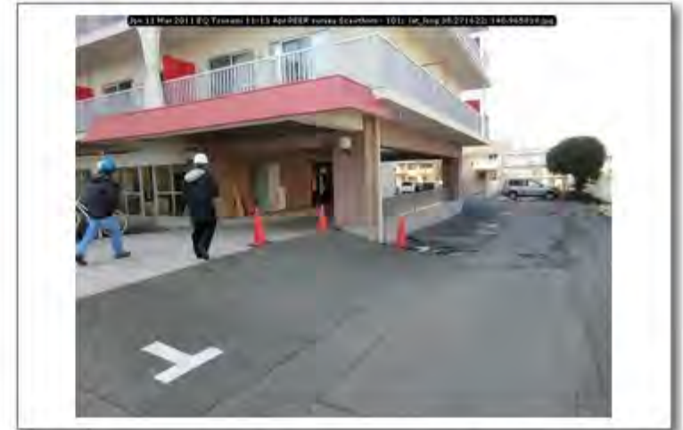
Jpn 11 Mar 2011 EQ Tsunami 11-13 Apr PEER survey Scawthorn - 101; lat_long 38.271622; 140.965818
