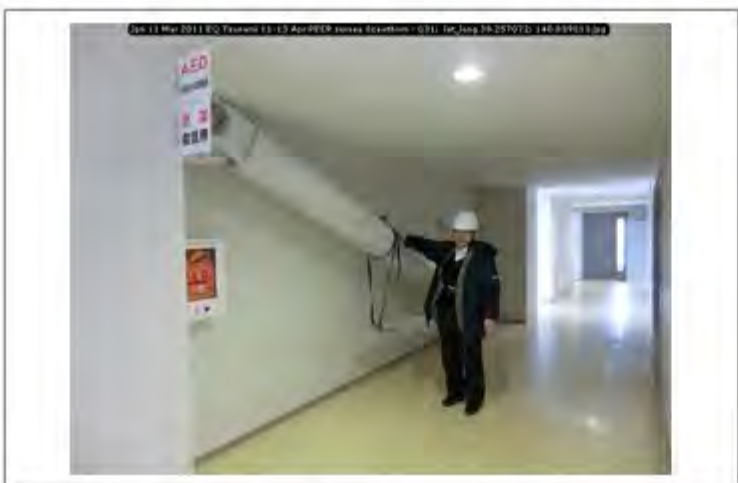
Jpn 11 Mar 2011 EQ Tsunami 11-13 Apr PEER survey Scawthorn - 031; lat_long 38.257072; 140.839013
