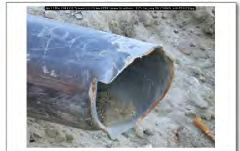
Jpn 11 Mar 2011 EQ Tsunami 11-13 Apr PEER survey Scawthorn - 217; lat_long 38.170843; 140.951022
