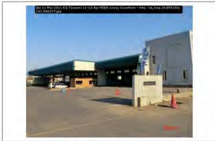
Jpn 11 Mar 2011 EQ Tsunami 11-13 Apr PEER survey Scawthorn - 446; lat_long 38.855183; 141.580377
