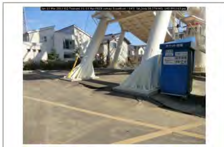
Jpn 11 Mar 2011 EQ Tsunami 11-13 Apr PEER survey Scawthorn - 147; lat_long 38.274943; 140.991163
