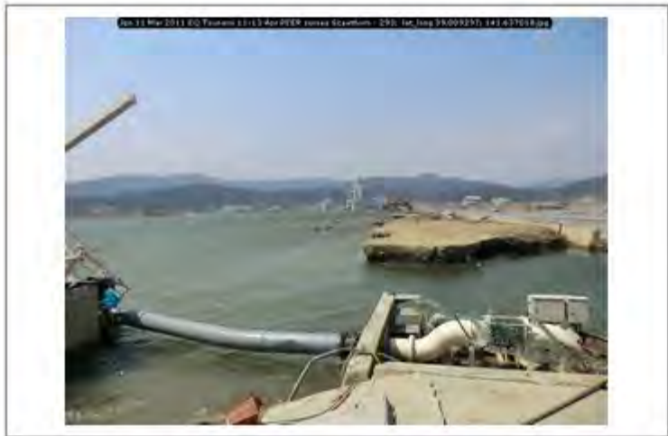
Jpn 11 Mar 2011 EQ Tsunami 11-13 Apr PEER survey Scawthorn - 293; lat_long 39.009297; 141.637018
