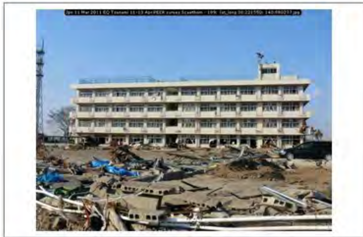
Jpn 11 Mar 2011 EQ Tsunami 11-13 Apr PEER survey Scawthorn - 189; lat_long 38.221550; 140.980237
