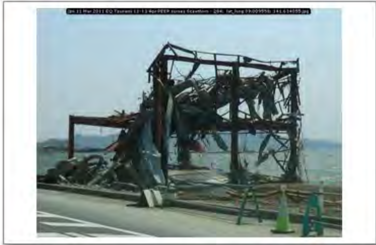
Jpn 11 Mar 2011 EQ Tsunami 11-13 Apr PEER survey Scawthorn - 284; lat_long 39.009558; 141.634055
