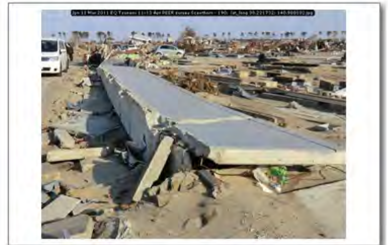
Jpn 11 Mar 2011 EQ Tsunami 11-13 Apr PEER survey Scawthorn - 190; lat_long 38.221732; 140.980102
