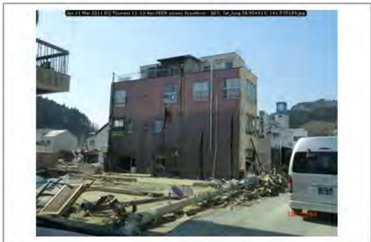
Jpn 11 Mar 2011 EQ Tsunami 11-13 Apr PEER survey Scawthorn - 367; lat_long 38.904917; 141.575183
