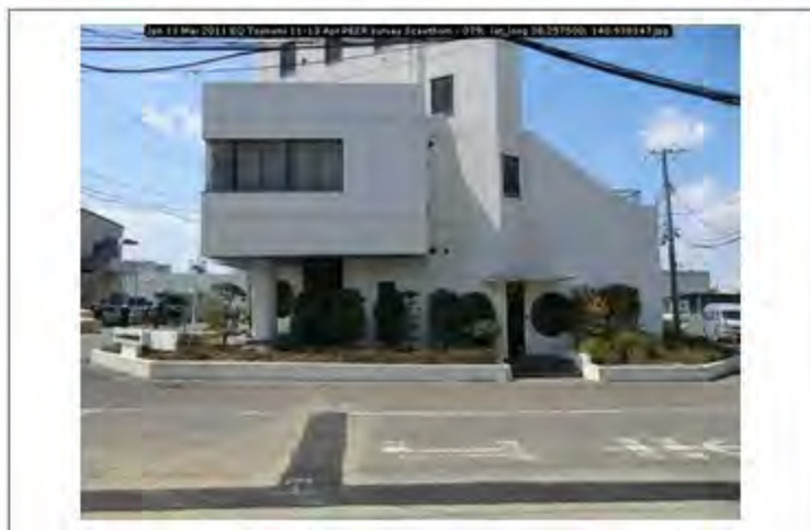
Jpn 11 Mar 2011 EQ Tsunami 11-13 Apr PEER survey Scawthorn - 079; lat_long 38.257500; 140.938147
