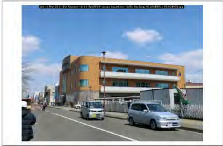
Jpn 11 Mar 2011 EQ Tsunami 11-13 Apr PEER survey Scawthorn - 065; lat_long 38.254555; 140.924502
