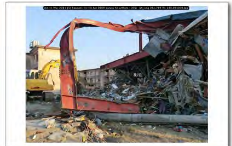
Jpn 11 Mar 2011 EQ Tsunami 11-13 Apr PEER survey Scawthorn - 232; lat_long 38.171575; 140.951005
