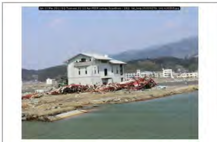
Jpn 11 Mar 2011 EQ Tsunami 11-13 Apr PEER survey Scawthorn - 282; lat_long 39.009270; 141.630205
