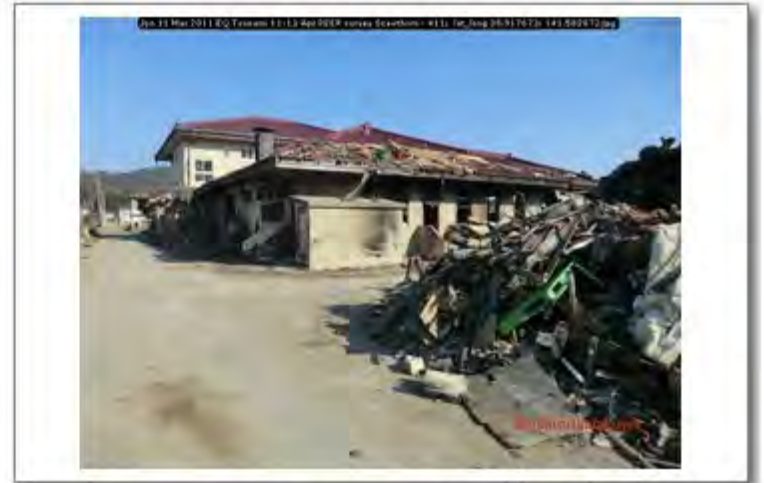
Jpn 11 Mar 2011 EQ Tsunami 11-13 Apr PEER survey Scawthorn - 411; lat_long 38.917673; 141.582872
