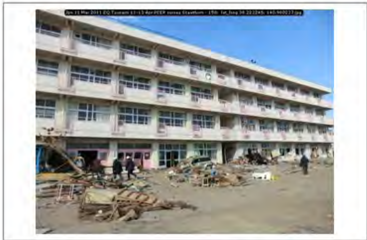
Jpn 11 Mar 2011 EQ Tsunami 11-13 Apr PEER survey Scawthorn - 158; lat_long 38.222245; 140.980227
