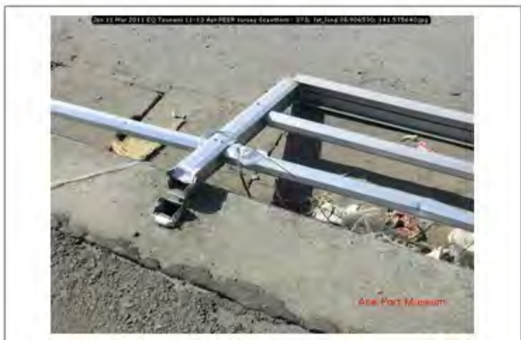
Jpn 11 Mar 2011 EQ Tsunami 11-13 Apr PEER survey Scawthorn - 373; lat_long 38.906530; 141.575640
