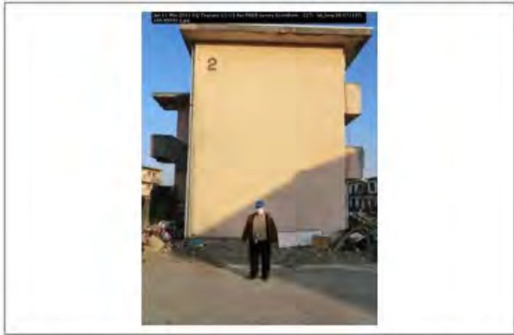
Jpn 11 Mar 2011 EQ Tsunami 11-13 Apr PEER survey Scawthorn - 227; lat_long 38.171137; 140.950912
