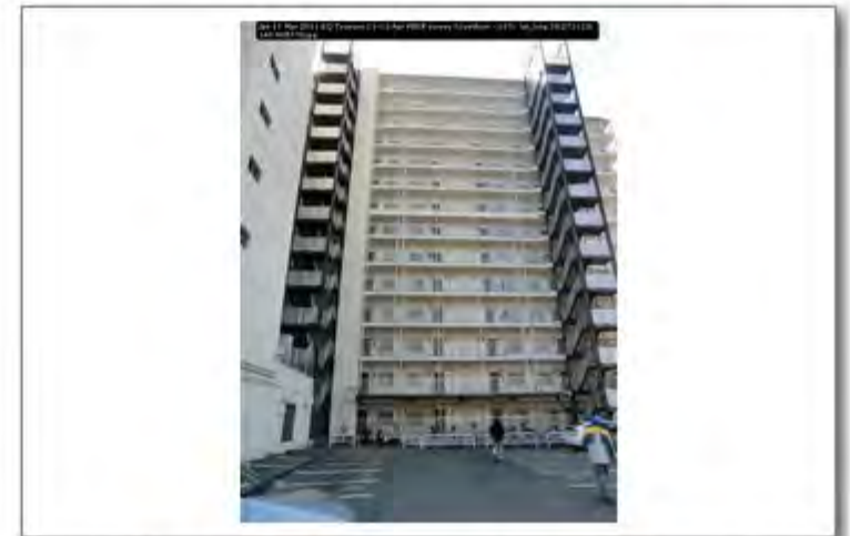
Jpn 11 Mar 2011 EQ Tsunami 11-13 Apr PEER survey Scawthorn - 107; lat_long 38.272123; 140.965370
