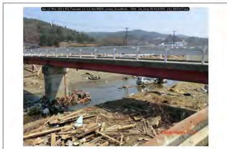
Jpn 11 Mar 2011 EQ Tsunami 11-13 Apr PEER survey Scawthorn - 354; lat_long 38.923255; 141.583347
