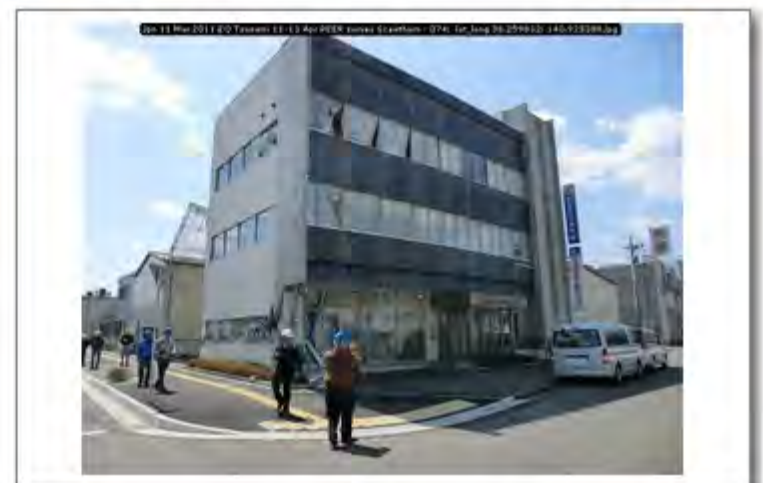
Jpn 11 Mar 2011 EQ Tsunami 11-13 Apr PEER survey Scawthorn - 074; lat_long 38.259832; 140.923388
