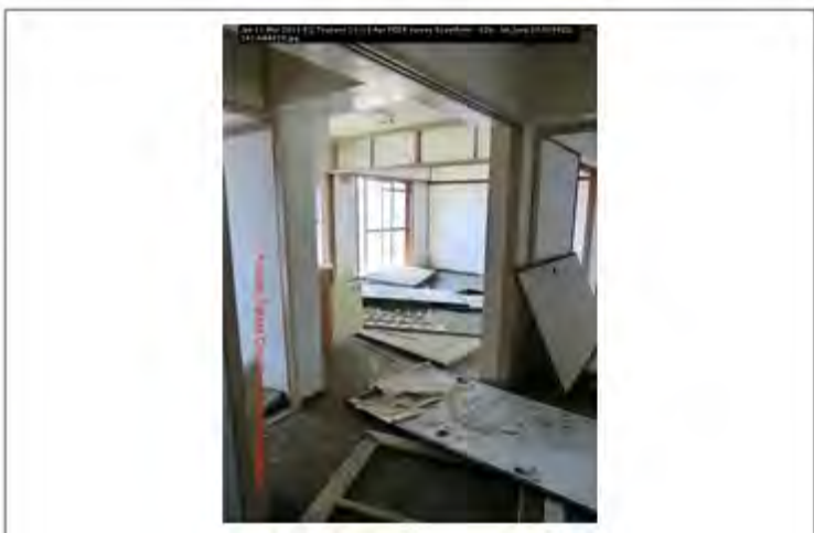
Jpn 11 Mar 2011 EQ Tsunami 11-13 Apr PEER survey Scawthorn - 326; lat_long 39.009822; 141.644818
