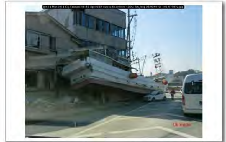
Jpn 11 Mar 2011 EQ Tsunami 11-13 Apr PEER survey Scawthorn - 366; lat_long 38.904873; 141.577872
