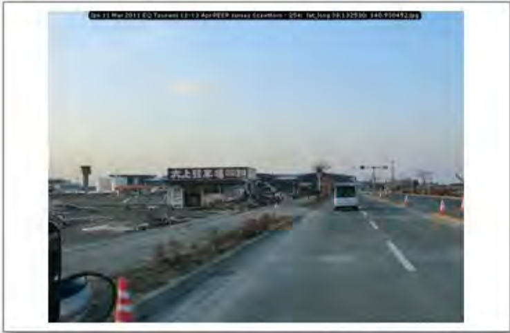
Jpn 11 Mar 2011 EQ Tsunami 11-13 Apr PEER survey Scawthorn - 254; lat_long 38.132530; 140.930452
