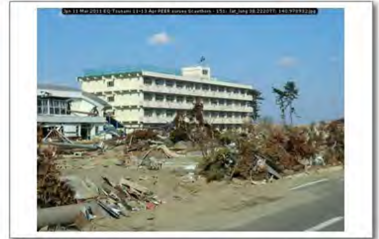
Jpn 11 Mar 2011 EQ Tsunami 11-13 Apr PEER survey Scawthorn - 151; lat_long 38.222077; 140.978932
