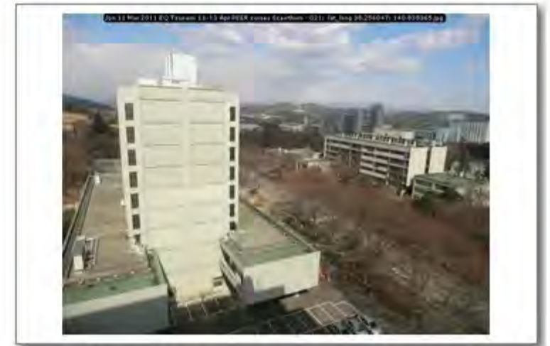
Jpn 11 Mar 2011 EQ Tsunami 11-13 Apr PEER survey Scawthorn - 021; lat_long 38.256047; 140.838365
