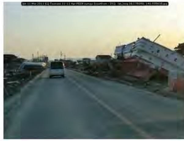
Jpn 11 Mar 2011 EQ Tsunami 11-13 Apr PEER survey Scawthorn - 252; lat_long 38.175090; 140.935635
