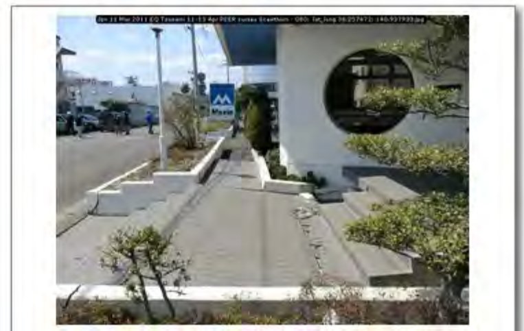
Jpn 11 Mar 2011 EQ Tsunami 11-13 Apr PEER survey Scawthorn - 080; lat_long 38.257472; 140.937933
