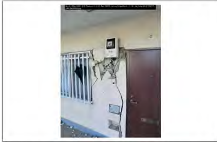
Jpn 11 Mar 2011 EQ Tsunami 11-13 Apr PEER survey Scawthorn - 112; lat_long 38.273437; 140.965088
