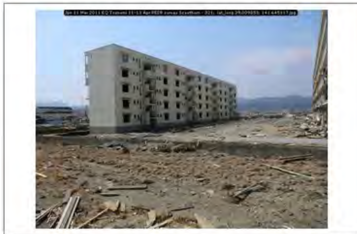
Jpn 11 Mar 2011 EQ Tsunami 11-13 Apr PEER survey Scawthorn - 321; lat_long 39.009853; 141.645117
