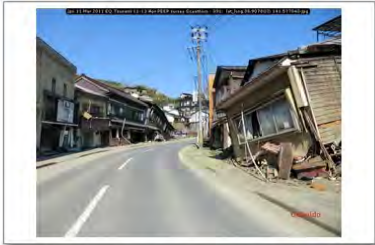
Jpn 11 Mar 2011 EQ Tsunami 11-13 Apr PEER survey Scawthorn - 391; lat_long 38.907807; 141.577040
