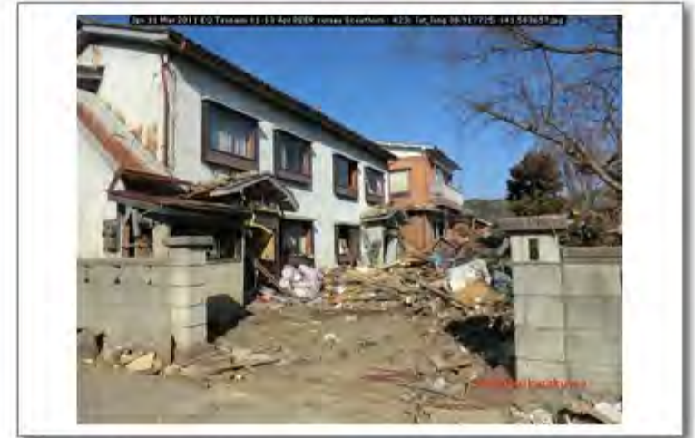
Jpn 11 Mar 2011 EQ Tsunami 11-13 Apr PEER survey Scawthorn - 423; lat_long 38.917725; 141.583657
