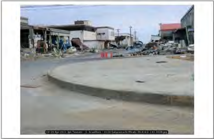
18-20 Apr 2011 Jpn Tsunami - C. Scawthorn - 0120 Sakanamachi Minato 38.4162; 141.3328
