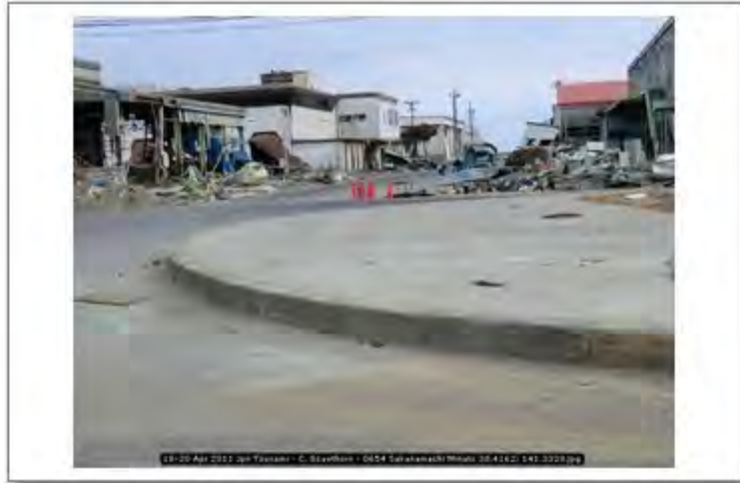
18-20 Apr 2011 Jpn Tsunami - C. Scawthorn - 0654 Sakanamachi Minato 38.4162; 141.3328
