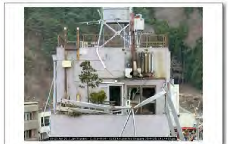
18-20 Apr 2011 Jpn Tsunami - C. Scawthorn - 0163 Koganechou Onagawa 38.4428; 141.4455
