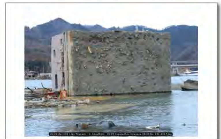
18-20 Apr 2011 Jpn Tsunami - C. Scawthorn - 0139 Koganechou Onagawa 38.4436; 141.4467
