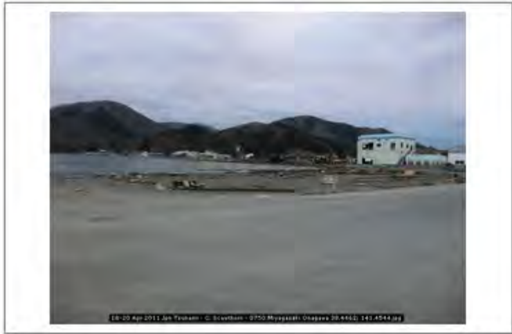
18-20 Apr 2011 Jpn Tsunami - C. Scawthorn - 0750 Miyagasaki Onagawa 38.4462; 141.4544
