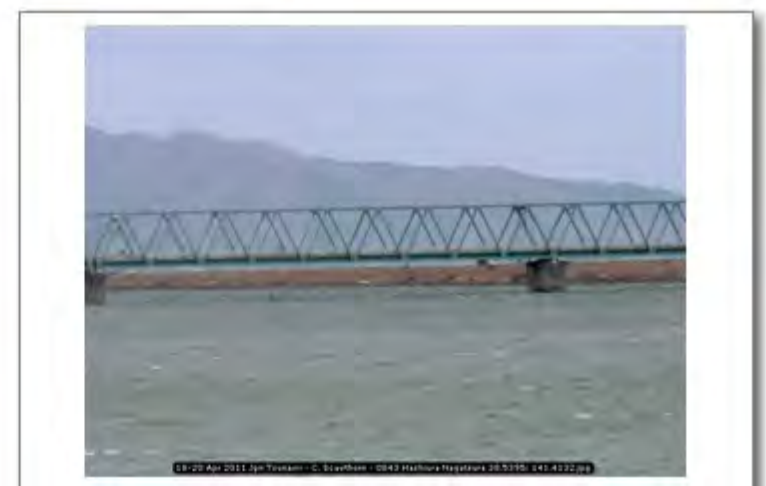
18-20 Apr 2011 Jpn Tsunami - C. Scawthorn - 0843 Hashiura Nagatsura 38.5395; 141.4132
