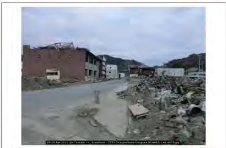
18-20 Apr 2011 Jpn Tsunami - C. Scawthorn - 0739 Onagawahama Onagawa 38.4465; 141.4473
