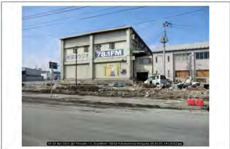
18-20 Apr 2011 Jpn Tsunami - C. Scawthorn - 0610 Nakanoshima Shiogama 38.3137; 141.0322
