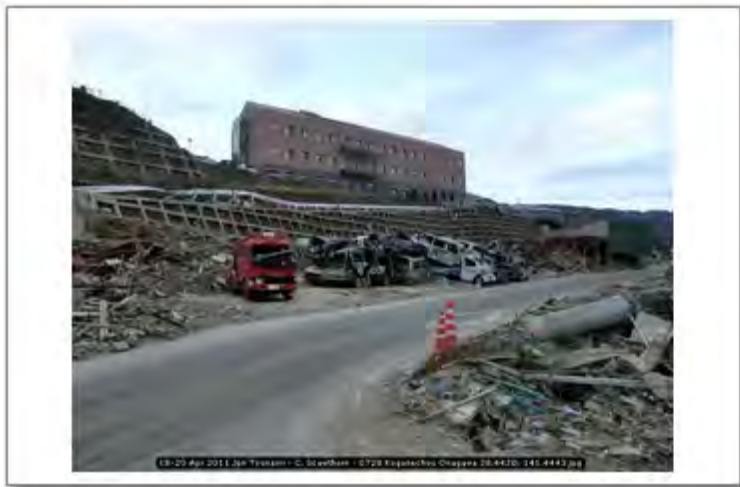
18-20 Apr 2011 Jpn Tsunami - C. Scawthorn - 0728 Koganechou Onagawa 38.4420; 141.4443
