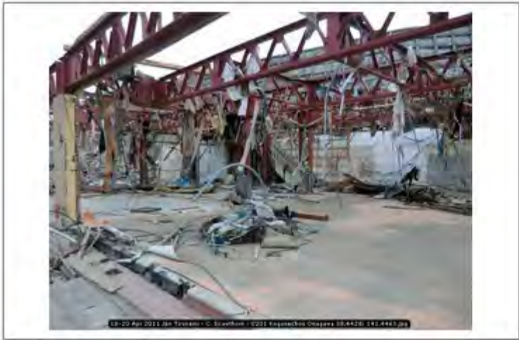
18-20 Apr 2011 Jpn Tsunami - C. Scawthorn - 0201 Koganechou Onagawa 38.4428; 141.4461
