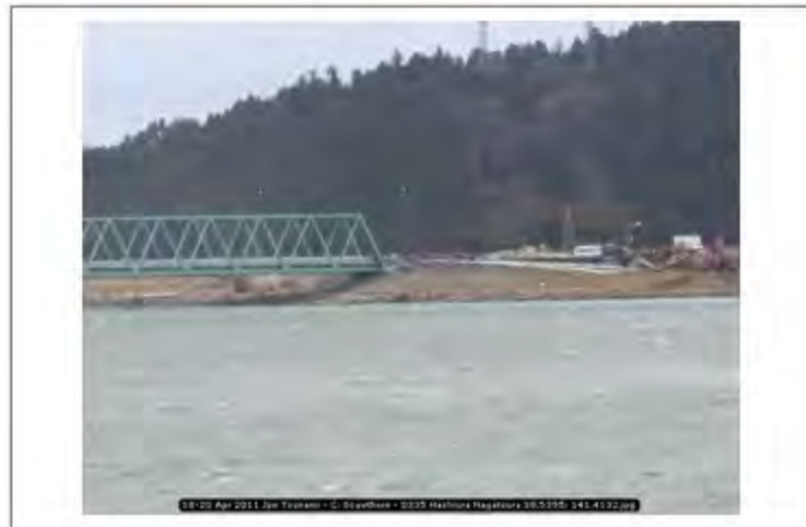
18-20 Apr 2011 Jpn Tsunami - C. Scawthorn - 0335 Hashiura Nagatsura 38.5395; 141.4132
