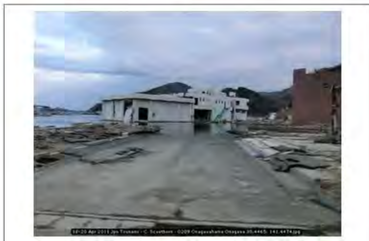
18-20 Apr 2011 Jpn Tsunami - C. Scawthorn - 0209 Onagawahama Onagawa 38.4465; 141.4474
