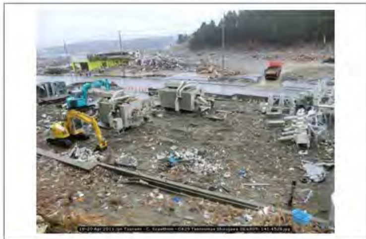
18-20 Apr 2011 Jpn Tsunami - C. Scawthorn - 0429 Tennoumae Shizugawa 38.6809; 141.4538
