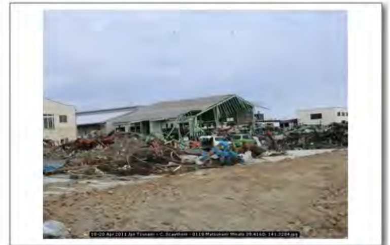
18-20 Apr 2011 Jpn Tsunami - C. Scawthorn - 0118 Matsunami Minato 38.4160; 141.3284
