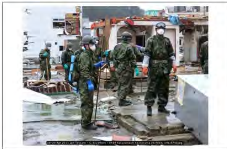
18-20 Apr 2011 Jpn Tsunami - C. Scawthorn - 0459 Sakanamachi Kesenuma 38.9066; 141.5755
