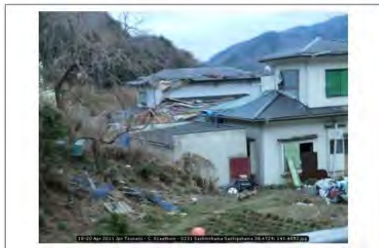
18-20 Apr 2011 Jpn Tsunami - C. Scawthorn - 0231 Sashinohama Sashigahama 38.4729; 141.4852
