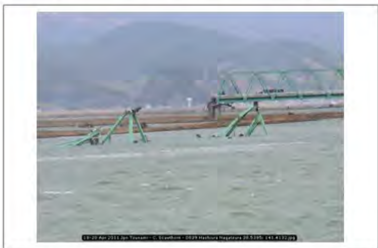
18-20 Apr 2011 Jpn Tsunami - C. Scawthorn - 0839 Hashiura Nagatsura 38.5395; 141.4132
