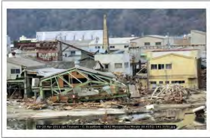
18-20 Apr 2011 Jpn Tsunami - C. Scawthorn - 0642 Myoujinchou Minato 38.4152; 141.3151
