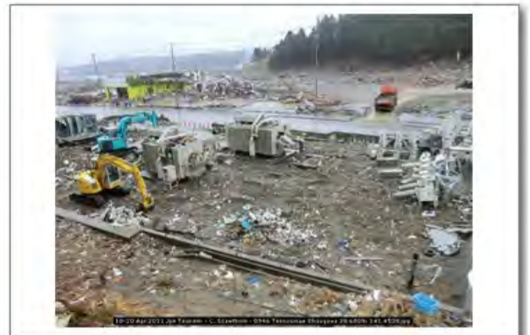
18-20 Apr 2011 Jpn Tsunami - C. Scawthorn - 0946 Tennoumae Shizugawa 38.6809; 141.4538
