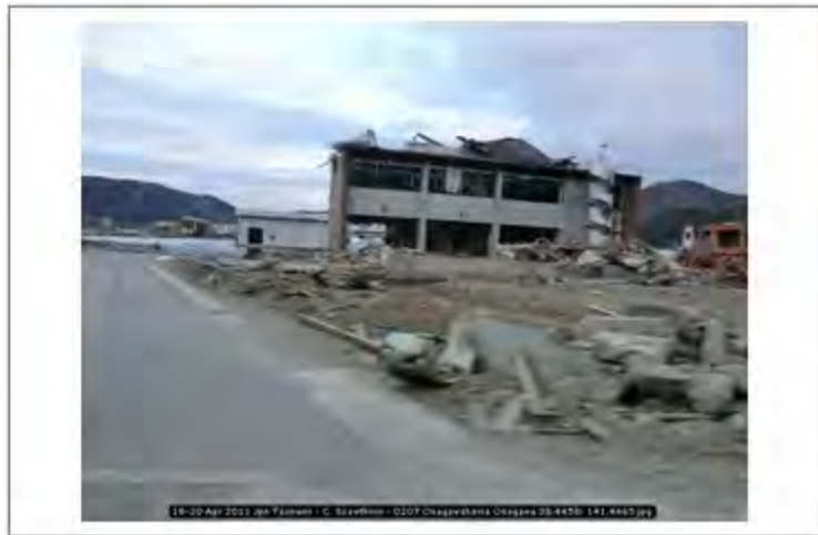
18-20 Apr 2011 Jpn Tsunami - C. Scawthorn - 0207 Onagawahama Onagawa 38.4458; 141.4465
