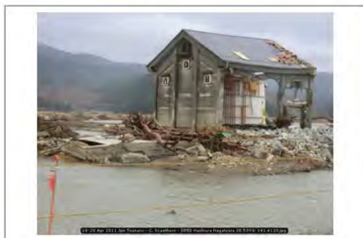
18-20 Apr 2011 Jpn Tsunami - C. Scawthorn - 0850 Hashiura Nagatsura 38.5393; 141.4133
