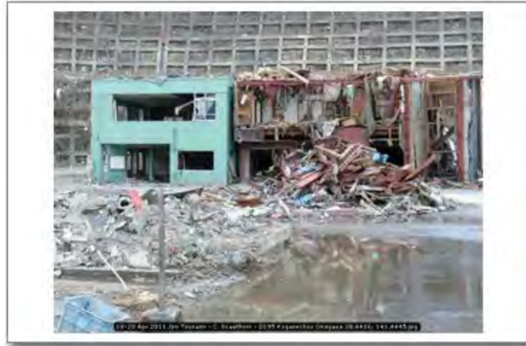
18-20 Apr 2011 Jpn Tsunami - C. Scawthorn - 0195 Koganechou Onagawa 38.4416; 141.4445
