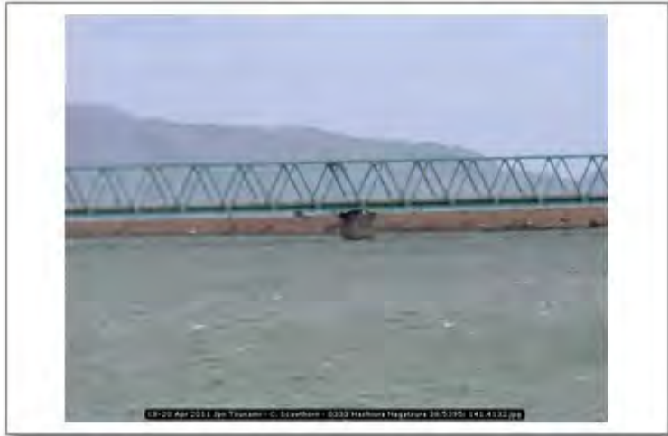
18-20 Apr 2011 Jpn Tsunami - C. Scawthorn - 0333 Hashiura Nagatsura 38.5395; 141.4132
