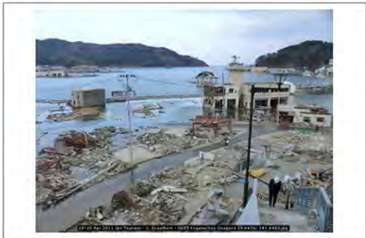
18-20 Apr 2011 Jpn Tsunami - C. Scawthorn - 0685 Koganechou Onagawa 38.4436; 141.4460
