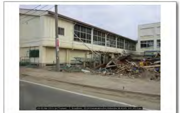
18-20 Apr 2011 Jpn Tsunami - C. Scawthorn - 0124 Hamamatsuchou Watanoha 38.4169; 141.3512
