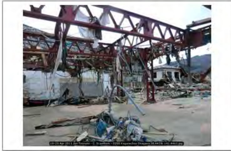
18-20 Apr 2011 Jpn Tsunami - C. Scawthorn - 0200 Koganechou Onagawa 38.4428; 141.4461
