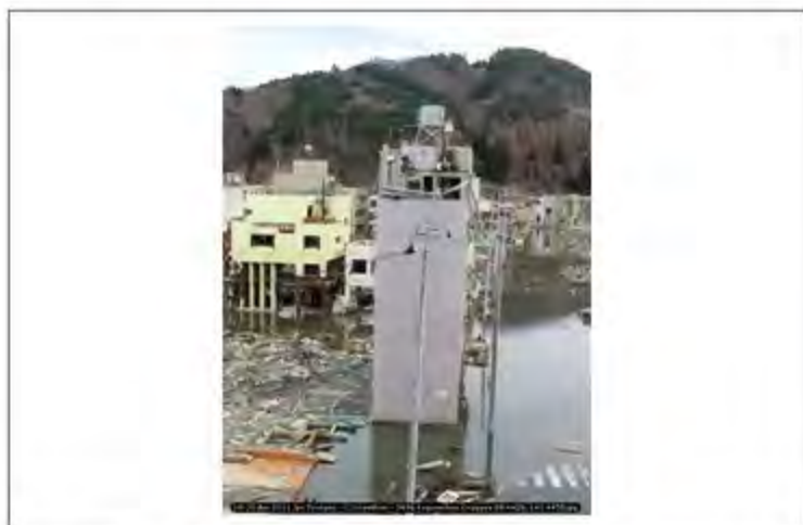
18-20 Apr 2011 Jpn Tsunami - C. Scawthorn - 0696 Koganechou Onagawa 38.4428; 141.4455
