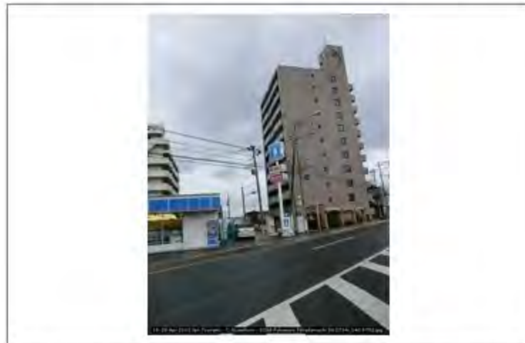
18-20 Apr 2011 Jpn Tsunami - C. Scawthorn - 0288 Fukumuro Fukudamachi 38.2734; 140.9702
