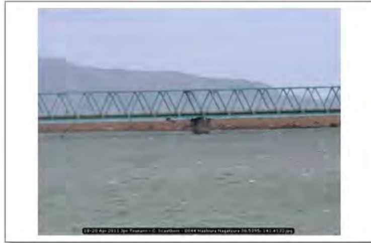
18-20 Apr 2011 Jpn Tsunami - C. Scawthorn - 0844 Hashiura Nagatsura 38.5395; 141.4132
