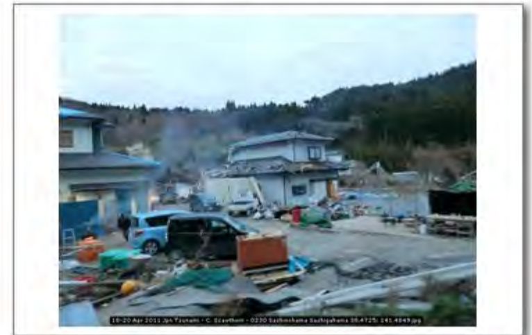
18-20 Apr 2011 Jpn Tsunami - C. Scawthorn - 0230 Sashinohama Sashigahama 38.4725; 141.4849
