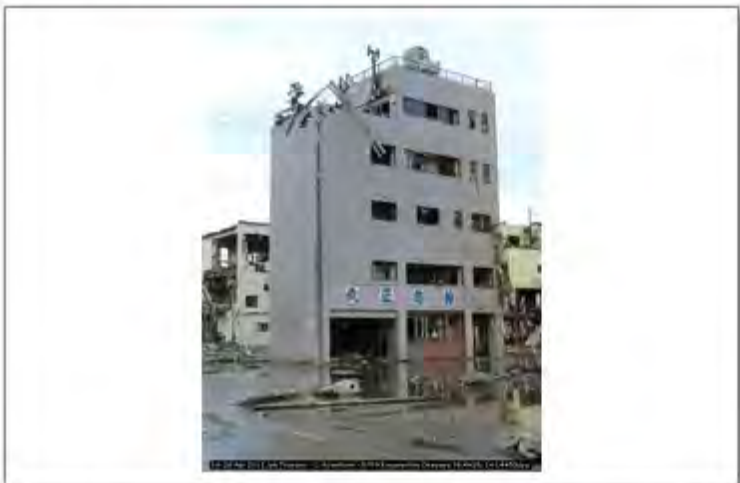
18-20 Apr 2011 Jpn Tsunami - C. Scawthorn - 0709 Koganechou Onagawa 38.4425; 141.4453
