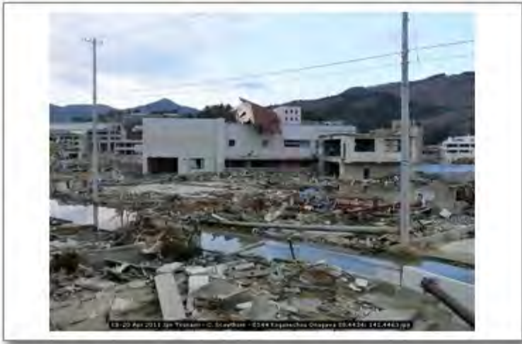
18-20 Apr 2011 Jpn Tsunami - C. Scawthorn - 0144 Koganechou Onagawa 38.4434; 141.4463
