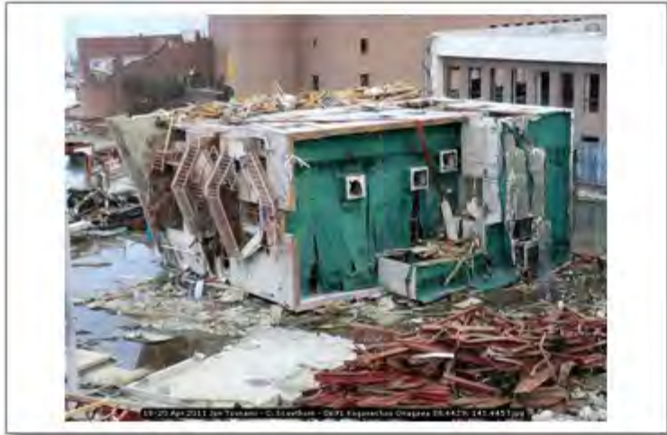
18-20 Apr 2011 Jpn Tsunami - C. Scawthorn - 0691 Koganechou Onagawa 38.4429; 141.4457
