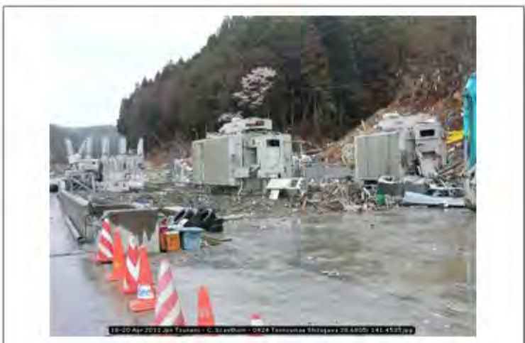
18-20 Apr 2011 Jpn Tsunami - C. Scawthorn - 0424 Tennoumae Shizugawa 38.6805; 141.4535
