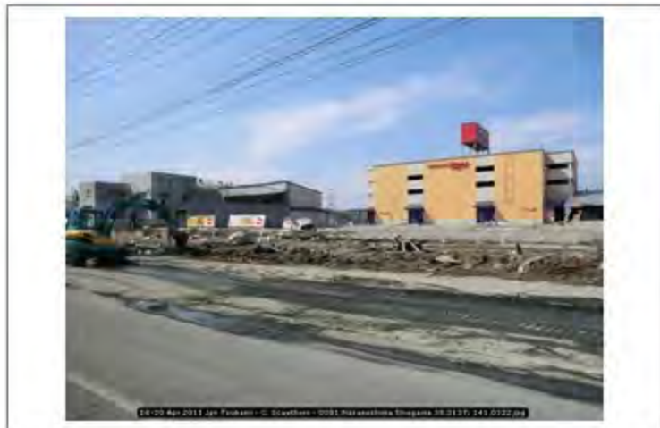
18-20 Apr 2011 Jpn Tsunami - C. Scawthorn - 0081 Nakanoshima Shiogama 38.3137; 141.0322
