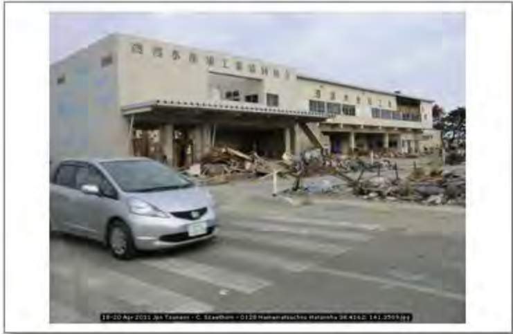
18-20 Apr 2011 Jpn Tsunami - C. Scawthorn - 0128 Hamamatsuchou Watanoha 38.4162; 141.3589
