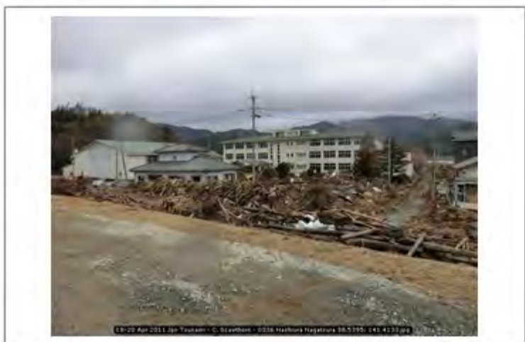
18-20 Apr 2011 Jpn Tsunami - C. Scawthorn - 0336 Hashiura Nagatsura 38.5395; 141.4133
