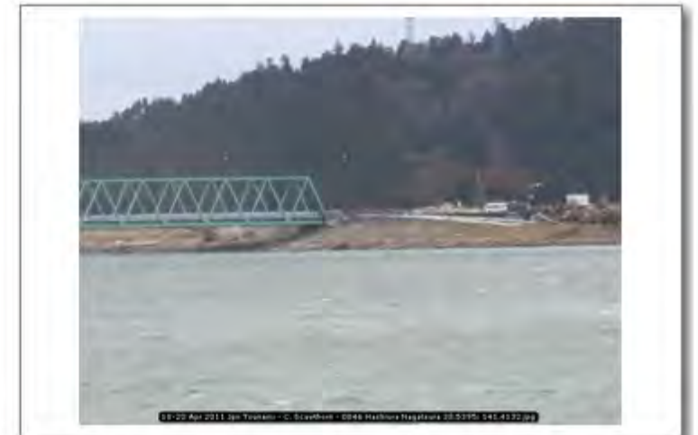
18-20 Apr 2011 Jpn Tsunami - C. Scawthorn - 0846 Hashiura Nagatsura 38.5395; 141.4132
