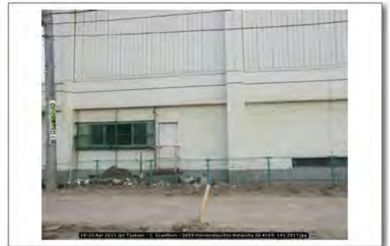
18-20 Apr 2011 Jpn Tsunami - C. Scawthorn - 0659 Hamamatsuchou Watanoha 38.4169; 141.3517
