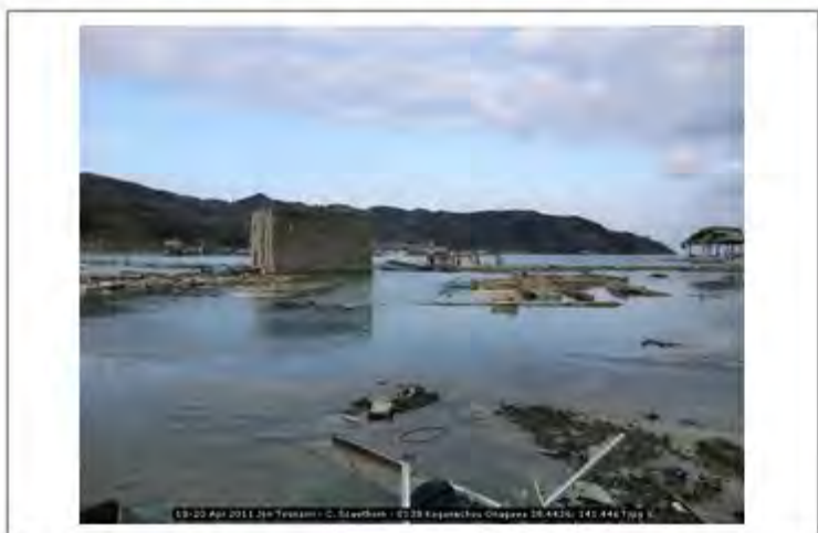
18-20 Apr 2011 Jpn Tsunami - C. Scawthorn - 0138 Koganechou Onagawa 38.4436; 141.4467
