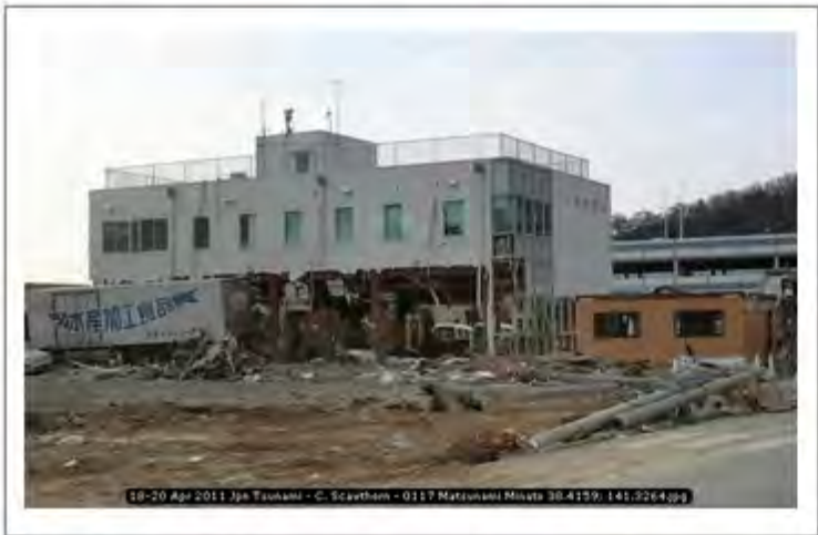
18-20 Apr 2011 Jpn Tsunami - C. Scawthorn - 0117 Matsunami Minato 38.4159; 141.3264
