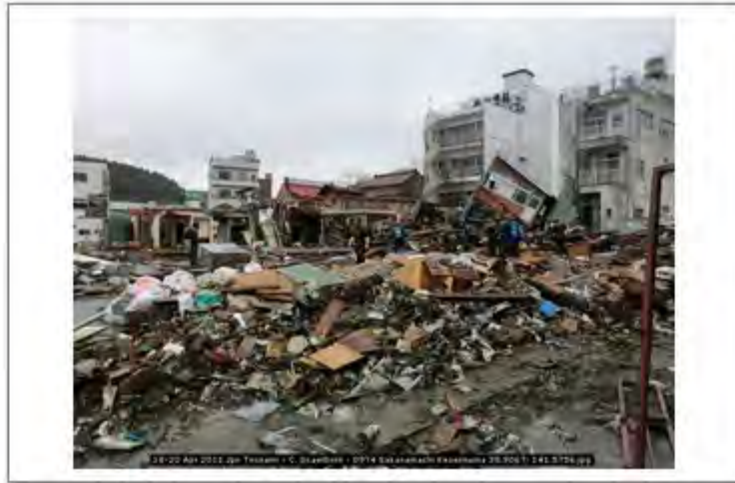
18-20 Apr 2011 Jpn Tsunami - C. Scawthorn - 0974 Sakanamachi Kesenuma 38.9067; 141.5756
