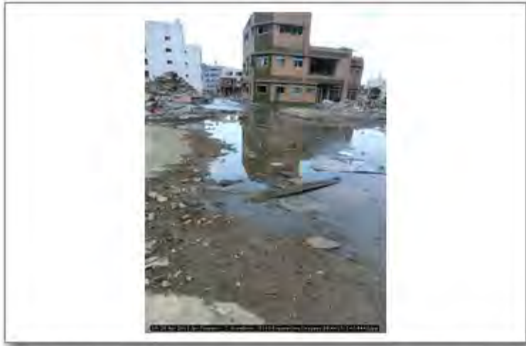
18-20 Apr 2011 Jpn Tsunami - C. Scawthorn - 0193 Koganechou Onagawa 38.4417; 141.4442
