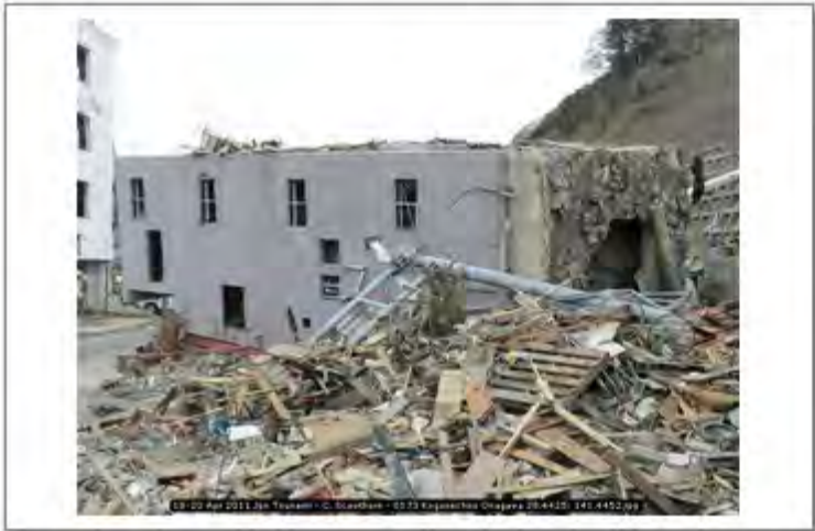
18-20 Apr 2011 Jpn Tsunami - C. Scawthorn - 0173 Koganechou Onagawa 38.4425; 141.4452
