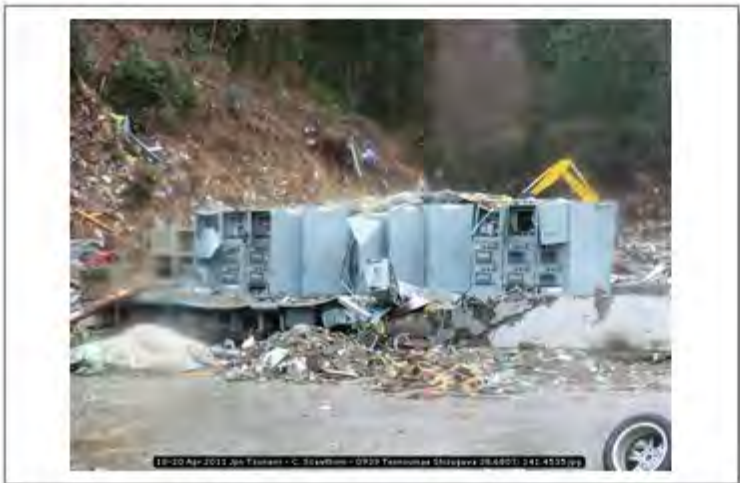
18-20 Apr 2011 Jpn Tsunami - C. Scawthorn - 0939 Tennoumae Shizugawa 38.6807; 141.4535
