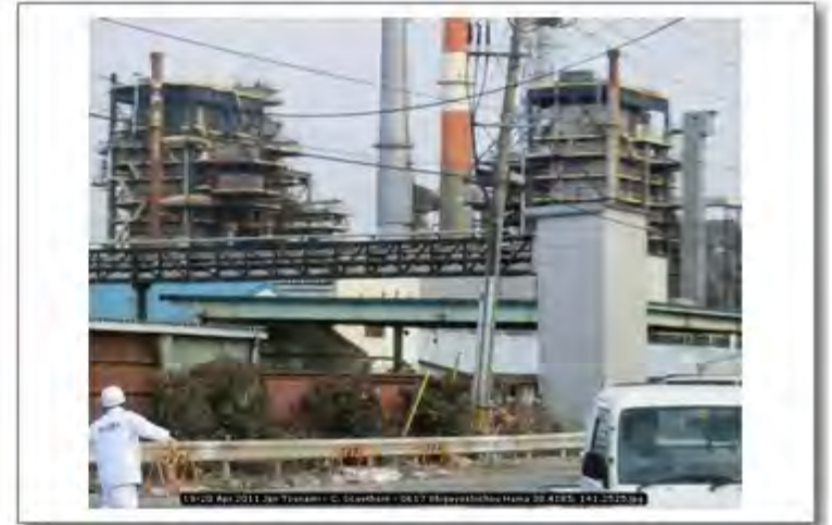
18-20 Apr 2011 Jpn Tsunami - C. Scawthorn - 0617 Shigeyoshichou Hama 38.4185; 141.2525
