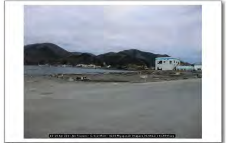
18-20 Apr 2011 Jpn Tsunami - C. Scawthorn - 0218 Miyagasaki Onagawa 38.4462; 141.4544
