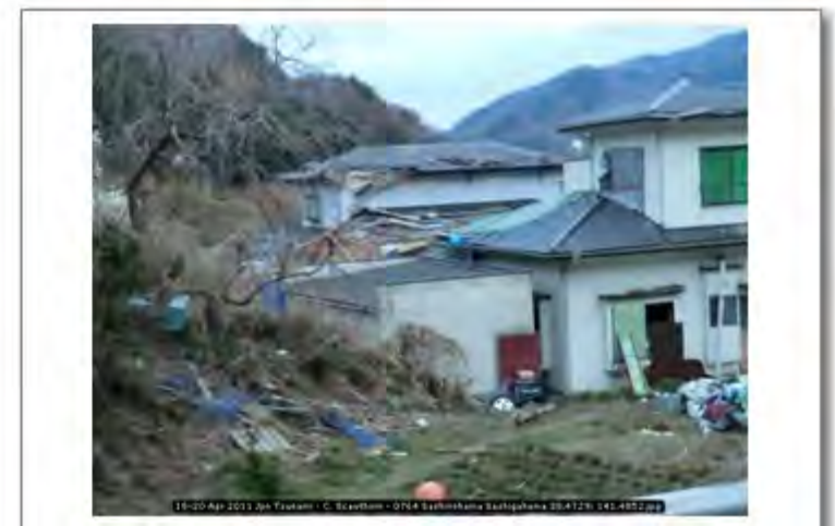
18-20 Apr 2011 Jpn Tsunami - C. Scawthorn - 0764 Sashinohama Sashigahama 38.4729; 141.4852
