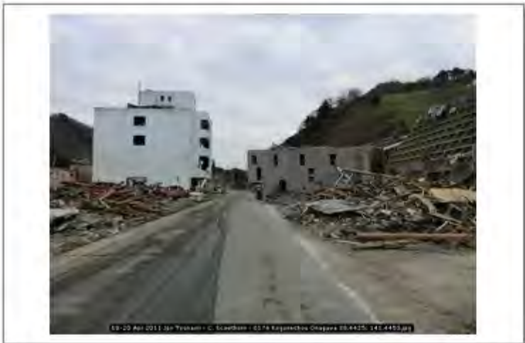
18-20 Apr 2011 Jpn Tsunami - C. Scawthorn - 0176 Koganechou Onagawa 38.4425; 141.4453
