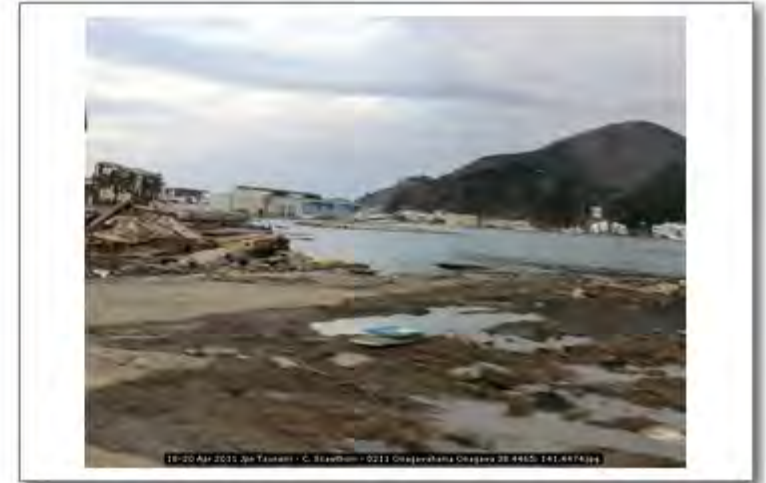
18-20 Apr 2011 Jpn Tsunami - C. Scawthorn - 0211 Onagawahama Onagawa 38.4465; 141.4474
