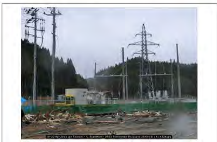
18-20 Apr 2011 Jpn Tsunami - C. Scawthorn - 0933 Tennoumae Shizugawa 38.6815; 141.4526
