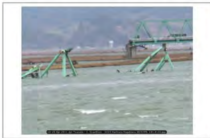
18-20 Apr 2011 Jpn Tsunami - C. Scawthorn - 0323 Hashiura Nagatsura 38.5395; 141.4132
