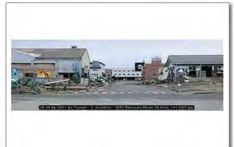
18-20 Apr 2011 Jpn Tsunami - C. Scawthorn - 0653 Matsunami Minato 38.4161; 141.3307
