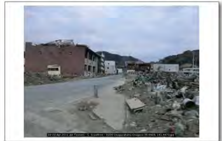
18-20 Apr 2011 Jpn Tsunami - C. Scawthorn - 0208 Onagawahama Onagawa 38.4465; 141.4473
