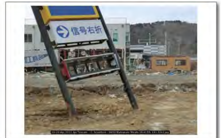
18-20 Apr 2011 Jpn Tsunami - C. Scawthorn - 0650 Matsunami Minato 38.4159; 141.3262
