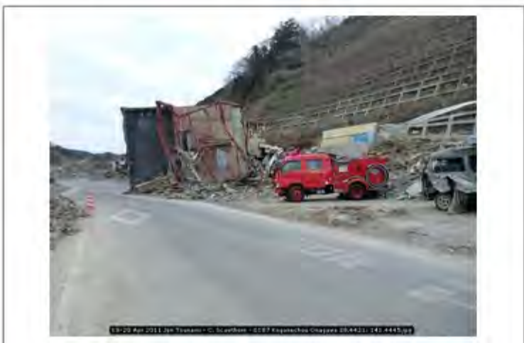
18-20 Apr 2011 Jpn Tsunami - C. Scawthorn - 0187 Koganechou Onagawa 38.4421; 141.4445
