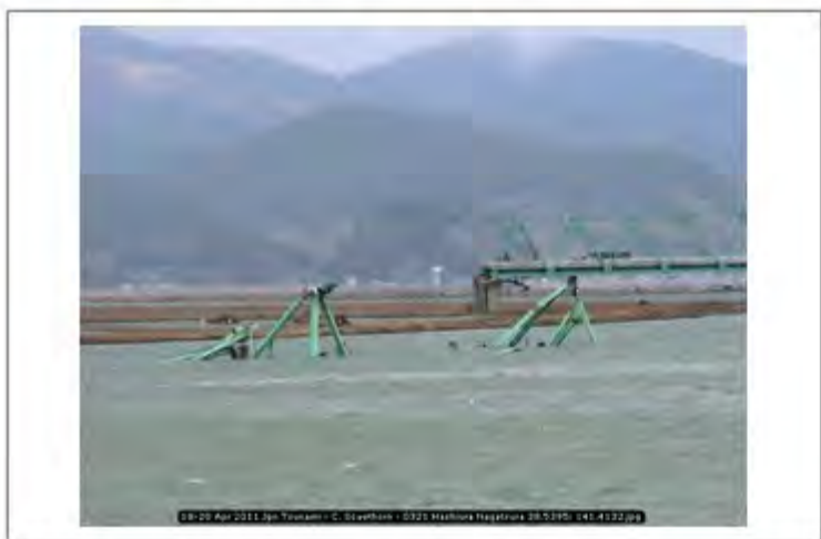
18-20 Apr 2011 Jpn Tsunami - C. Scawthorn - 0321 Hashiura Nagatsura 38.5395; 141.4132
