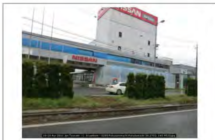
18-20 Apr 2011 Jpn Tsunami - C. Scawthorn - 0285 Fukuzumimachi Fukudamachi 38.2702; 140.9520
