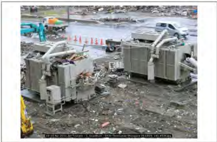
18-20 Apr 2011 Jpn Tsunami - C. Scawthorn - 0430 Tennoumae Shizugawa 38.6809; 141.4538
