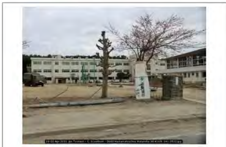
18-20 Apr 2011 Jpn Tsunami - C. Scawthorn - 0660 Hamamatsuchou Watanoha 38.4169; 141.3522
