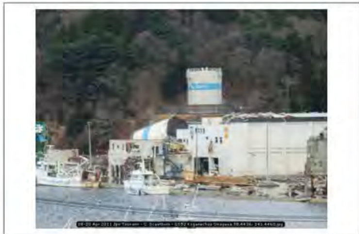
18-20 Apr 2011 Jpn Tsunami - C. Scawthorn - 0152 Koganechou Onagawa 38.4436; 141.4460
