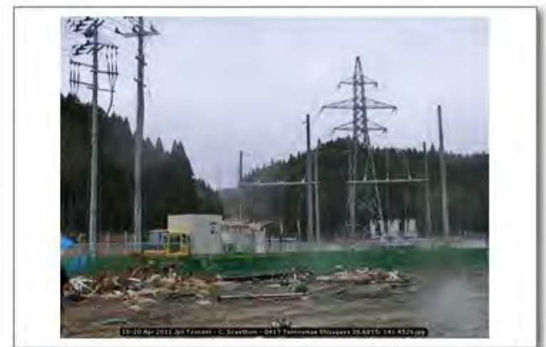
18-20 Apr 2011 Jpn Tsunami - C. Scawthorn - 0417 Tennoumae Shizugawa 38.6815; 141.4526
