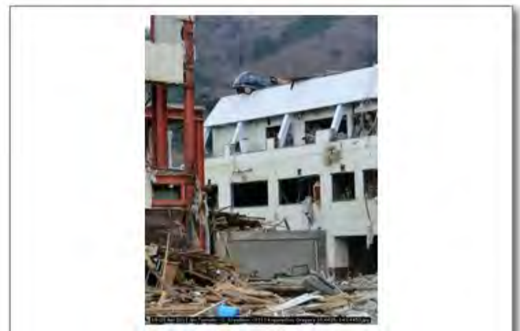
18-20 Apr 2011 Jpn Tsunami - C. Scawthorn - 0713 Koganechou Onagawa 38.4425; 141.4453
