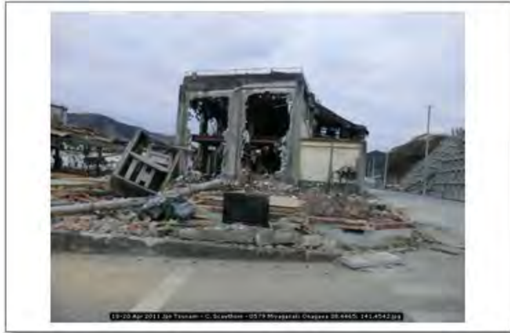
18-20 Apr 2011 Jpn Tsunami - C. Scawthorn - 0579 Miyagasaki Onagawa 38.4465; 141.4542
