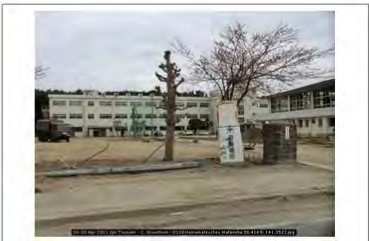
18-20 Apr 2011 Jpn Tsunami - C. Scawthorn - 0126 Hamamatsuchou Watanoha 38.4169; 141.3522
