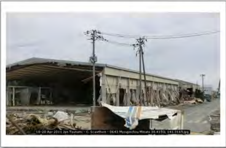
18-20 Apr 2011 Jpn Tsunami - C. Scawthorn - 0643 Myoujinchou Minato 38.4153; 141.3165
