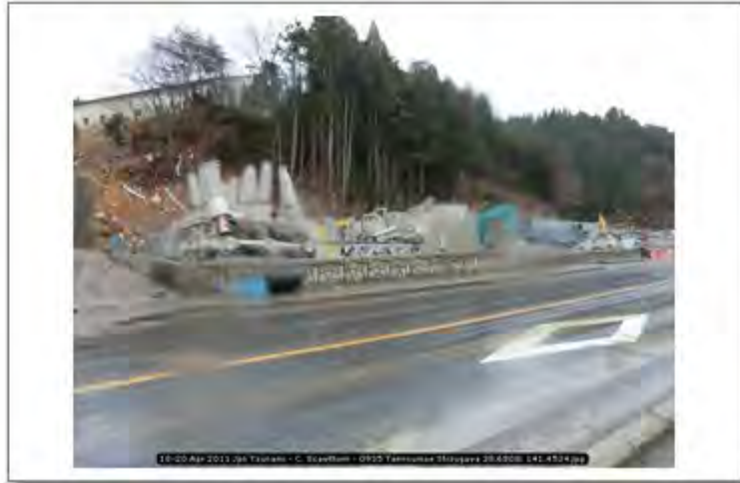
18-20 Apr 2011 Jpn Tsunami - C. Scawthorn - 0935 Tennoumae Shizugawa 38.6808; 141.4534
