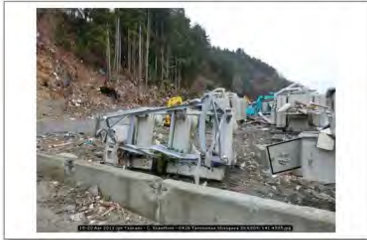
18-20 Apr 2011 Jpn Tsunami - C. Scawthorn - 0426 Tennoumae Shizugawa 38.6809; 141.4535
