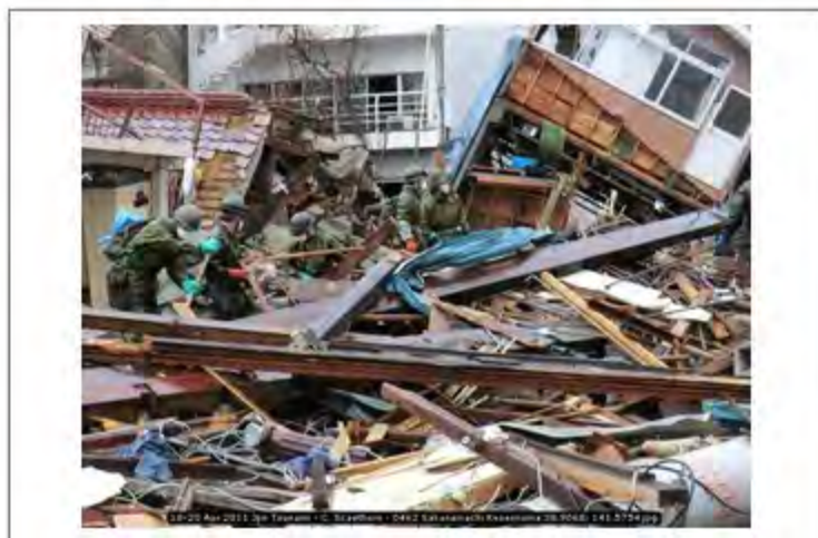
18-20 Apr 2011 Jpn Tsunami - C. Scawthorn - 0462 Sakanamachi Kesenuma 38.9068; 141.5754
