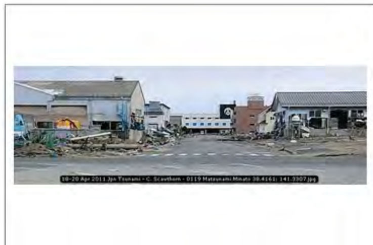
18-20 Apr 2011 Jpn Tsunami - C. Scawthorn - 0119 Matsunami Minato 38.4161; 141.3307
