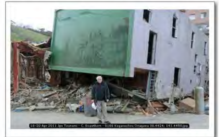
18-20 Apr 2011 Jpn Tsunami - C. Scawthorn - 0186 Koganechou Onagawa 38.4424; 141.4450
