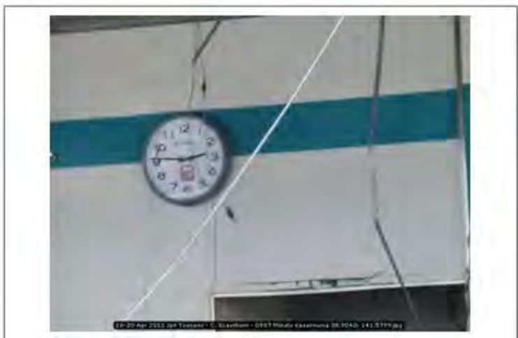
18-20 Apr 2011 Jpn Tsunami - C. Scawthorn - 0987 Minato Kesennuma 38.9040; 141.5799
