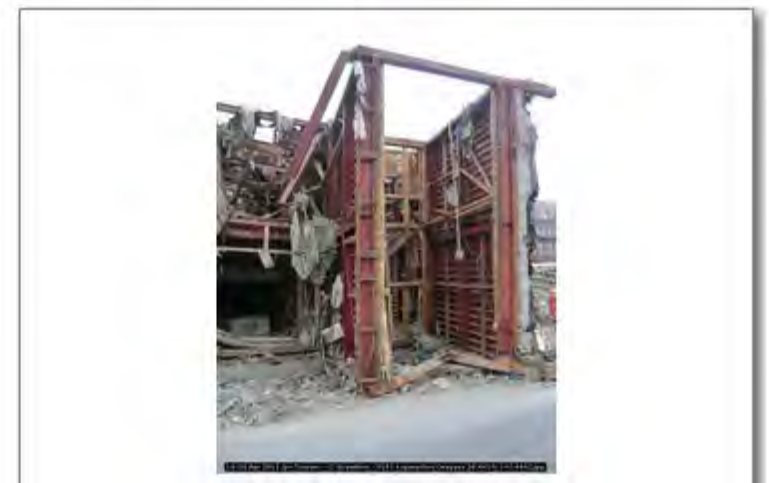
18-20 Apr 2011 Jpn Tsunami - C. Scawthorn - 0191 Koganechou Onagawa 38.4419; 141.4442
