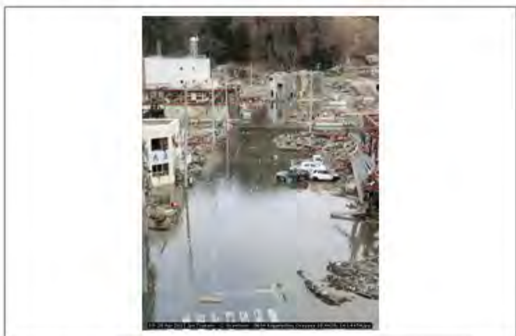
18-20 Apr 2011 Jpn Tsunami - C. Scawthorn - 0694 Koganechou Onagawa 38.4428; 141.4454
