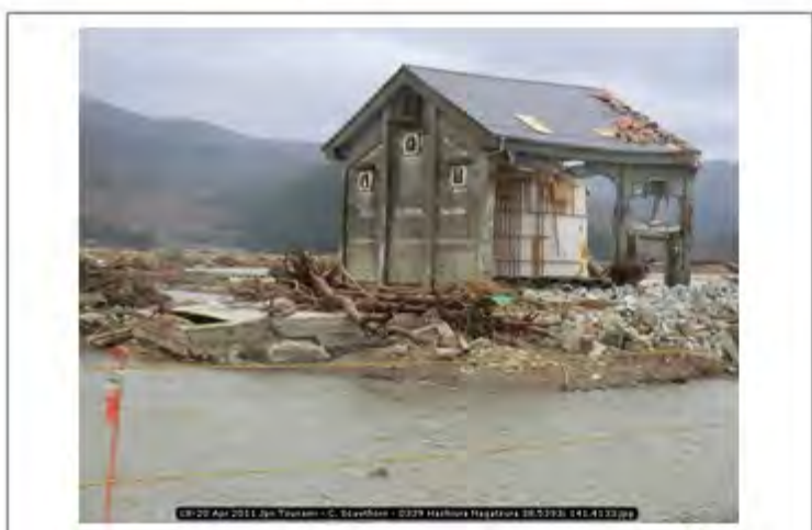
18-20 Apr 2011 Jpn Tsunami - C. Scawthorn - 0339 Hashiura Nagatsura 38.5393; 141.4133
