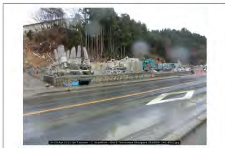
18-20 Apr 2011 Jpn Tsunami - C. Scawthorn - 0418 Tennoumae Shizugawa 38.6809; 141.4532
