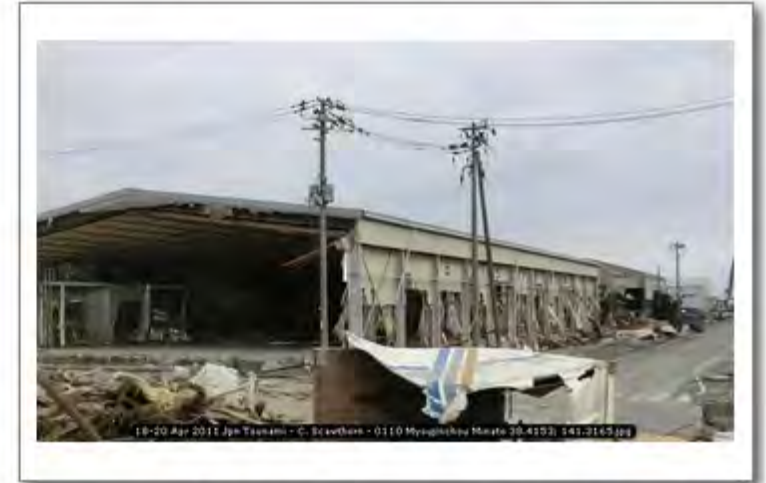
18-20 Apr 2011 Jpn Tsunami - C. Scawthorn - 0110 Myoujinchou Minato 38.4153; 141.3165
