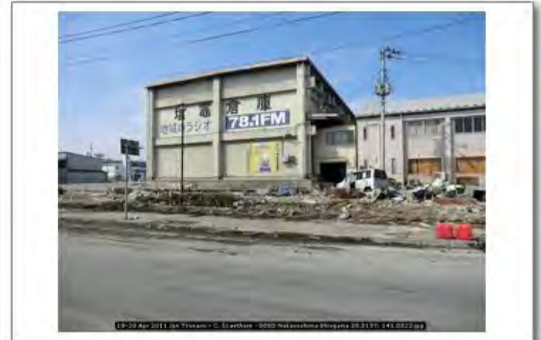
18-20 Apr 2011 Jpn Tsunami - C. Scawthorn - 0080 Nakanoshima Shiogama 38.3137; 141.0322
