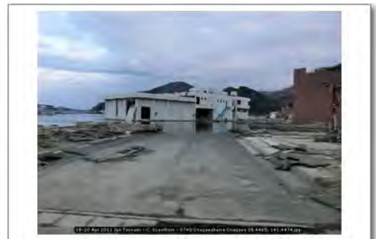
18-20 Apr 2011 Jpn Tsunami - C. Scawthorn - 0740 Onagawahama Onagawa 38.4465; 141.4474
