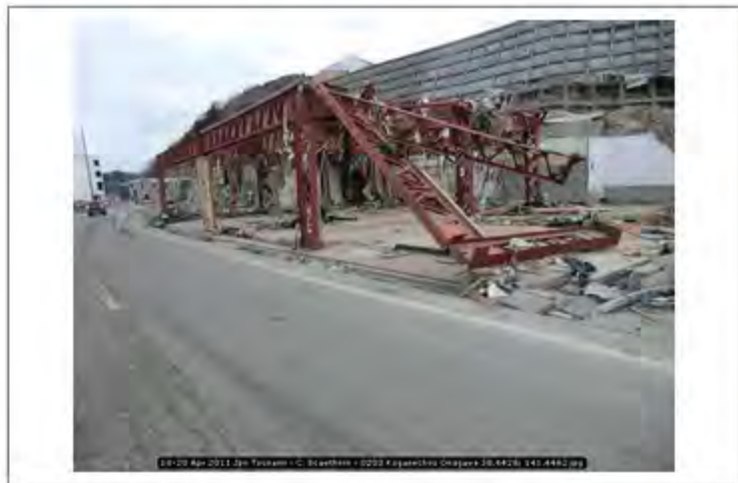
18-20 Apr 2011 Jpn Tsunami - C. Scawthorn - 0203 Koganechou Onagawa 38.4428; 141.4462
