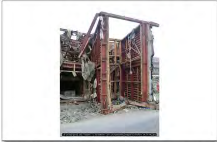
18-20 Apr 2011 Jpn Tsunami - C. Scawthorn - 0722 Koganechou Onagawa 38.4419; 141.4442
