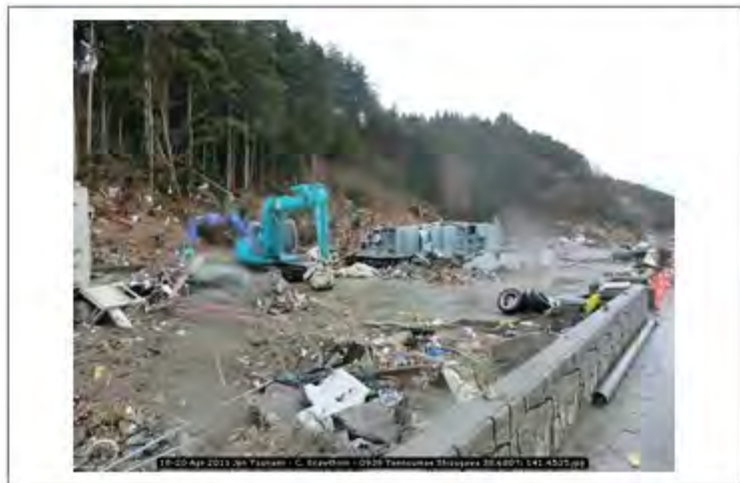
18-20 Apr 2011 Jpn Tsunami - C. Scawthorn - 0938 Tennoumae Shizugawa 38.6807; 141.4535
