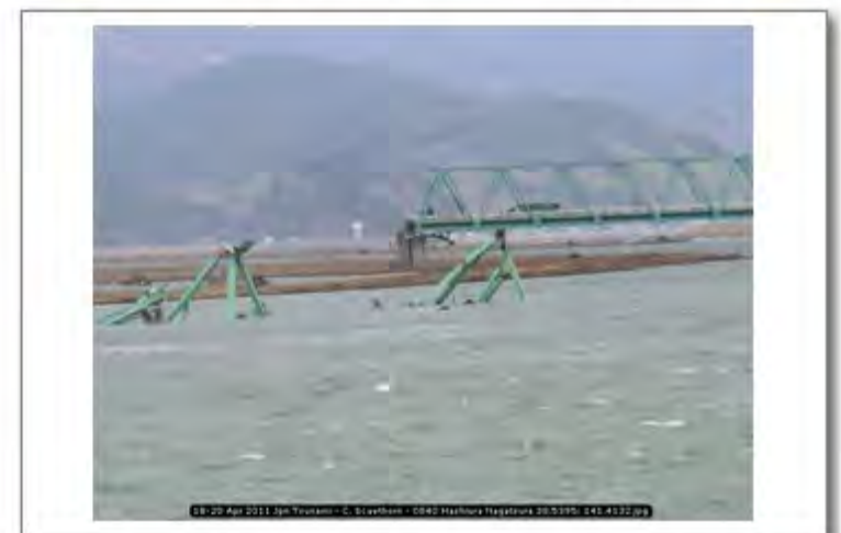
18-20 Apr 2011 Jpn Tsunami - C. Scawthorn - 0840 Hashiura Nagatsura 38.5395; 141.4132
