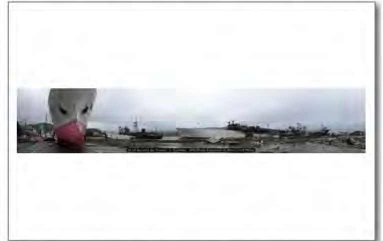
18-20 Apr 2011 Jpn Tsunami - C. Scawthorn - 0982 Minato Kesennuma 38.9042; 141.5798
