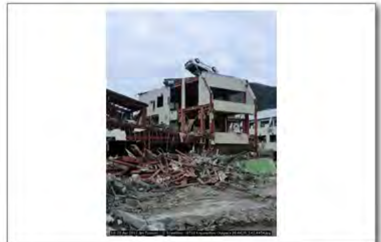
18-20 Apr 2011 Jpn Tsunami - C. Scawthorn - 0710 Koganechou Onagawa 38.4425; 141.4454
