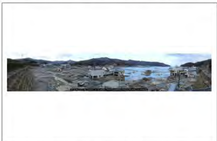
18-20 Apr 2011 Jpn Tsunami - C. Scawthorn - 0153 Koganechou Onagawa 38.4436; 141.4460
