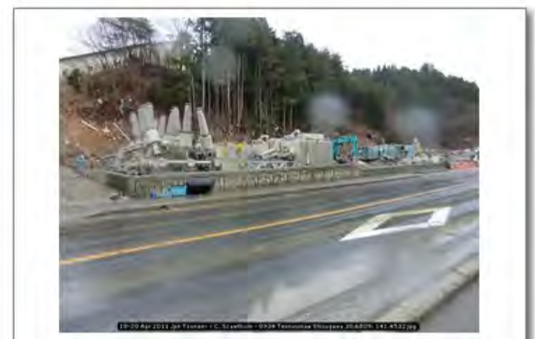
18-20 Apr 2011 Jpn Tsunami - C. Scawthorn - 0934 Tennoumae Shizugawa 38.6809; 141.4532
