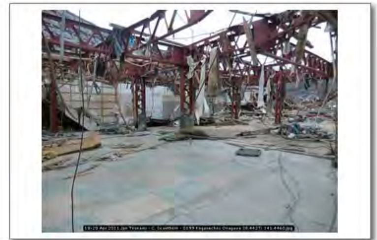
18-20 Apr 2011 Jpn Tsunami - C. Scawthorn - 0199 Koganechou Onagawa 38.4427; 141.4460
