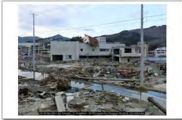
18-20 Apr 2011 Jpn Tsunami - C. Scawthorn - 0678 Koganechou Onagawa 38.4434; 141.4463
