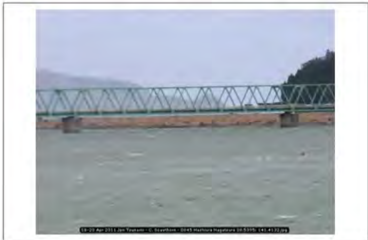
18-20 Apr 2011 Jpn Tsunami - C. Scawthorn - 0845 Hashiura Nagatsura 38.5395; 141.4132
