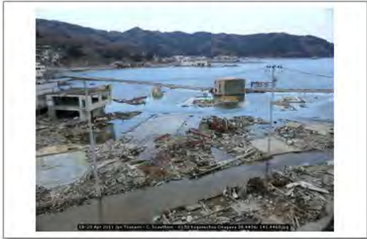
18-20 Apr 2011 Jpn Tsunami - C. Scawthorn - 0150 Koganechou Onagawa 38.4436; 141.4460
