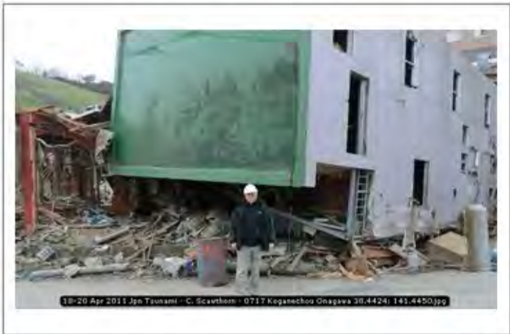
18-20 Apr 2011 Jpn Tsunami - C. Scawthorn - 0717 Koganechou Onagawa 38.4424; 141.4450
