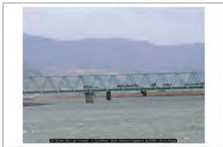
18-20 Apr 2011 Jpn Tsunami - C. Scawthorn - 0841 Hashiura Nagatsura 38.5395; 141.4132
