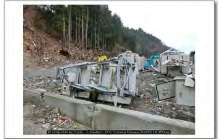
18-20 Apr 2011 Jpn Tsunami - C. Scawthorn - 0943 Tennoumae Shizugawa 38.6809; 141.4535
