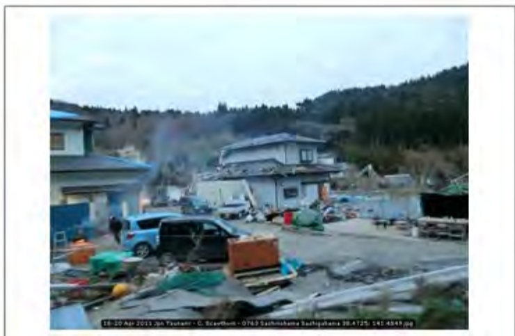
18-20 Apr 2011 Jpn Tsunami - C. Scawthorn - 0763 Sashinohama Sashigahama 38.4725; 141.4849
