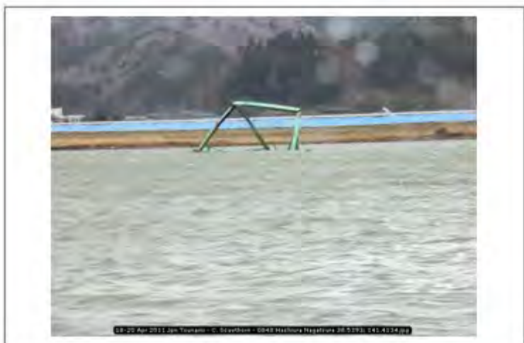
18-20 Apr 2011 Jpn Tsunami - C. Scawthorn - 0848 Hashiura Nagatsura 38.5393; 141.4134
