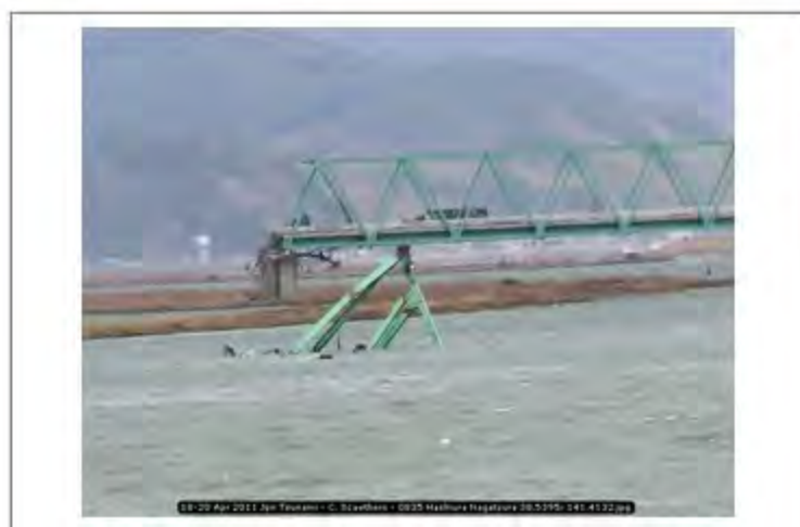
18-20 Apr 2011 Jpn Tsunami - C. Scawthorn - 0835 Hashiura Nagatsura 38.5395; 141.4132
