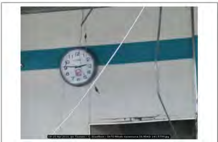
18-20 Apr 2011 Jpn Tsunami - C. Scawthorn - 0470 Minato Kesennuma 38.9040; 141.5799
