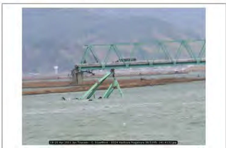
18-20 Apr 2011 Jpn Tsunami - C. Scawthorn - 0324 Hashiura Nagatsura 38.5395; 141.4132
