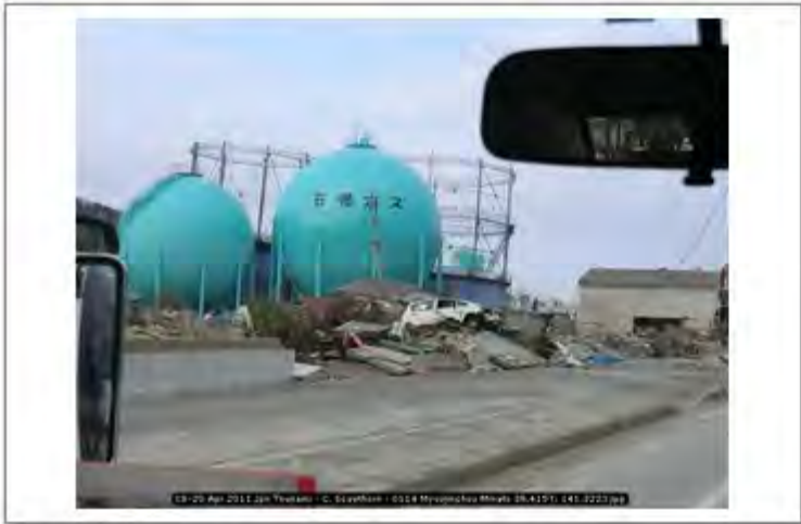
18-20 Apr 2011 Jpn Tsunami - C. Scawthorn - 0114 Myoujinchou Minato 38.4157; 141.3223
