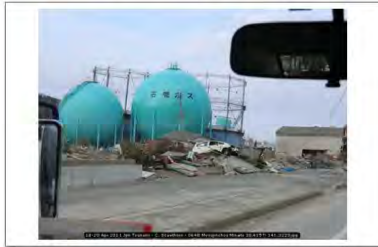
18-20 Apr 2011 Jpn Tsunami - C. Scawthorn - 0648 Myoujinchou Minato 38.4157; 141.3223
