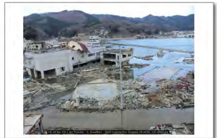
18-20 Apr 2011 Jpn Tsunami - C. Scawthorn - 0683 Koganechou Onagawa 38.4436; 141.4460
