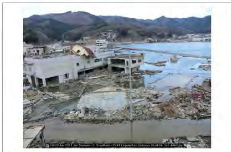
18-20 Apr 2011 Jpn Tsunami - C. Scawthorn - 0149 Koganechou Onagawa 38.4436; 141.4460
