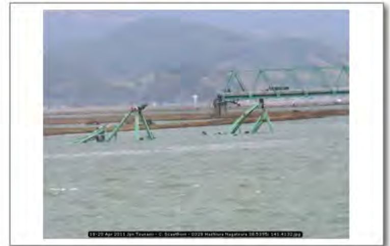
18-20 Apr 2011 Jpn Tsunami - C. Scawthorn - 0328 Hashiura Nagatsura 38.5395; 141.4132
