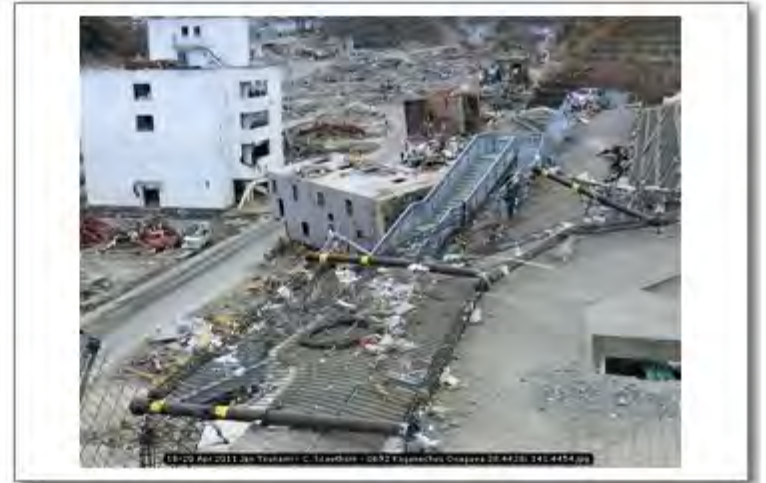
18-20 Apr 2011 Jpn Tsunami - C. Scawthorn - 0692 Koganechou Onagawa 38.4428; 141.4454
