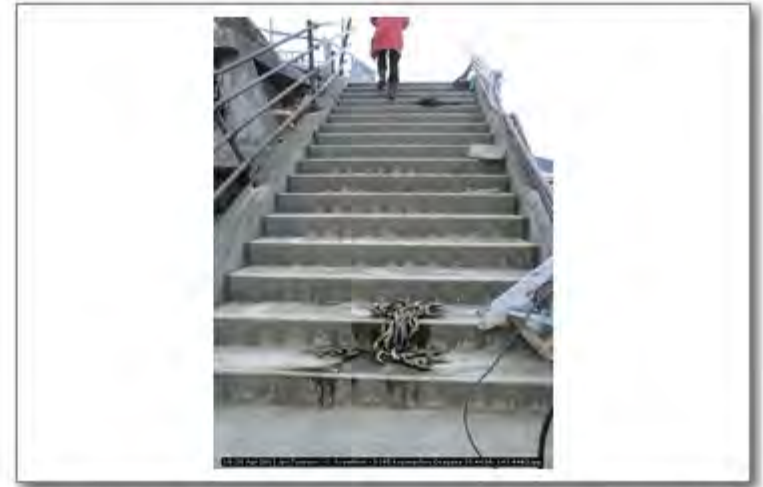
18-20 Apr 2011 Jpn Tsunami - C. Scawthorn - 0145 Koganechou Onagawa 38.4434; 141.4463
