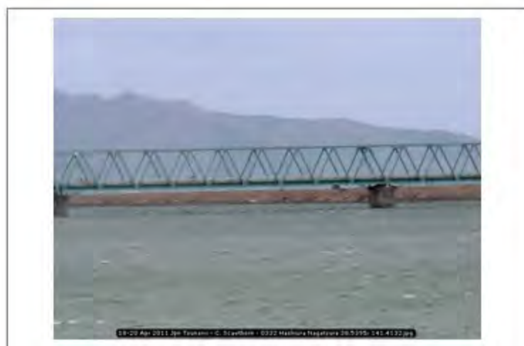
18-20 Apr 2011 Jpn Tsunami - C. Scawthorn - 0332 Hashiura Nagatsura 38.5395; 141.4132
