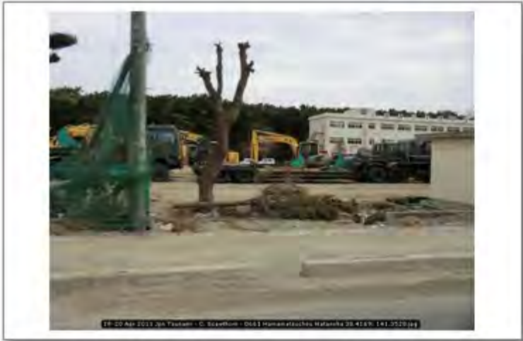
18-20 Apr 2011 Jpn Tsunami - C. Scawthorn - 0661 Hamamatsuchou Watanoha 38.4169; 141.3528
