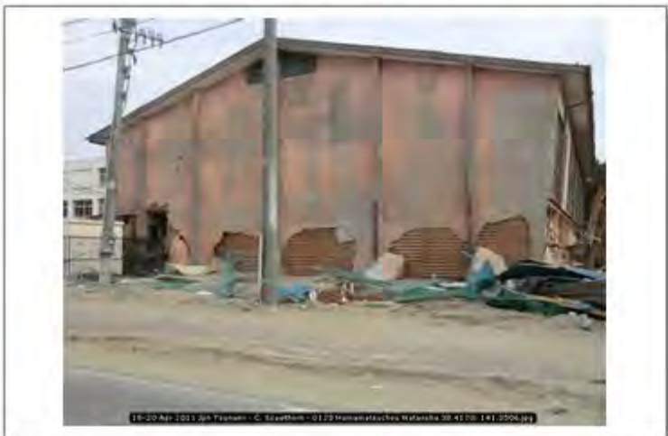
18-20 Apr 2011 Jpn Tsunami - C. Scawthorn - 0123 Hamamatsuchou Watanoha 38.4170; 141.3506
