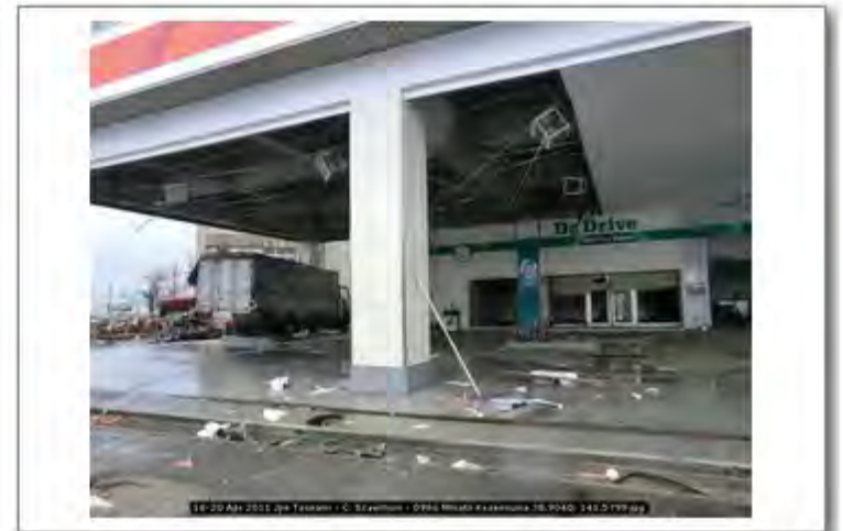
18-20 Apr 2011 Jpn Tsunami - C. Scawthorn - 0986 Minato Kesennuma 38.9040; 141.5799
