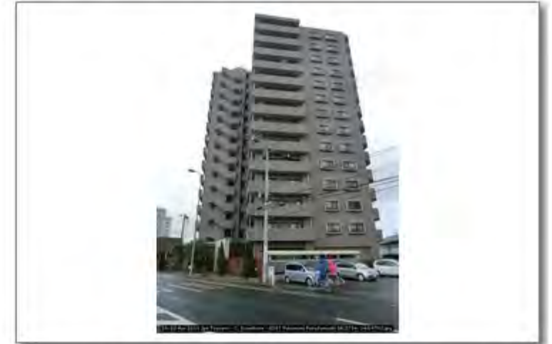
18-20 Apr 2011 Jpn Tsunami - C. Scawthorn - 0287 Fukumuro Fukudamachi 38.2734; 140.9702
