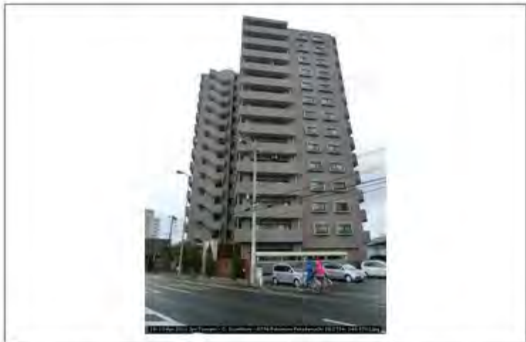
18-20 Apr 2011 Jpn Tsunami - C. Scawthorn - 0796 Fukumuro Fukudamachi 38.2734; 140.9702
