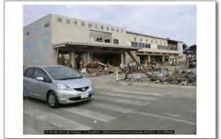
18-20 Apr 2011 Jpn Tsunami - C. Scawthorn - 0662 Hamamatsuchou Watanoha 38.4162; 141.3589
