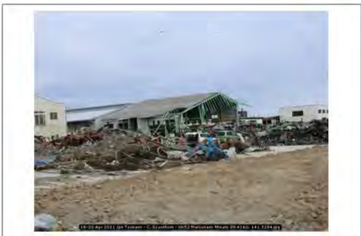
18-20 Apr 2011 Jpn Tsunami - C. Scawthorn - 0652 Matsunami Minato 38.4160; 141.3284
