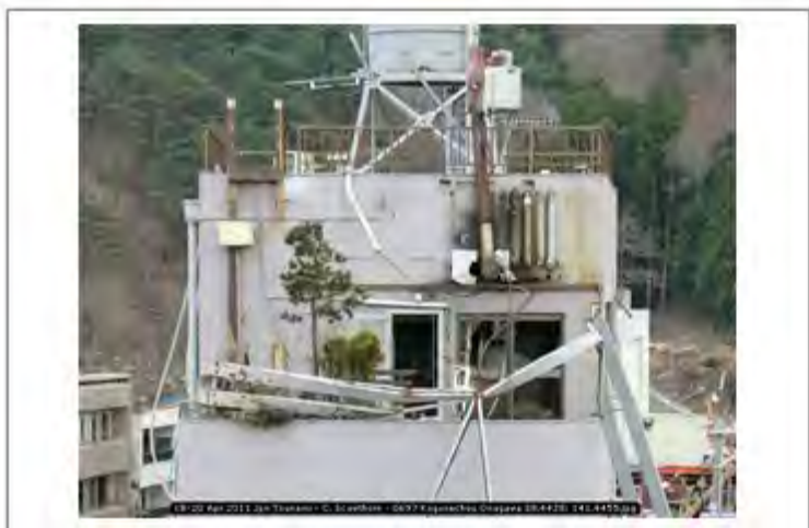
18-20 Apr 2011 Jpn Tsunami - C. Scawthorn - 0697 Koganechou Onagawa 38.4428; 141.4455
