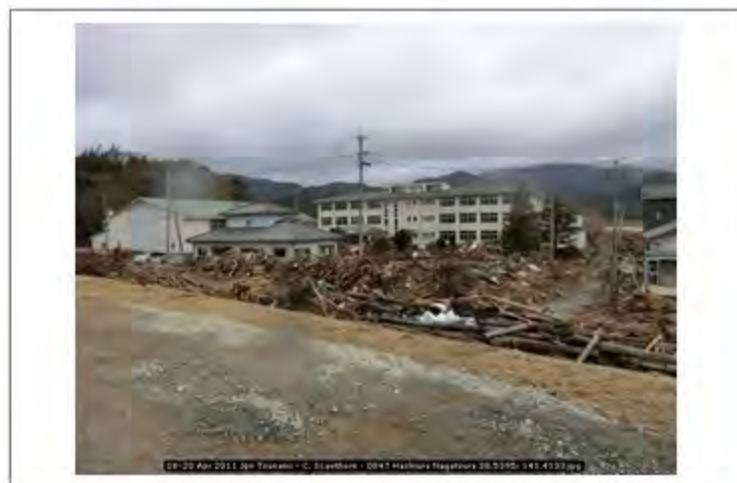
18-20 Apr 2011 Jpn Tsunami - C. Scawthorn - 0847 Hashiura Nagatsura 38.5395; 141.4133
