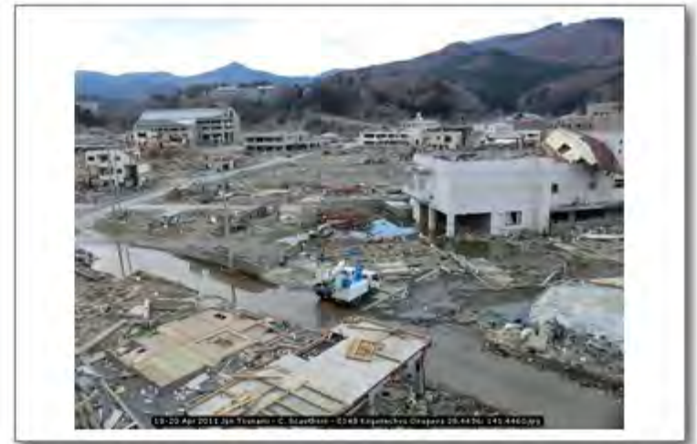
18-20 Apr 2011 Jpn Tsunami - C. Scawthorn - 0148 Koganechou Onagawa 38.4436; 141.4460
