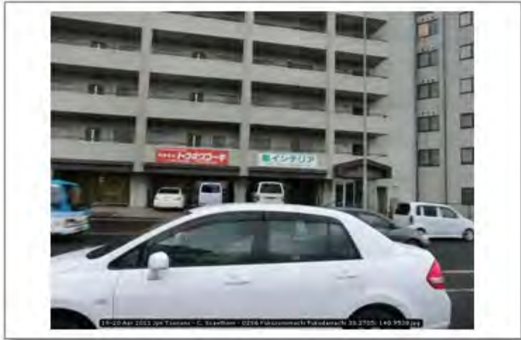
18-20 Apr 2011 Jpn Tsunami - C. Scawthorn - 0286 Fukuzumimachi Fukudamachi 38.2705; 140.9538
