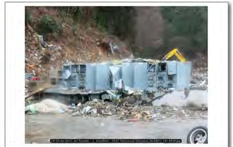
18-20 Apr 2011 Jpn Tsunami - C. Scawthorn - 0422 Tennoumae Shizugawa 38.6807; 141.4535
