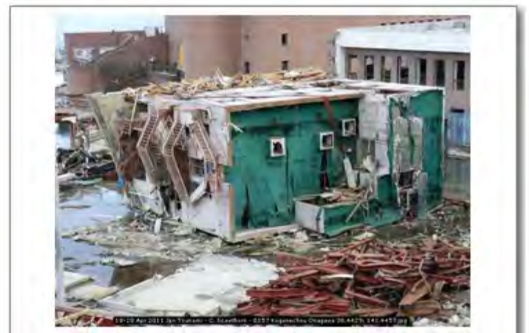
18-20 Apr 2011 Jpn Tsunami - C. Scawthorn - 0157 Koganechou Onagawa 38.4429; 141.4457
