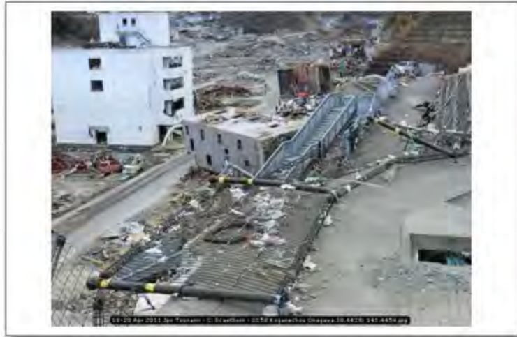
18-20 Apr 2011 Jpn Tsunami - C. Scawthorn - 0158 Koganechou Onagawa 38.4428; 141.4454
