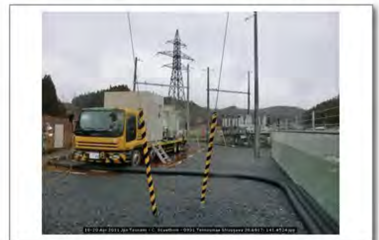
18-20 Apr 2011 Jpn Tsunami - C. Scawthorn - 0931 Tennoumae Shizugawa 38.6817; 141.4524
