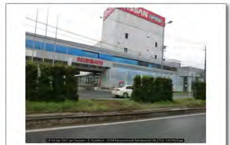
18-20 Apr 2011 Jpn Tsunami - C. Scawthorn - 0794 Fukuzumimachi Fukudamachi 38.2702; 140.9520
