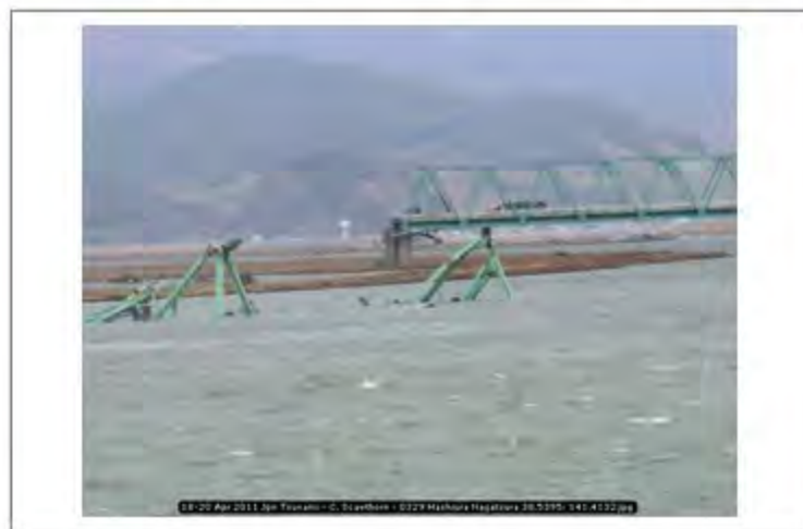
18-20 Apr 2011 Jpn Tsunami - C. Scawthorn - 0329 Hashiura Nagatsura 38.5395; 141.4132
