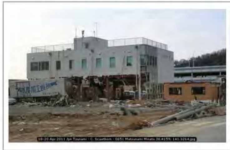
18-20 Apr 2011 Jpn Tsunami - C. Scawthorn - 0651 Matsunami Minato 38.4159; 141.3264
