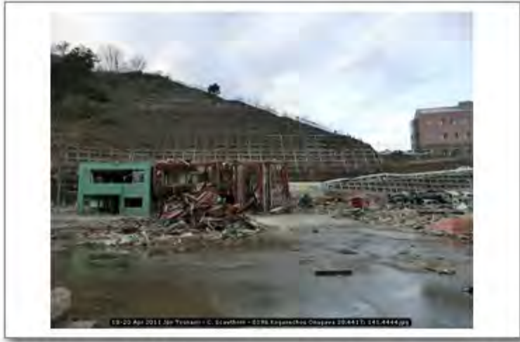
18-20 Apr 2011 Jpn Tsunami - C. Scawthorn - 0196 Koganechou Onagawa 38.4417; 141.4444
