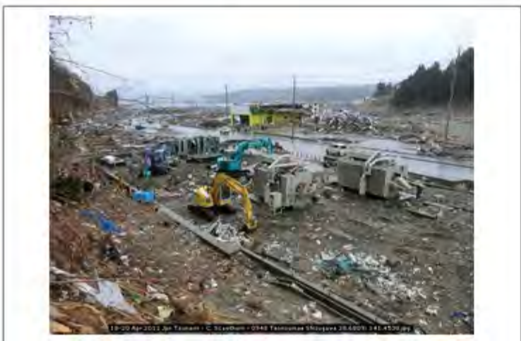
18-20 Apr 2011 Jpn Tsunami - C. Scawthorn - 0948 Tennoumae Shizugawa 38.6809; 141.4538
