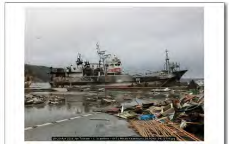
18-20 Apr 2011 Jpn Tsunami - C. Scawthorn - 0471 Minato Kesennuma 38.9040; 141.5799
