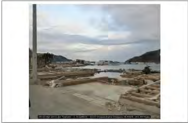
18-20 Apr 2011 Jpn Tsunami - C. Scawthorn - 0210 Onagawahama Onagawa 38.4465; 141.4474
