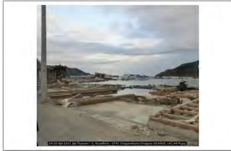
18-20 Apr 2011 Jpn Tsunami - C. Scawthorn - 0741 Onagawahama Onagawa 38.4465; 141.4474
