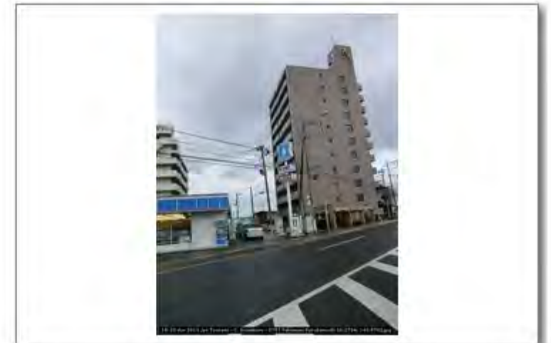
18-20 Apr 2011 Jpn Tsunami - C. Scawthorn - 0797 Fukumuro Fukudamachi 38.2734; 140.9702
