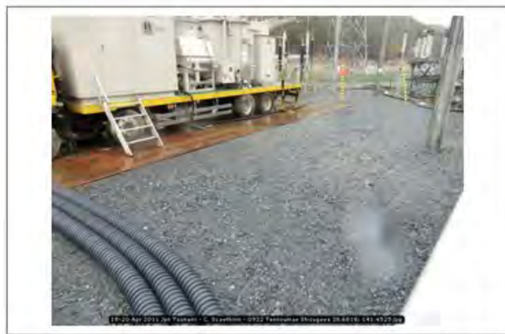
18-20 Apr 2011 Jpn Tsunami - C. Scawthorn - 0932 Tennoumae Shizugawa 38.6818; 141.4525
